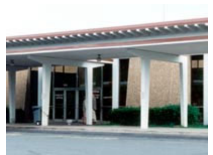
Figure 6-21: Existing Charlotte Station
