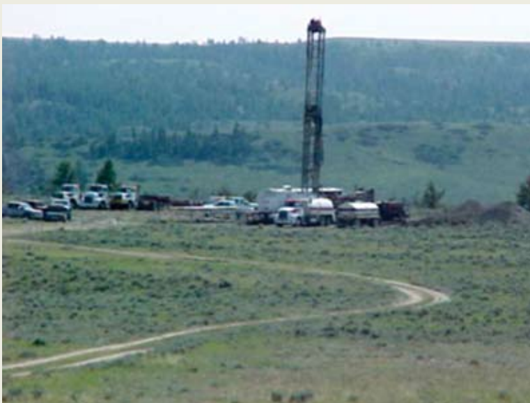
A minimum disturbance, primitive, two-track road winds its way to a drilling operation. To further reduce disturbance, most of the well location has not been stripped of vegetation or topsoil.
