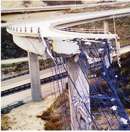
TRANSPORTATION SYSTEM CATASTROPHES: Collapsed highway in Los Angeles caused by the Northridge earthquake. (Photo courtesy of the National Information Service for Earthquake Engineering, Univ. of California, Berkeley) CENTER: New York City subway on the morning of September 11, after the attack. (Photo ©AP/World Wide Photo) RIGHT: One of the primary transportation actions taken in Washington on September 11 was closing I-395 inside the Beltway to facilitate movement of emergency vehicles. (Photo courtesy of the Federal Emergency Management Administration)
