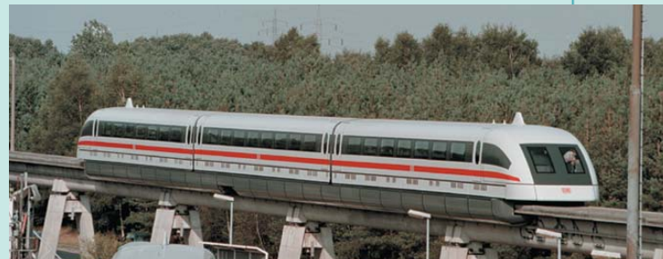
The Transrapid 08 prototype maglev train in Hamburg, Germany, installed on an improved guideway.
