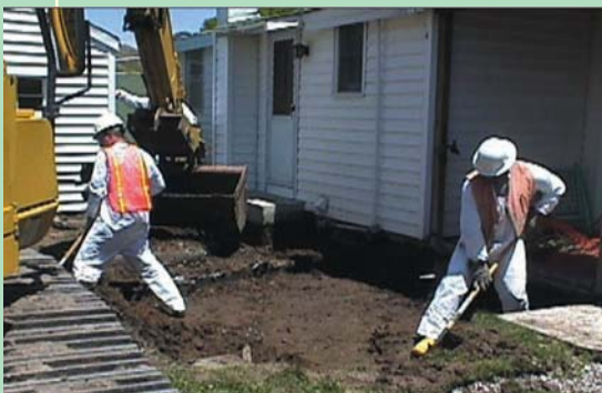
Soil contaminated with lead and arsenic from old ore smelters being cleaned up in Stockton, Utah.
