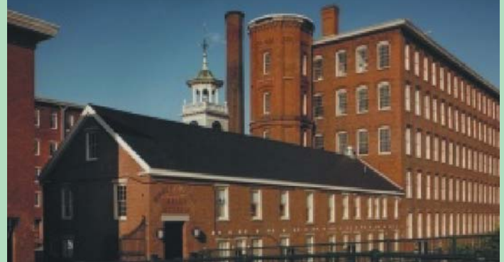
An EPA brownfields site in Lowell, Massachusetts, where contaminants are being cleaned up to ready the site for redevelopment.
