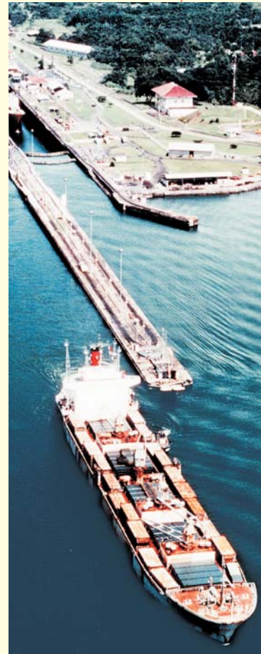
Aerial view of Gatun Locks in the Panama Canal.
