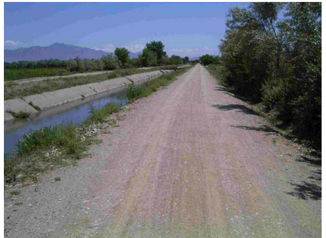
Photograph of the Canal Road in the province of Parwan, Afghanistan after rehabilitation (RIG/Manila auditor took the photograph in May 2005).
