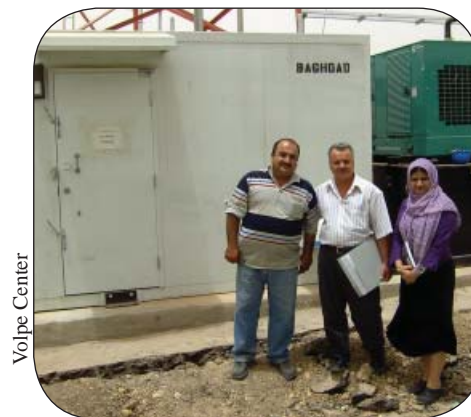
Iraqi team inspects telecommunications equipment shelter at the Bagdad site
