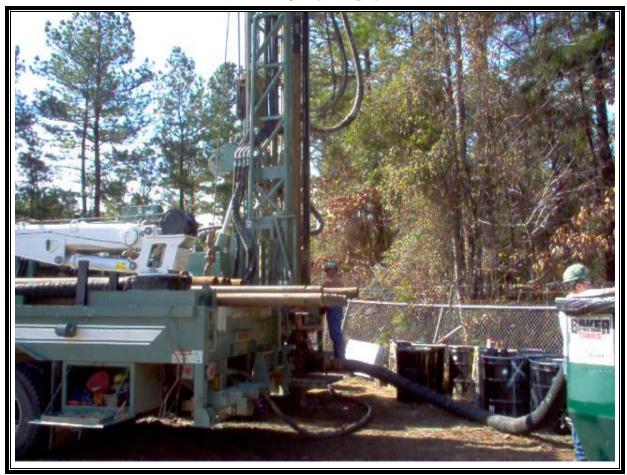
Photo Number: 053 Direction: South Photographer: Tim Osburn Witness: None Date: 02/23/07 Time: 0803 Logbook Photo Number: TO-03 **Description:** View of setting up of air rig at DW-3.
