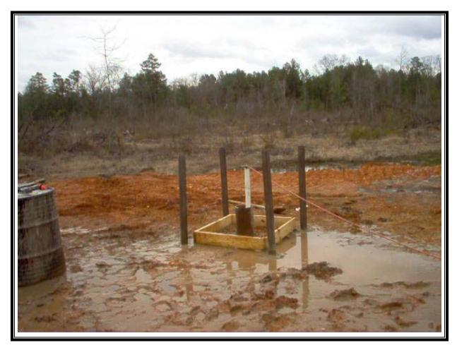
Photo Number: 072 Direction: East Photographer: Tim Osburn Witness: None Date: 03/13/07 Time: 1446 Logbook Photo Number: TO-14 **Description:** View of development of well at DW-4.
