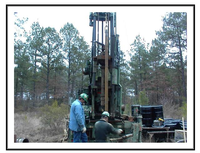
Photo Number: 094 Direction: East Photographer: Stephen Phillips Witness: Anna Cornelious Date: 2/8/2007 Time: 0902 Logbook Photo Number: SP-07 **Description:** NQ rods being lowered into borehole at DW-6
