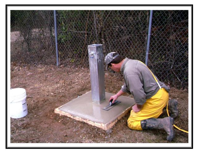
Photo Number: 031 Direction: North Photographer: Richard Hardy Witness: None Date: 2/12/2007 Time:1000 Logbook Photo Number: RH-13 **Description:** Construction of 6"x5' square stand with galvanized steel around SW-8
