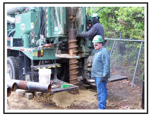
Photo Number: 067 Direction: East Photographer: Todd Quillen Witness: Date: 4/18/07 Time: 1104 Logbook Photo Number: TQ-02 **Description:** Setting the stem on wet gravel at DW-3L.
