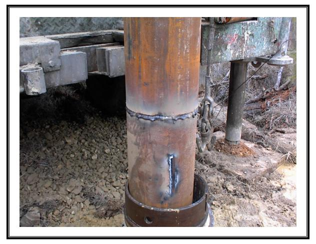
Photo Number: 083 Direction: N/A Photographer: Stephen Phillips Witness: Anna Cornelious Date: 2/10/2007 Time: 0953 Logbook Photo Number: SP-16 **Description:** Surface casing welded joint at DW-5.
