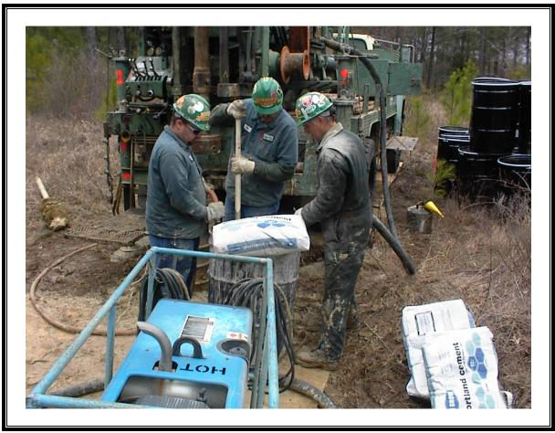
Photo Number: 092 Direction: East Photographer: Stephen Phillips Witness: Anna Cornelious Date: 2/7/2007 Time: 1507 Logbook Photo Number: SP-05 **Description:** Mixing of grout at DW-6 which included 460 lbs of Portland cement and 40 gallons of water.
