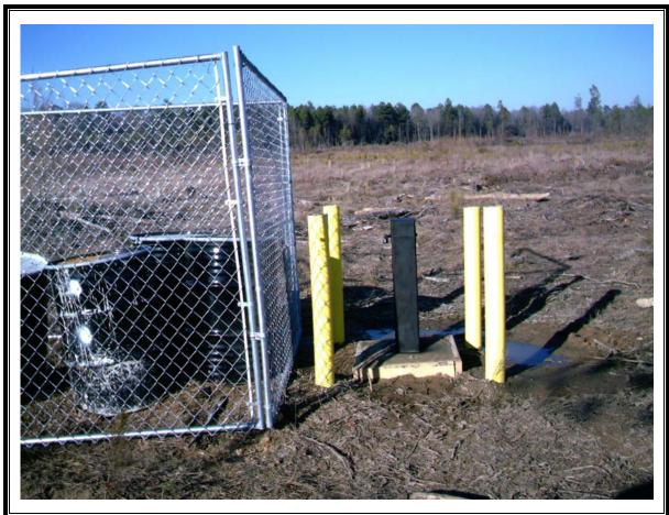
Photo Number: 034 Direction: North Photographer: Richard Hardy Witness: None Date: 2/16/07 Time: 1610 Logbook Photo Number: RH-19 **Description:** Black painted cover, completed pad and fenced IDW drums at SW-10
