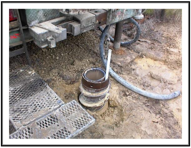
Photo Number: 084 Direction: N/A Photographer: Stephen Phillips Witness: Anna Cornelious Date: 2/10/2007 Time: 1015 Logbook Photo Number: SP-17 **Description:** Tremie pipe in place between surface casing and H.S. auger at DW-5.
