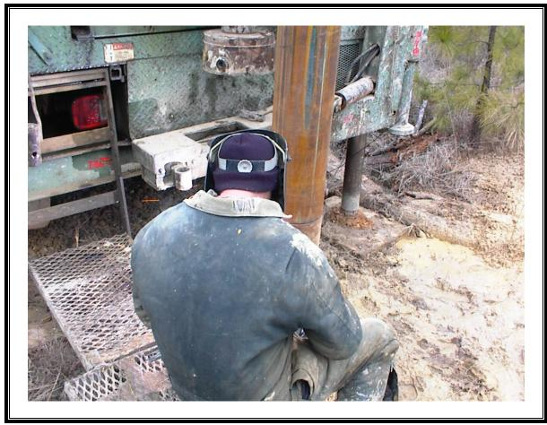
Photo Number: 082 Direction: N/A Photographer: Stephen Phillips Witness: Anna Cornelious Date: 2/10/2007 Time: 0945 Logbook Photo Number: SP-15 **Description:** Welding two sections of surface casing together at DW-5.
