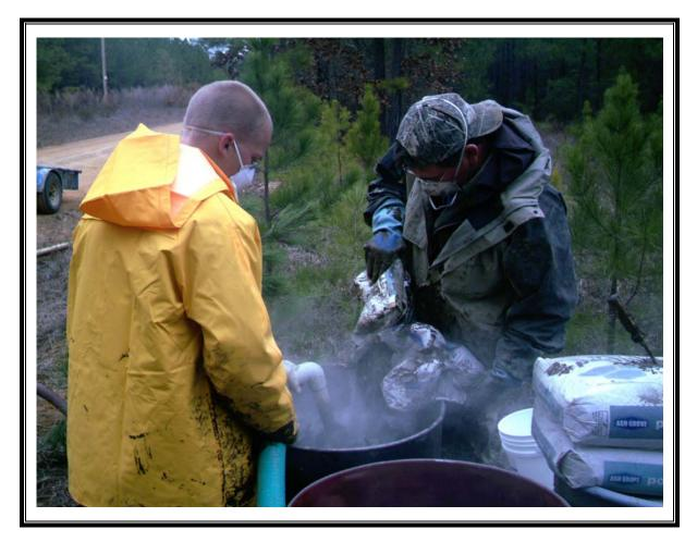
Photo Number: 016 Direction: Northeast Photographer: Richard Hardy Witness: None Date: 2/10/07 Time: 0840 Logbook Photo Number: RH-08 **Description:** Grout mixture; which comprised of 3 bags of Type 1 Portland cement, 15 lbs of 5% bentonite and 20 gallons of water, for the installation of SW-3
