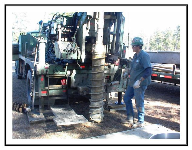
Photo Number: 037 Direction: N/A Photographer: Stephen Phillips Witness: None Date: 2/21/2007 Time: 1406 Logbook Photo Number: SP-25 **Description:** First H.S. auger in place to begin drilling at DW-1
