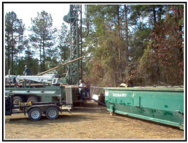
Photo Number: 051 Direction: South Photographer: Tim Osburn Witness: None Date: 02/23/07 Time: 0800 Logbook Photo Number: TO-01 **Description:** View of setting up of air rig at DW-3.
