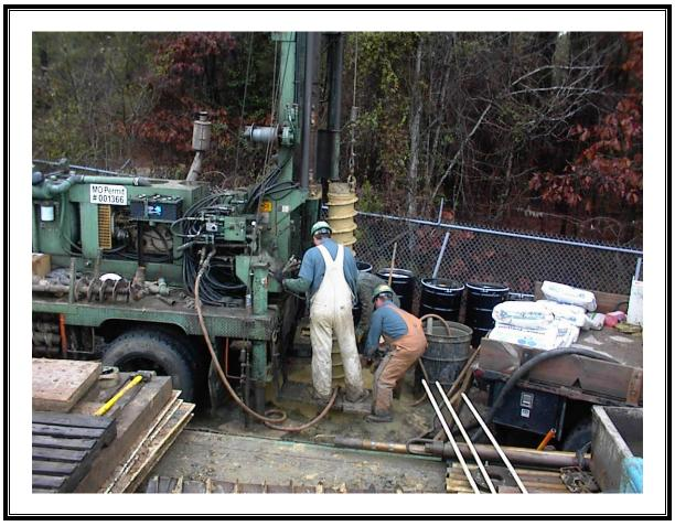
Photo Number: 047 Direction: West Photographer: Stephen Phillips Witness: Anna Cornelious Date: 2/13/2007 Time: 0840 Logbook Photo Number: SP-21 **Description:** Pulling of 5' of H.S. auger during grouting operations at DW-3
