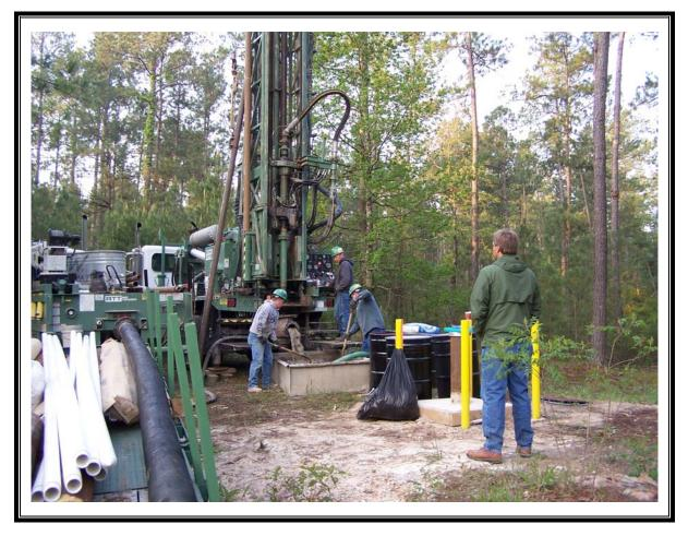
Photo Number: 044 Direction: South - Southwest Photographer: Todd Quillen Witness: Date: 4/22/07 Time: 0730 Logbook Photo Number: TQ-04 **Description:** Mud rotary drilling at DW-2L.
