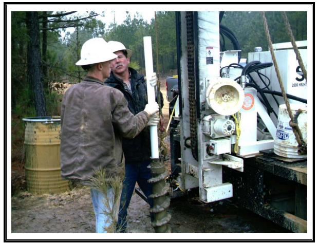
Photo Number: 006 Direction: South Photographer: Richard Hardy Witness: None Date: 2/7/07 Time: 1240 Logbook Photo Number: RH-06 **Description:** Installation of 10' screen with 6" point and 4-10' risers at SW-1.
