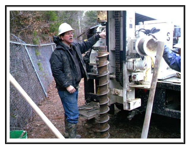
Photo Number: 030 Direction: South Photographer: Richard Hardy Witness: None Date: 2/10/2007 Time: 1130 Logbook Photo Number: RH-10 **Description:** Removal of the hollow-stem (HS) augers from the borehole at SW-8
