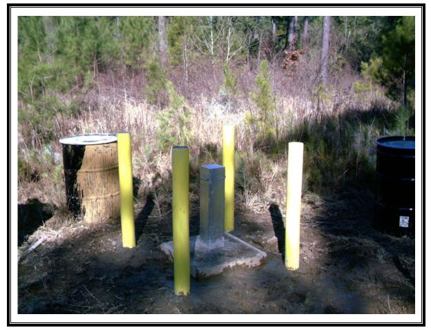
Photo Number: 007 Direction: East Photographer: Richard Hardy Witness: None Date: 2/16/2007 Time: 1130 Logbook Photo Number: RH-17 **Description:** Completed cement pad for SW-1 before IDW drums were removed
