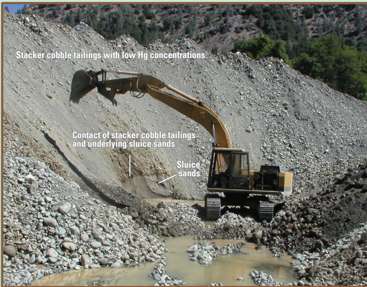
Sluice sands covered by stacker cobble tailings in the Trinity River Restoration Project. The sands and silts in the tailings contain much higher concentrations of mercury (Hg) than the coarser cobby material.
