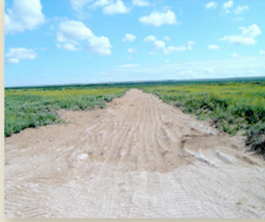
Caliche-packed roads can be reclaimed and restored. This restoration took place in one summer growing season. Caliche is a layer of calcium carbonate formed in the soils of semi-arid regions.
