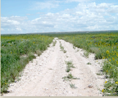
Caliche-packed roads can be reclaimed and restored. This restoration took place in one summer growing season. Caliche is a layer of calcium carbonate formed in the soils of semi-arid regions.
