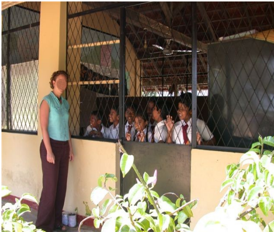
OIG photograph of the renovated Bundala secondary school, one of ten schools in Hambantota that benefited from the tsunami supplemental funding. Also shown in the photograph are the students from the school and DAI's regional program manager. (Hambantota, Sri Lanka, March 2007)
