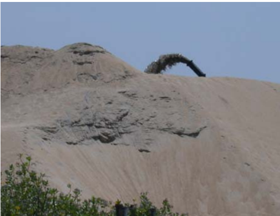
OIG photograph of the nozzle of the sand-conveying pipe spewing sand dredged from the mouth of the Kirinda harbor. (Hambantota, Sri Lanka, March 2007)
