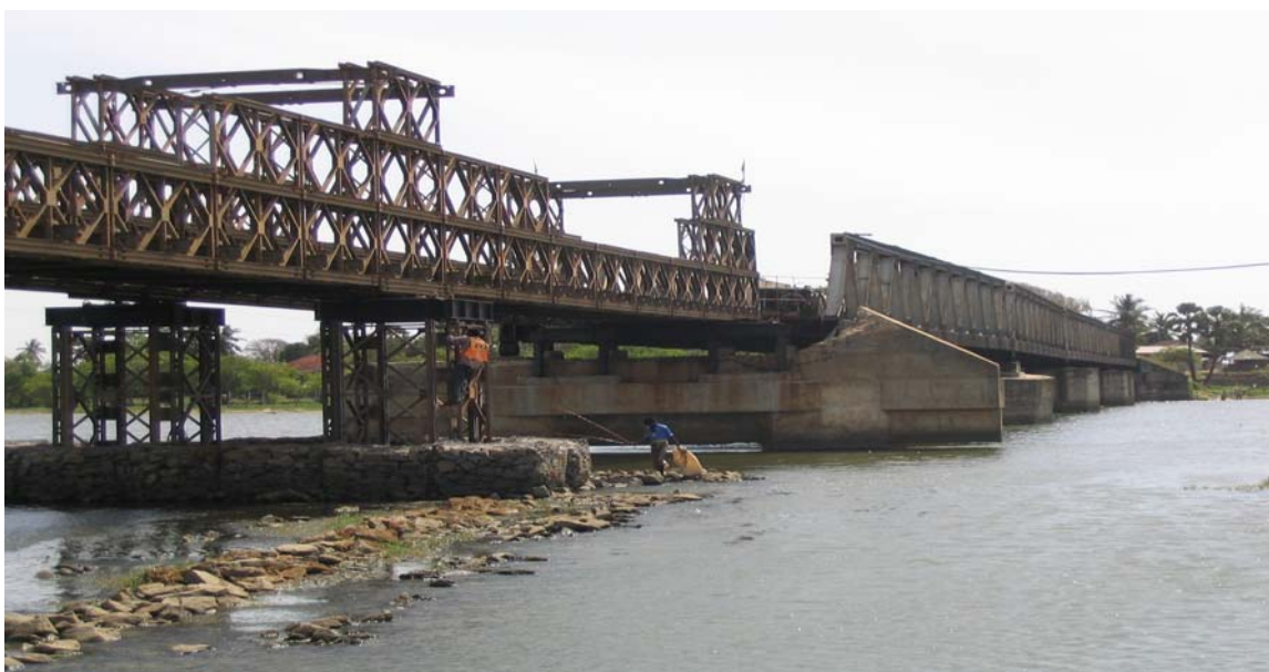
OIG photograph showing the half of the original steel-truss Arugam Bay Bridge that survived the tsunami connected to a temporary bailey bridge. A new bridge will be built adjacent to this one. (Arugam Bay, southeastern coast of Sri Lanka, June 2006)
