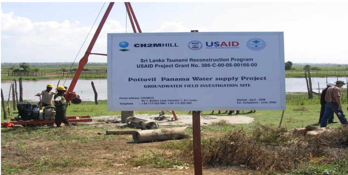
OIG photograph of drilling operations to determine the feasibility of using groundwater instead of surface water as the water source for the communities of Pottuvil and Panama, which are located along the eastern coast of Sri Lanka. (June 2006)
