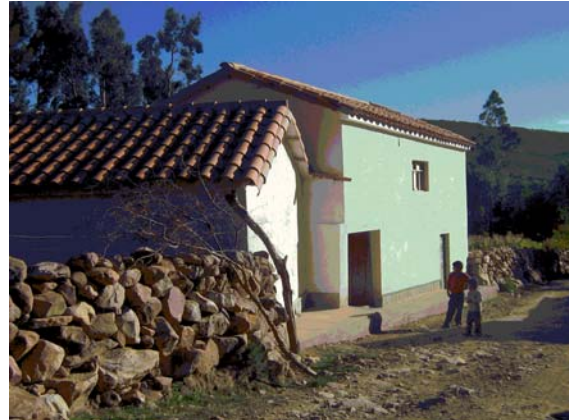
A house in Icla after renovation by Esperanza Bolivia's Chagas prevention housing improvement program. Photograph taken by a USAID/Bolivia employee during the OIG's visit to Chuquisaca, Bolivia on April 23, 2007.
