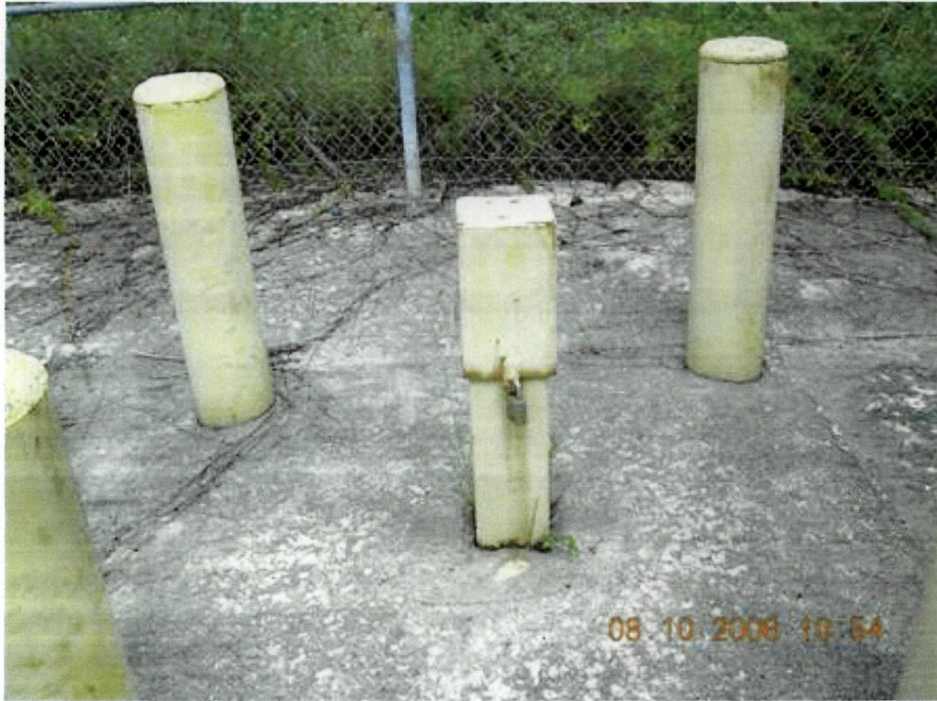
Photo 15: . View of monitor well GW-33. The outer casing is properly secured.
