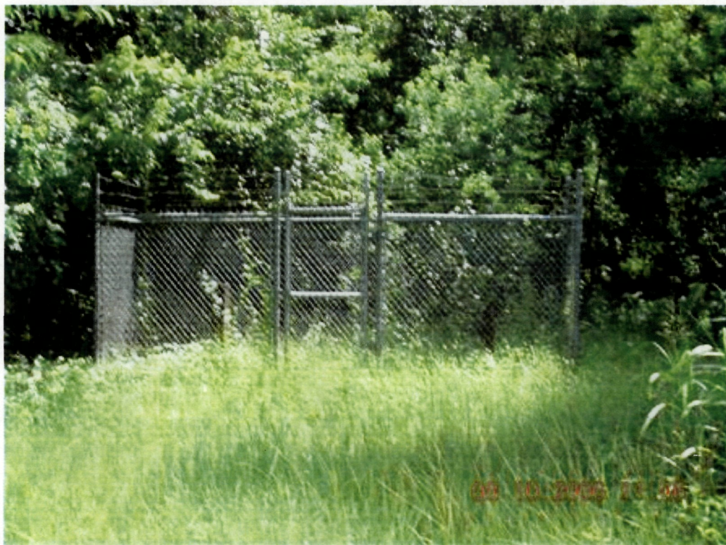
Photo 37: View of chain link fence at monitor wells SI-116 and INT-116.
