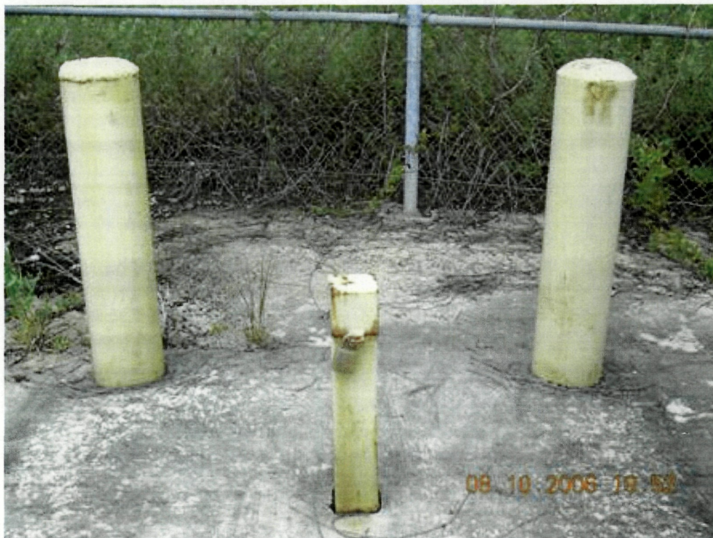
Photo 13: View of monitor well GW-32. The outer casing is properly secured.
