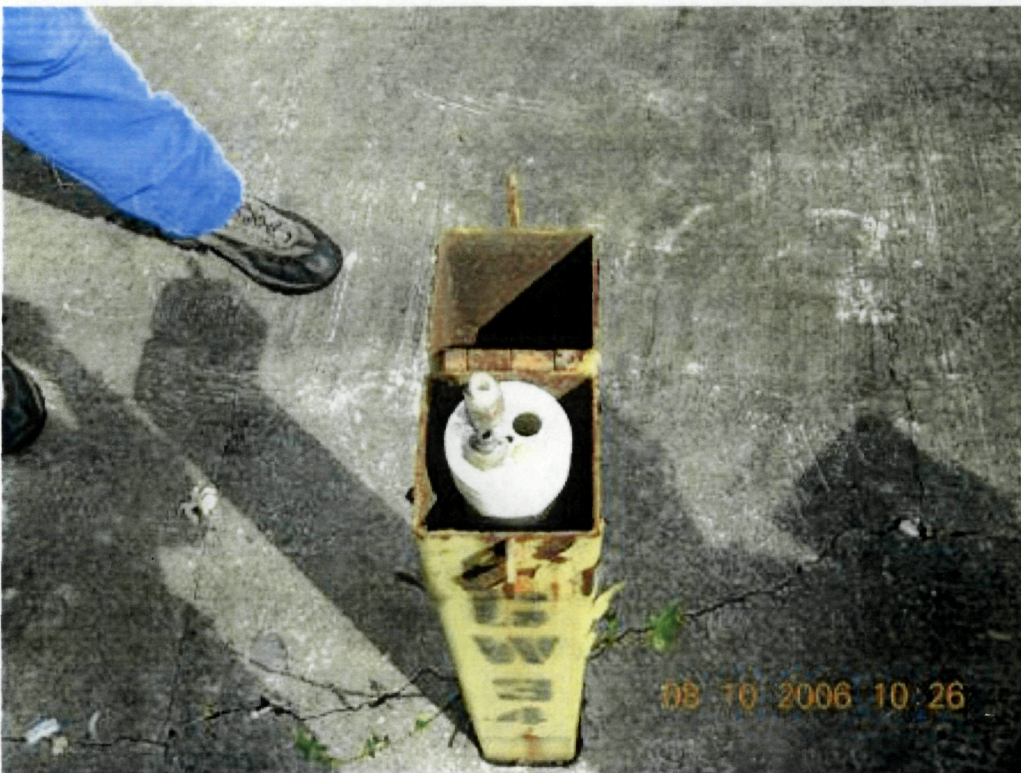
Photo 2: View of monitor well GW-34. A dust cap is missing from the well cap.
