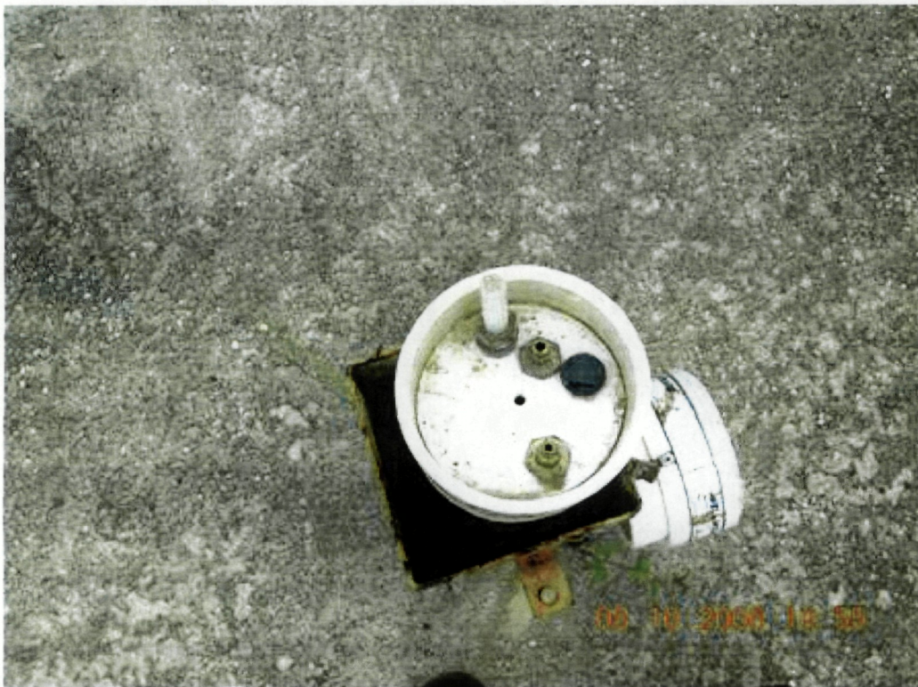
Photo 16: View inside outer protective casing at monitor well GW-33.
