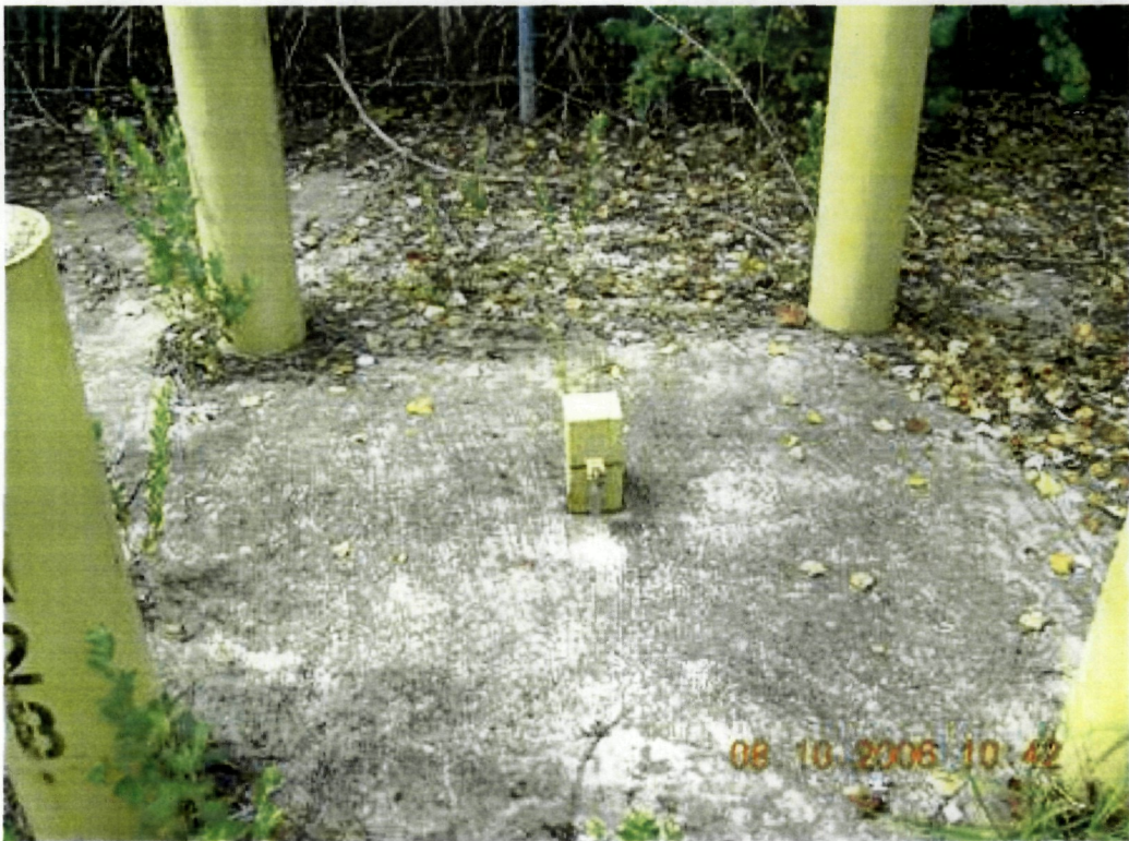
Photo 10: View of monitor well GW-28. The outer casing is properly secured.
