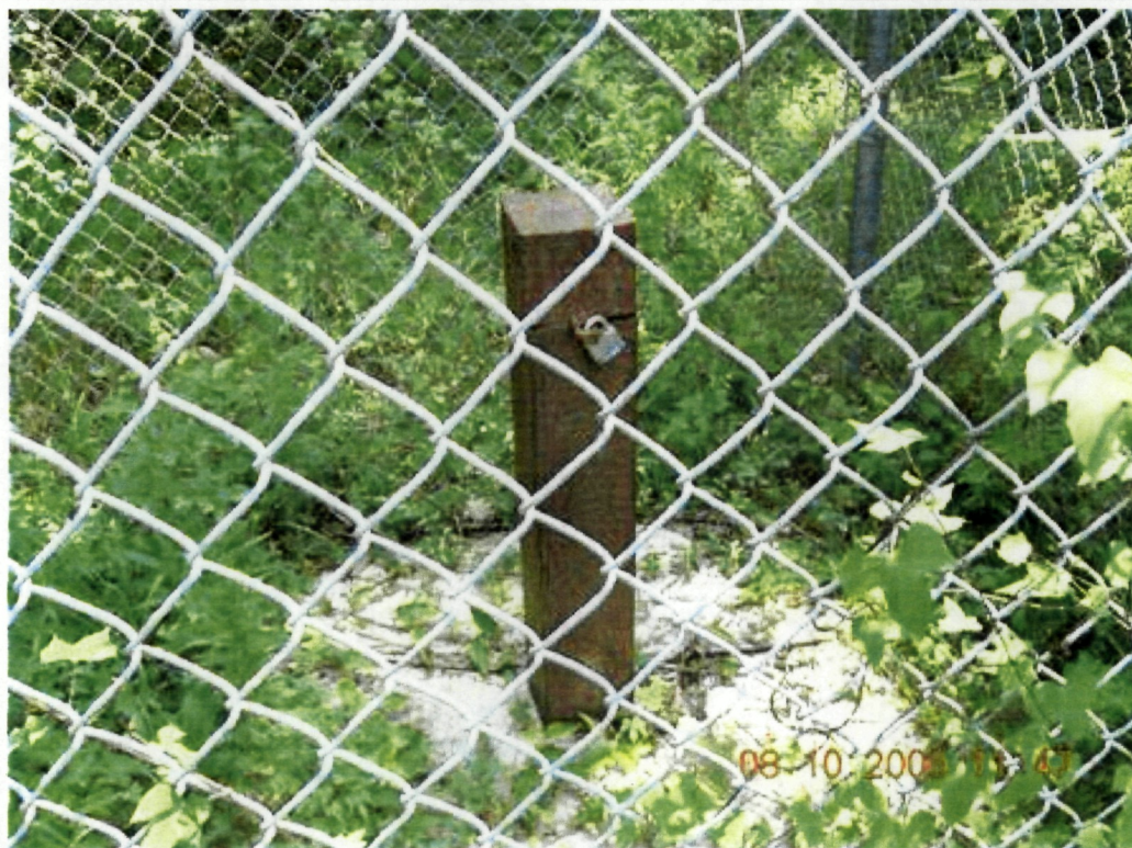
Photo 38: View of monitor well SI-116. The outer casing is properly secured.
