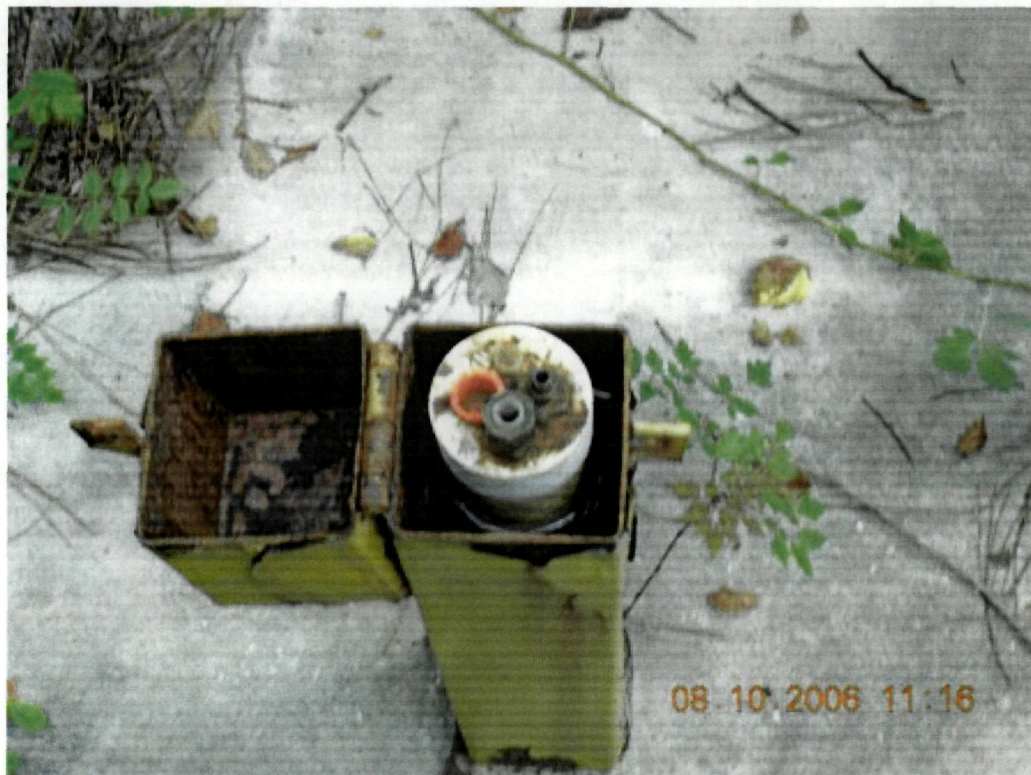
Photo 21: View inside outer protective casing at monitor well GW-35.
