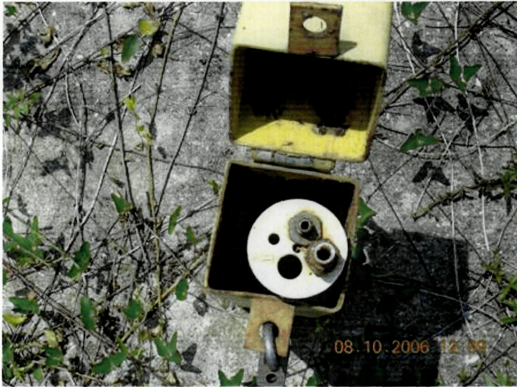
Photo 47: View inside outer protective casing at monitor well GW-30. A dust cap is missing from the well cap.
