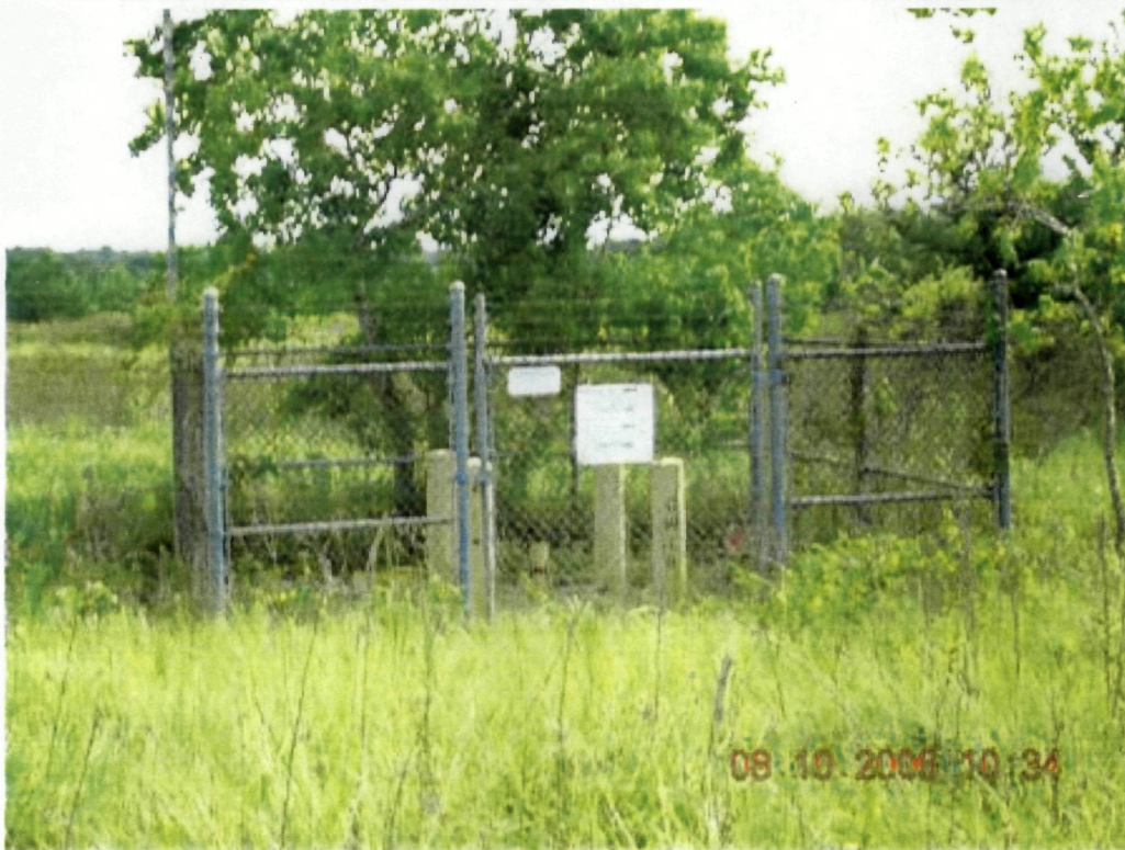
Photo 4: View of chain link fence at monitor well GW-18 facing northeast. Warning sign is still posted and in good condition.
