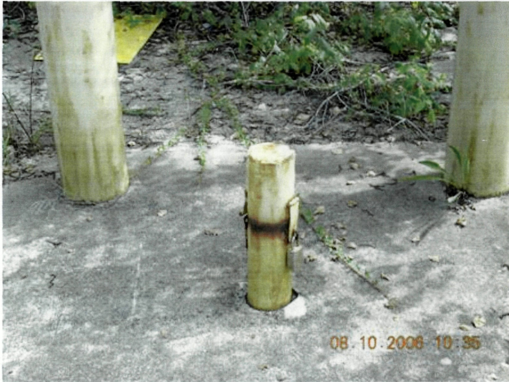
Photo 5: View of monitor well GW-18. The outer casing is properly secured.
