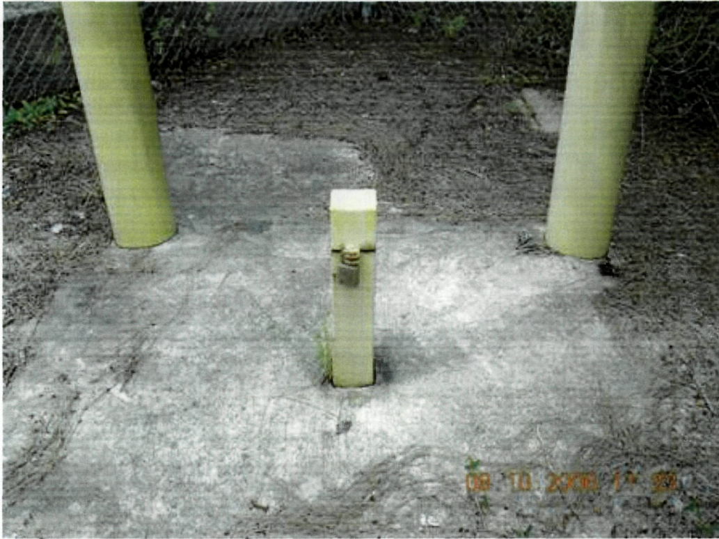
Photo 25: View of monitor well GW-27. The outer casing is properly secured.
