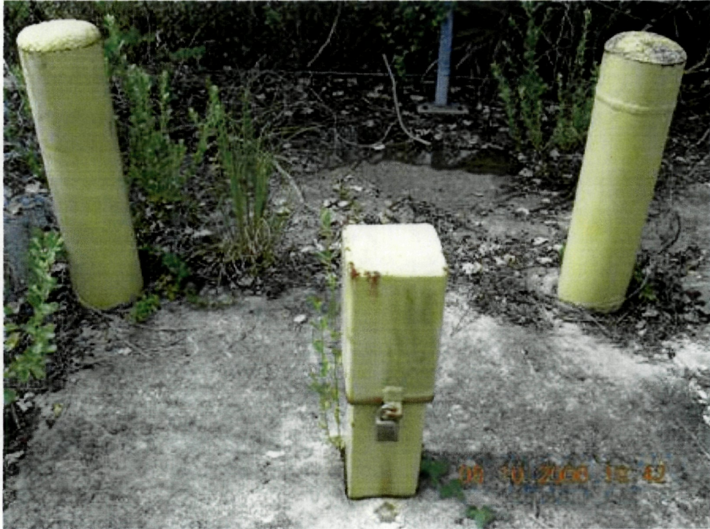
Photo 9: View of monitor well GW-29. The lock on the outer casing does not work.
