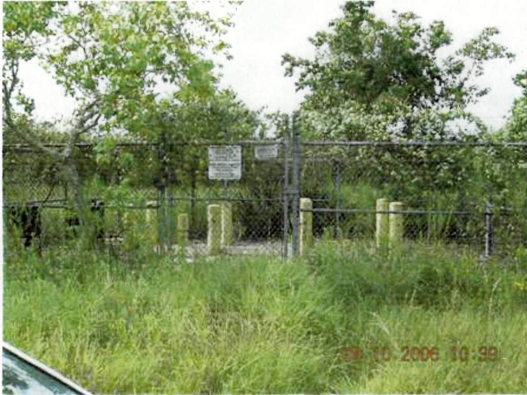
Photo 7: View of chain link fence at monitor well GW-28 and GW-29 facing south. Warning sign is still posted and in good condition. Three drums are present inside the fence to the left.
