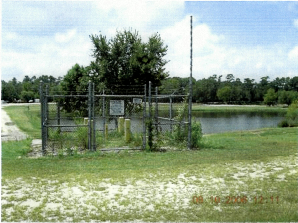
Photo 49: View of west pond facing southwest at monitor well GW-30.
