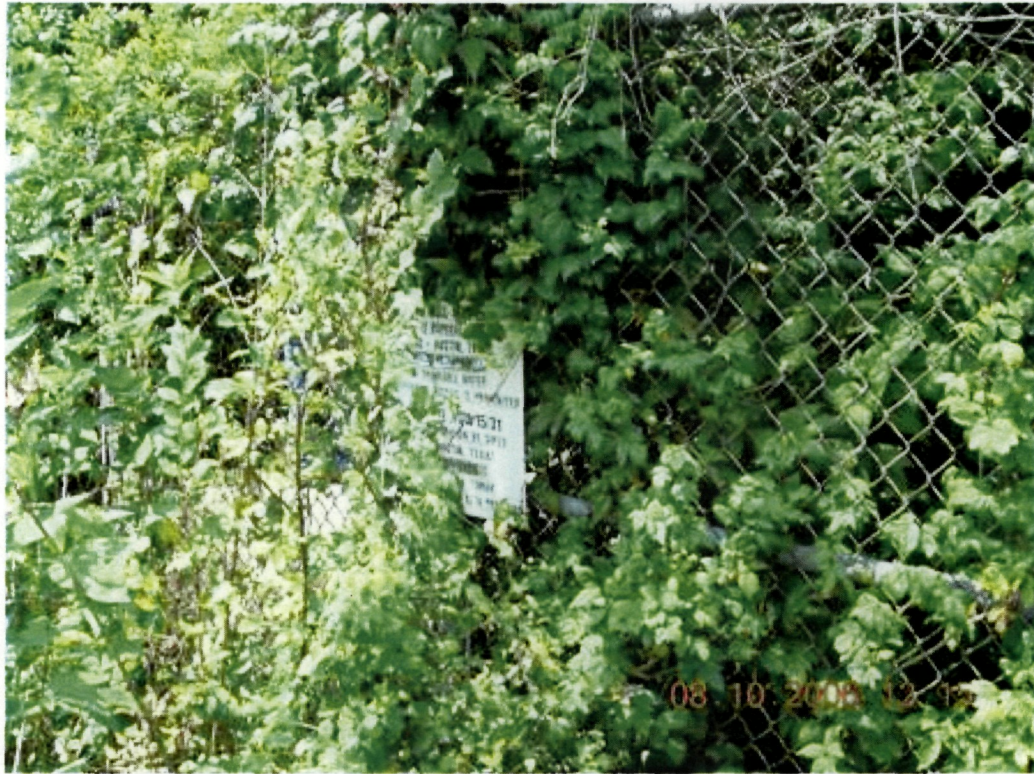
Photo 53: Warning signs are posted and in good condition at monitor wells GW-15 and GW-31.
