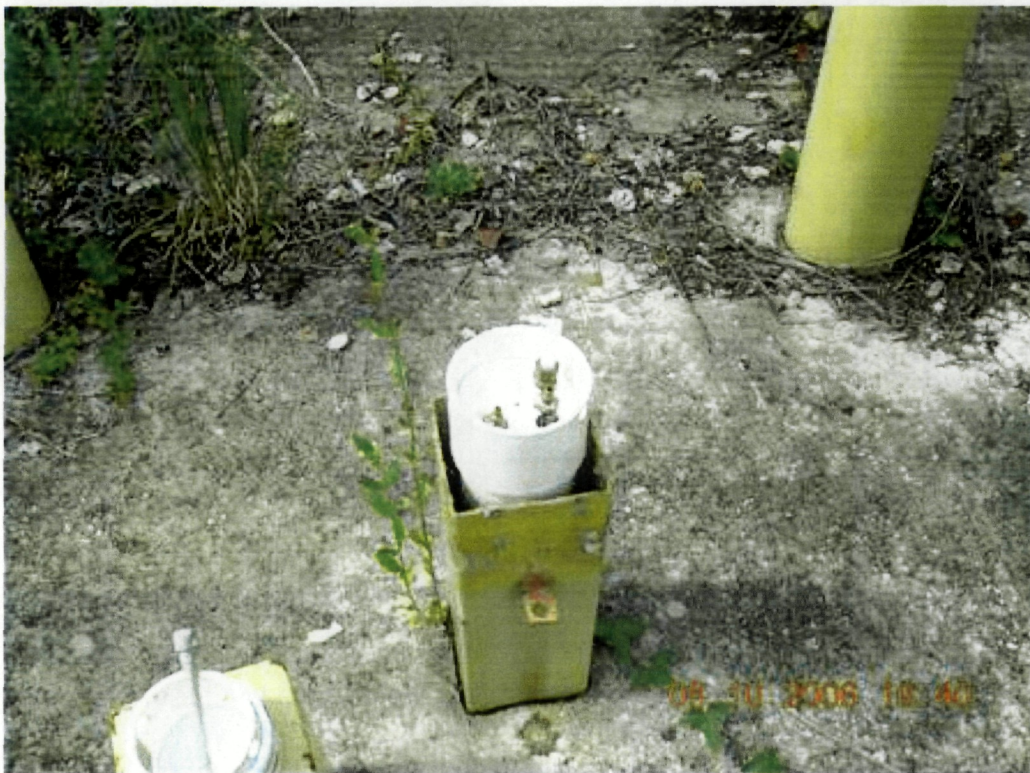
Photo 8: View inside outer protective casing at monitor well GW-29.
