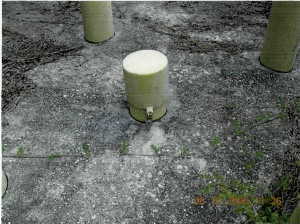
Photo 27: View of monitor well GW-21. The outer casing is properly secured.
