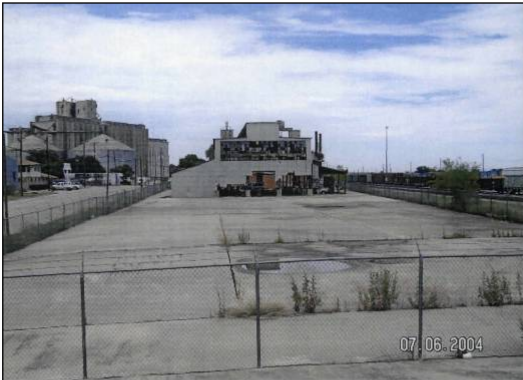
View to the north across concrete paved South Storage Yard From the Containment Cell Cap
