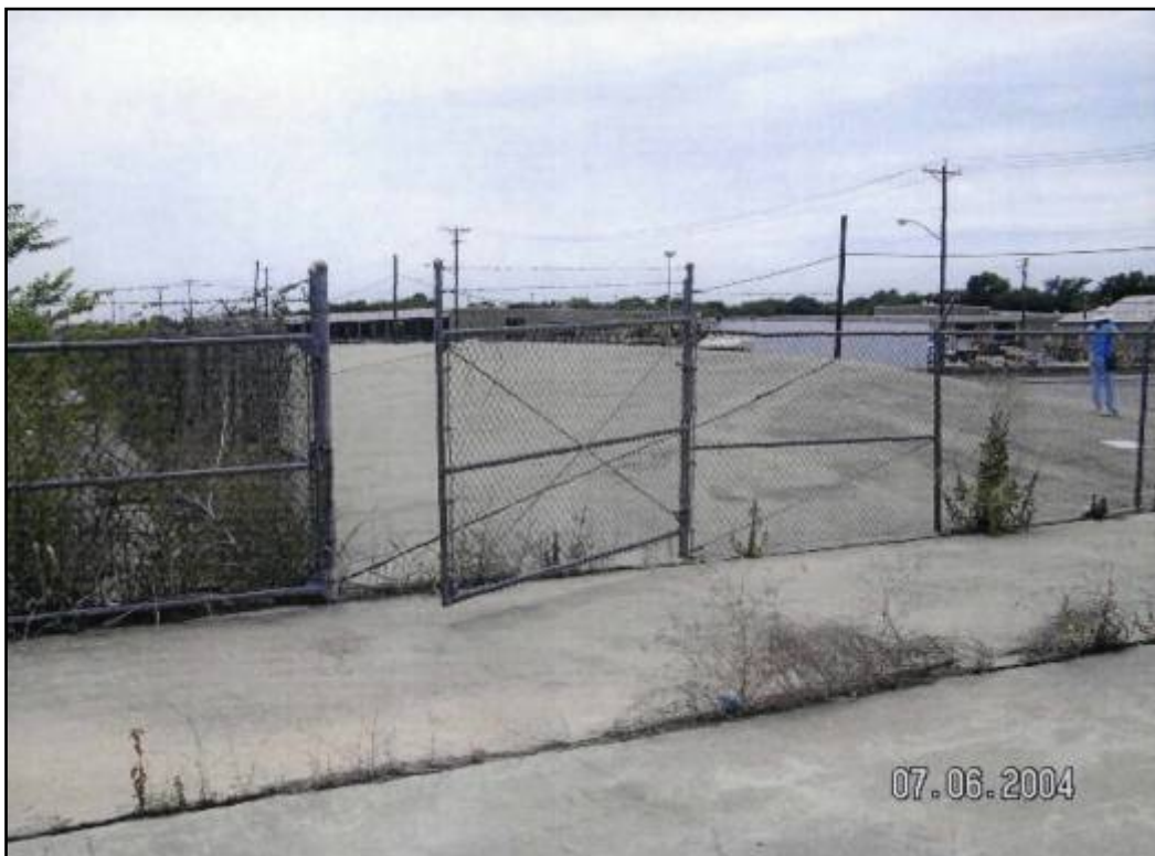
Containment Cell View to southwest from the concrete paved South Storage Yard
