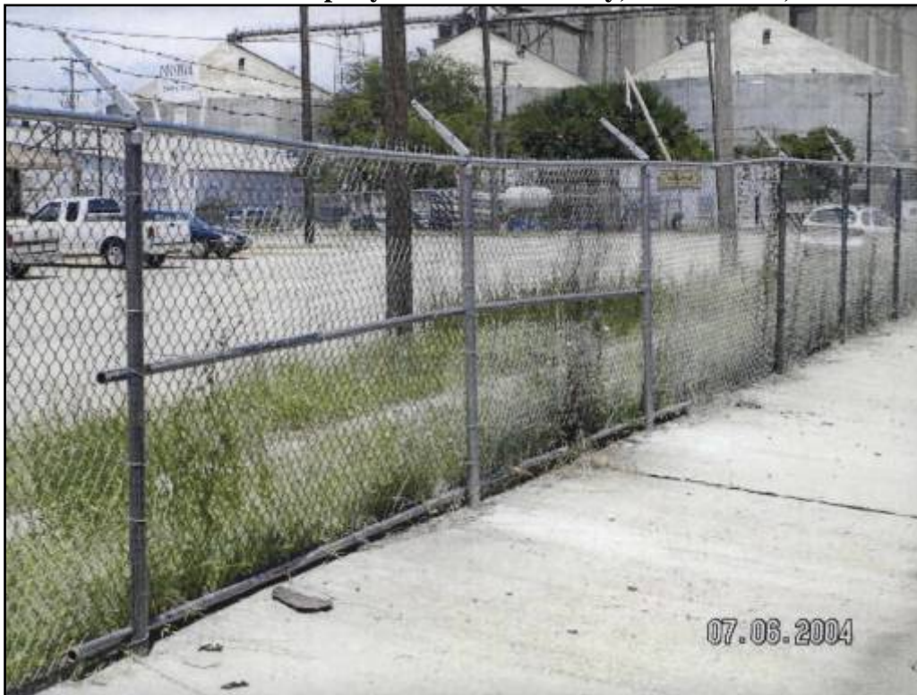
View to Northwest from the Metal warehouse Fence Repair Area
