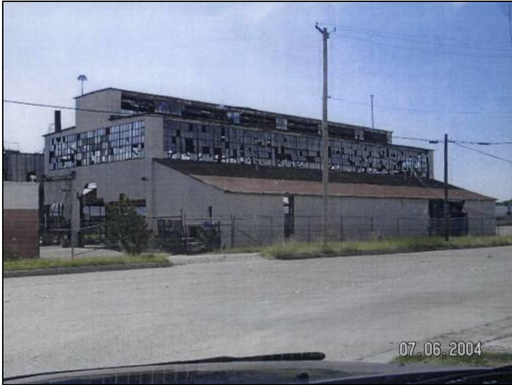
Metal Warehouse View to southwest across South Main Street
