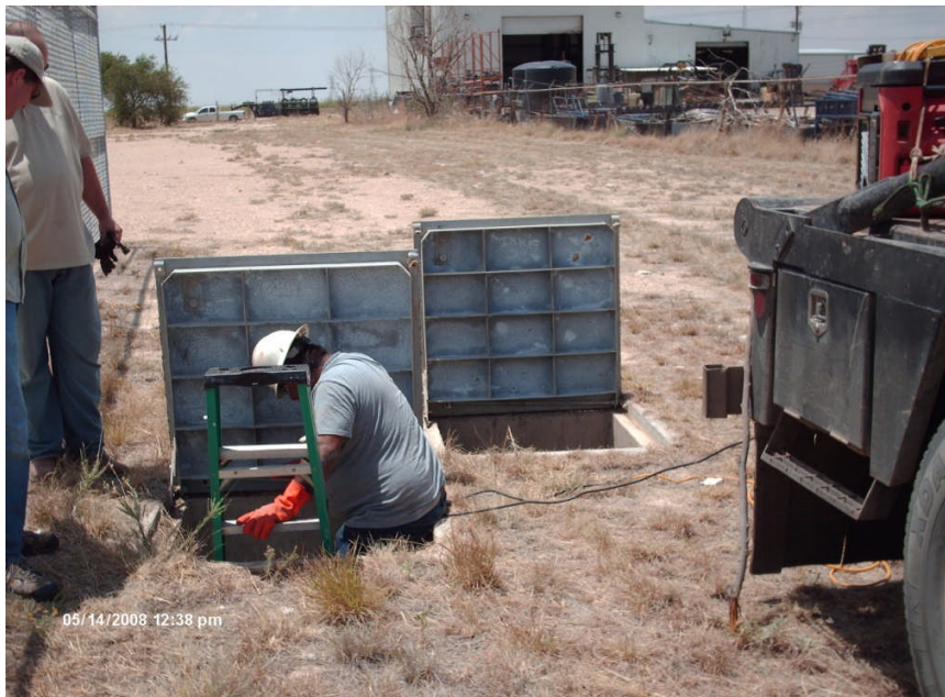
Photograph No. 3 Site: Sprague Road Ground Water Plume Superfund Site Description: View of contractor drilling drainage holes in flooded electrical pull boxes at the M&C facility. Date: 14 May 2008
