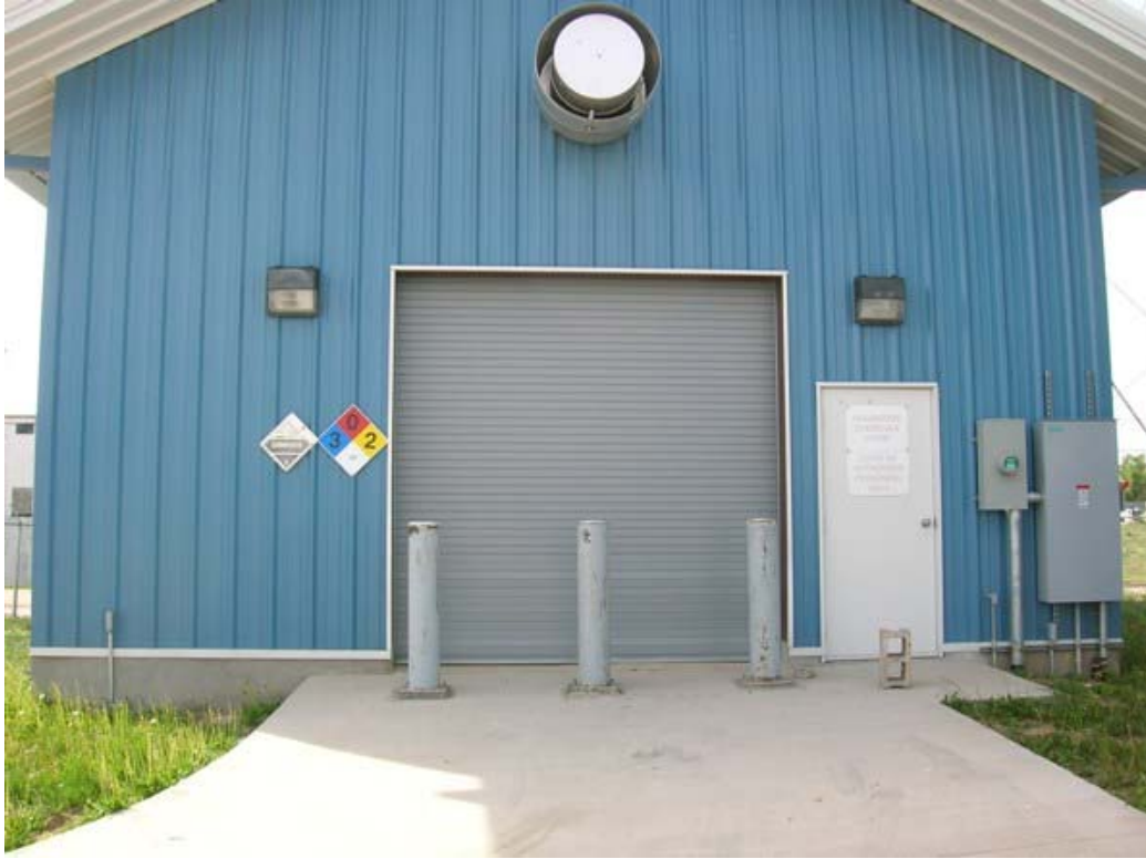
Photo 5: North side of Reverse Osmosis (RO) Facility building.
