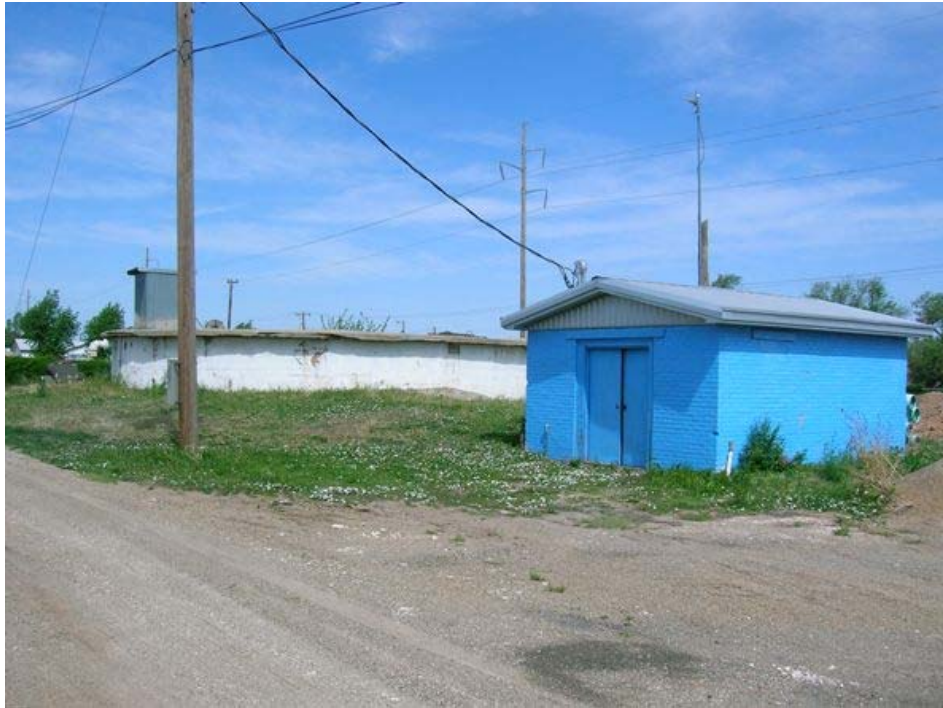
Photo 27: North Groundwater Storage Tank (NGST).
