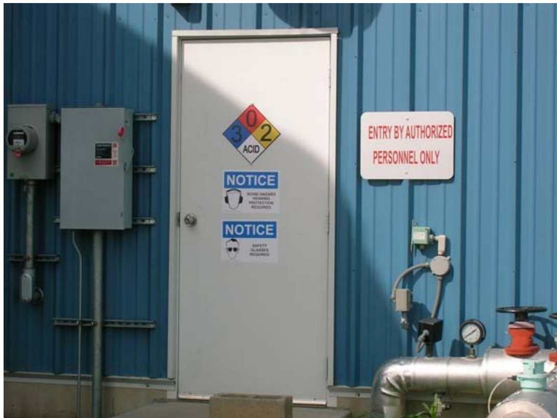
Photo 4: Entrance door on east side of ASTP building.
