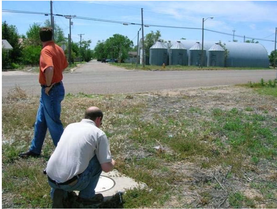
Photo 40: View of MWCL-13 D/S looking south.
