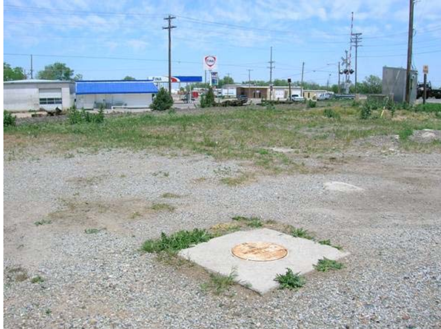
Photo 41: View of MPMW-06 looking north.
