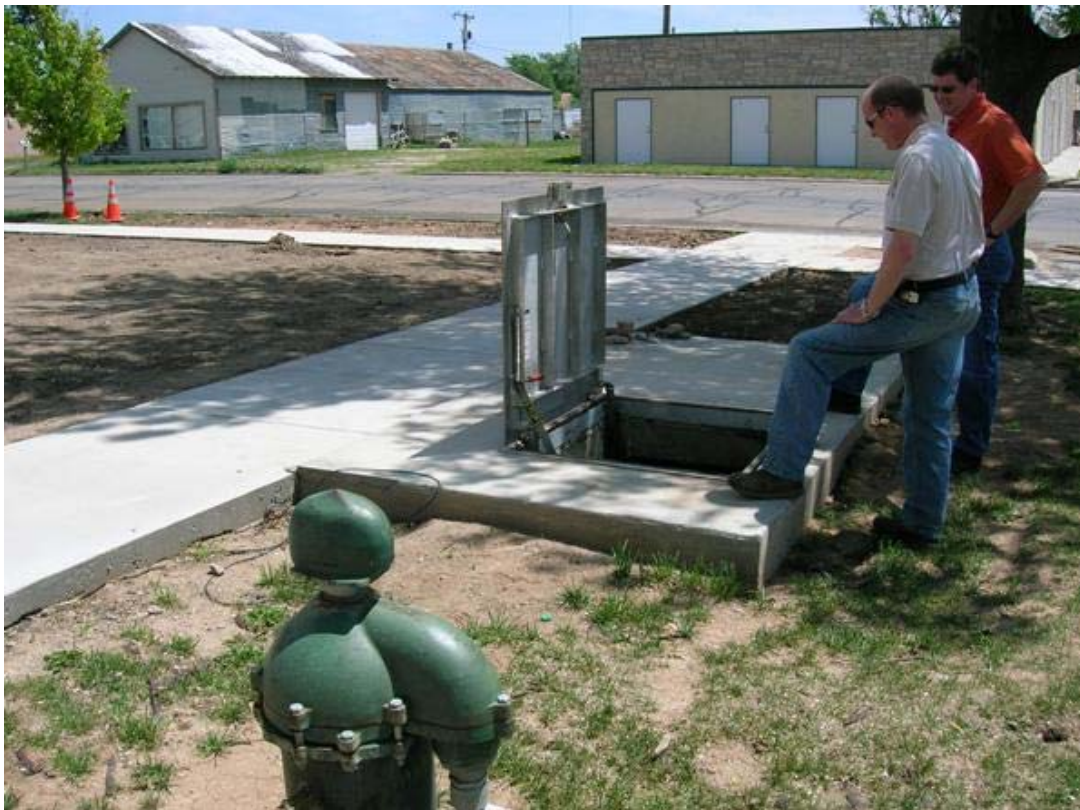
Photo 36: MW-17-EX well vault in front of City of Perryton City Hall.
