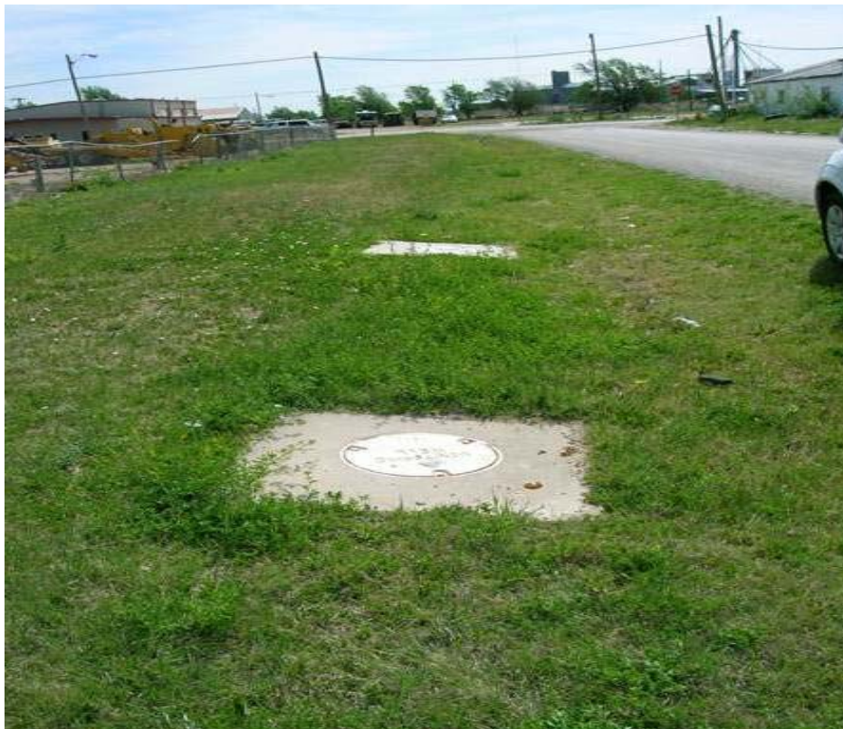
Photo 28: View of MW-5 D/S looking east.
