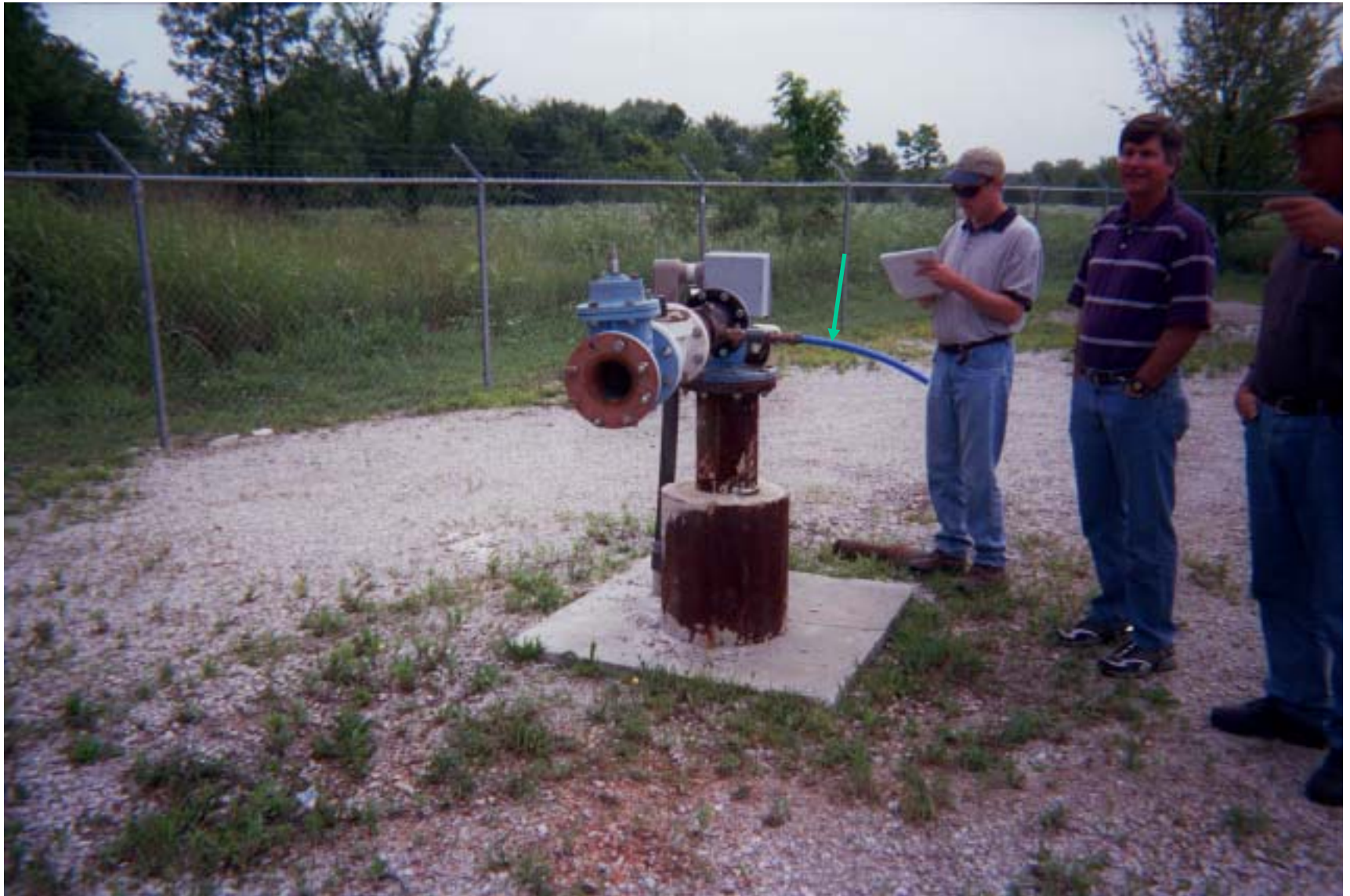
Photo 51: View of Quapaw #5 MW. Sampling tube is located at green arrow.
