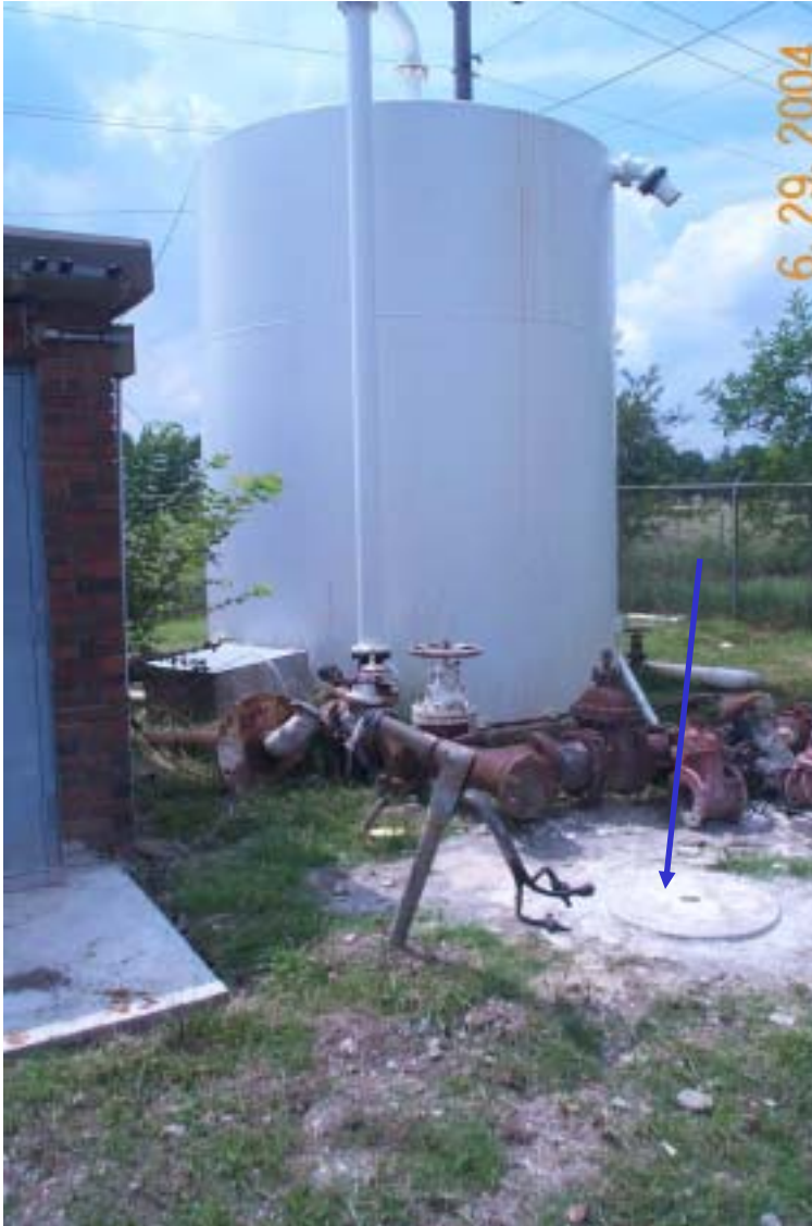
Photo 2: View of the plugged Commerce #3 well (blue arrow). White tank in background receives and stores water from the Commerce #4 well (located to the east of this location). Building at left is where chlorine is added to the water prior to entry into drinking water system.
