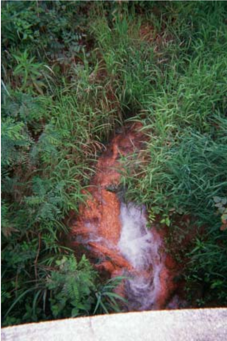
Photo 75: View of old Lytle Creek channel, just prior to its confluence with Tar Creek. Photo taken from the Douthat Bridge. Red staining is iron oxide deposition. The iron oxide precipitates out of the water and is deposited in the stream bed.
