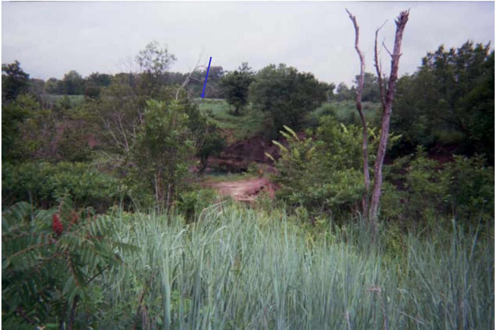
Photo 59: View of subsidence at the Big John Mine site, located in Kansas, facing northwest. This subsidence feature is surrounded by a diversion dike to prevent inflow of water into the mines. Tar Creek was diverted around the subsidence to the west (behind dike in background at blue arrow).
