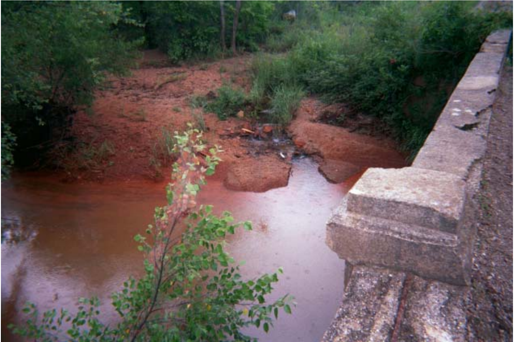
Photo 76: View of the downstream side of Tar Creek at the Douthat Bridge. The color of the water in the stream is red and orange from iron oxide precipitating out of solution in the water. Note the red staining on the shore, where the iron oxide has been deposited by the stream.
