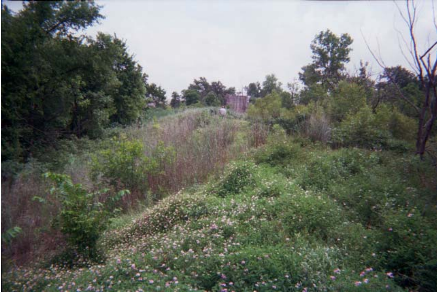
Photo 58: View of diversion dike at the Big John Mine site, located in Kansas.
