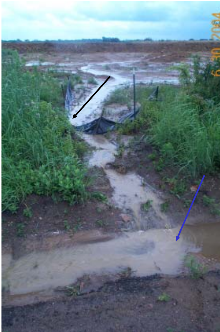
Photo 49: View of drainage ditch and runoff discharge point from borrow source property. The silt curtain erected across the discharge point has collapsed (black arrow). Water in the drainage ditch becomes discolored where runoff enters from the borrow source property (blue arrow).
