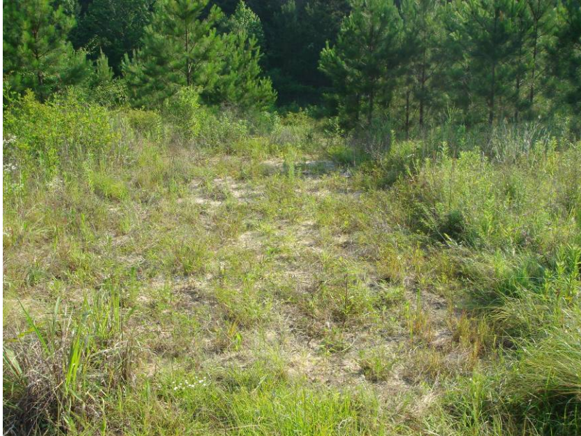
Photo 3. Eroded area on top of landfill cell. Picture taken facing east in May 2006.
