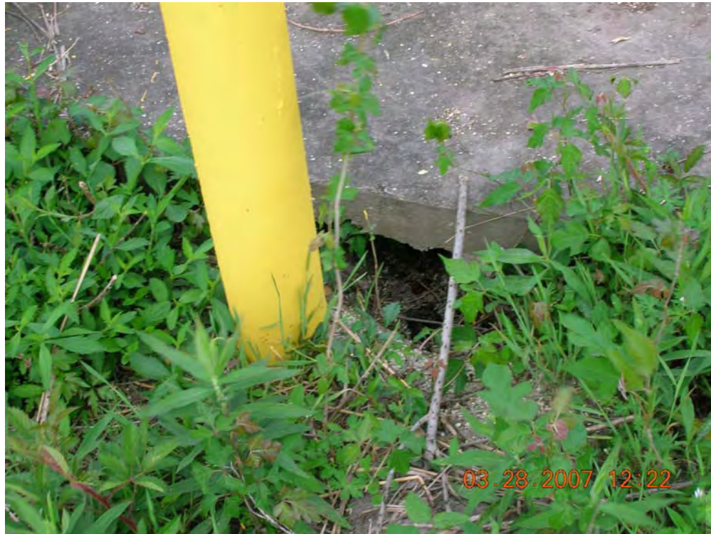
Photograph No. 5 Description: Animal burrow under MW-8 well pad
