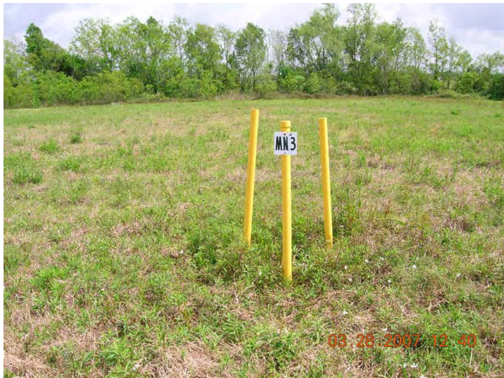
Photograph No. 6 Description: Cap elevation monument MN-3
