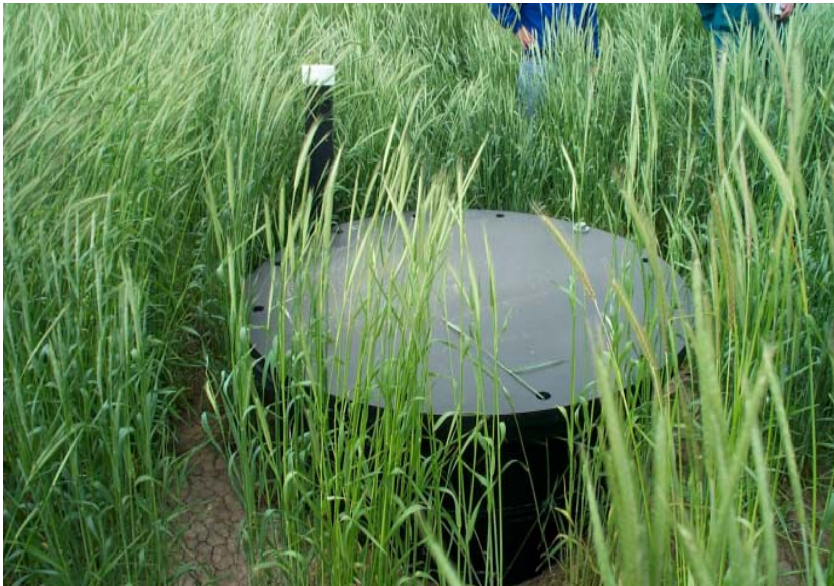
Photograph 23: Landfill sump, hazardous waste landfill.
