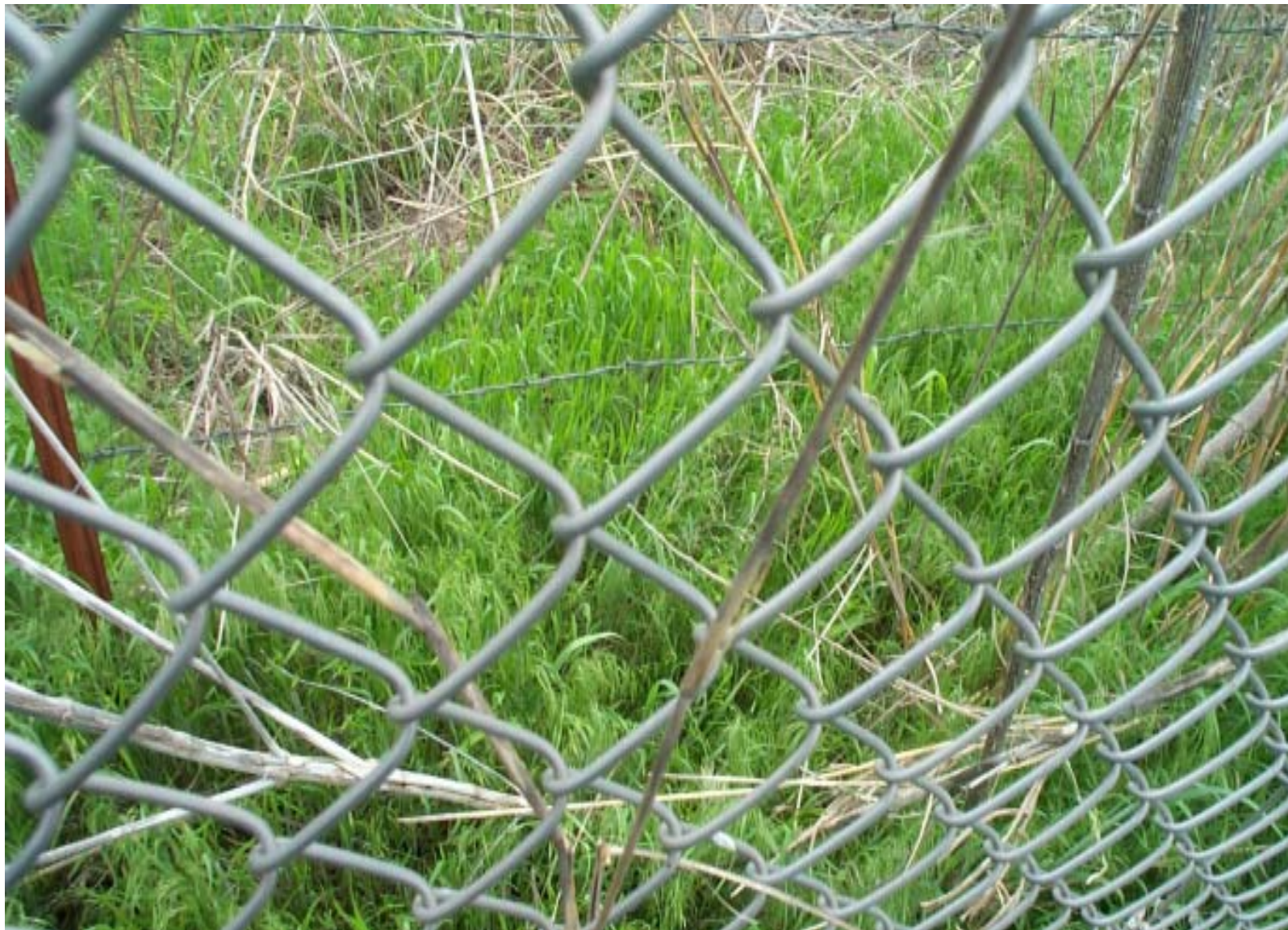
Photograph 16: East perimeter fence.
