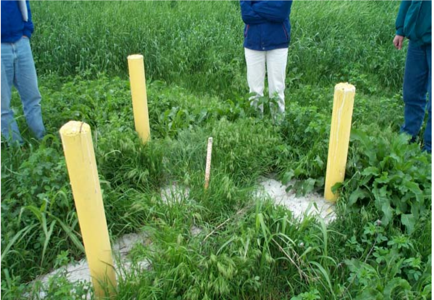
Photograph 3: Settlement monument on non-hazardous waste landfill.
