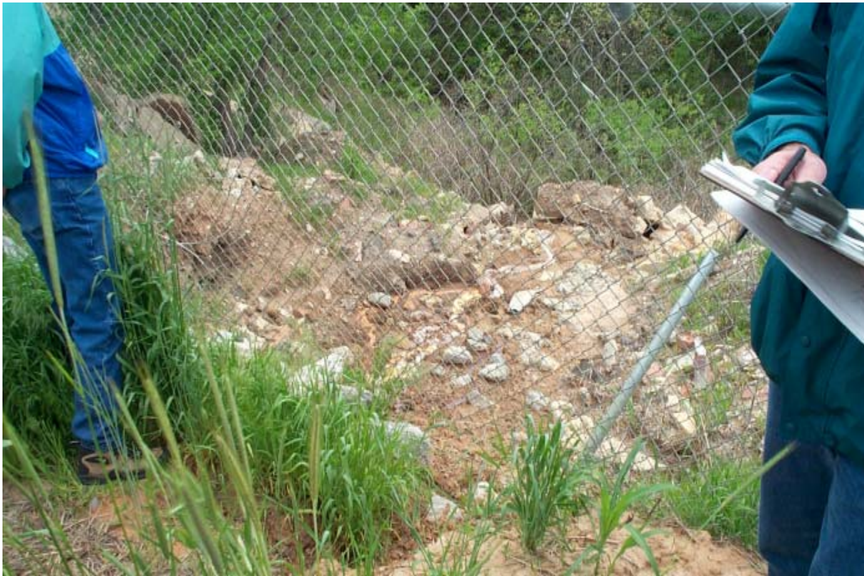
Photograph 14: Looking east through east perimeter fence, at Gladys Creek.
