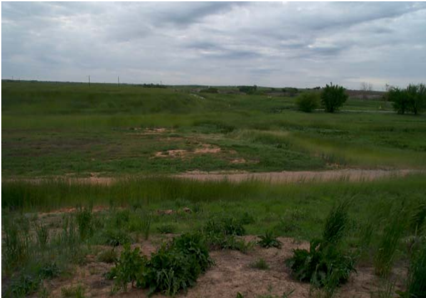
Photograph 4: Looking east from non-hazardous waste landfill across access road to hazardous waste landfill.
