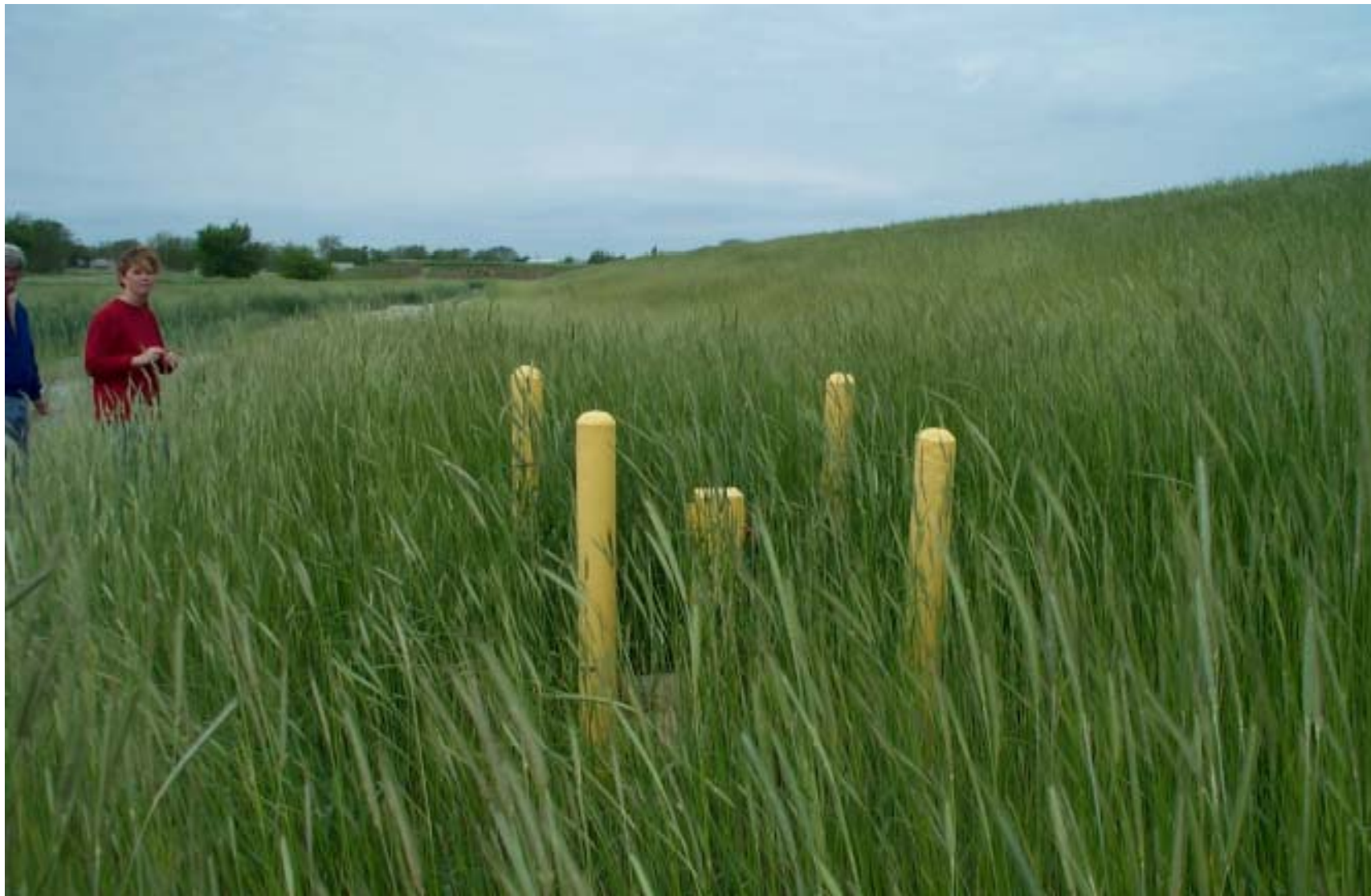
Photograph 25: Ground water monitoring well at south embankment of hazardous waste landfill.
