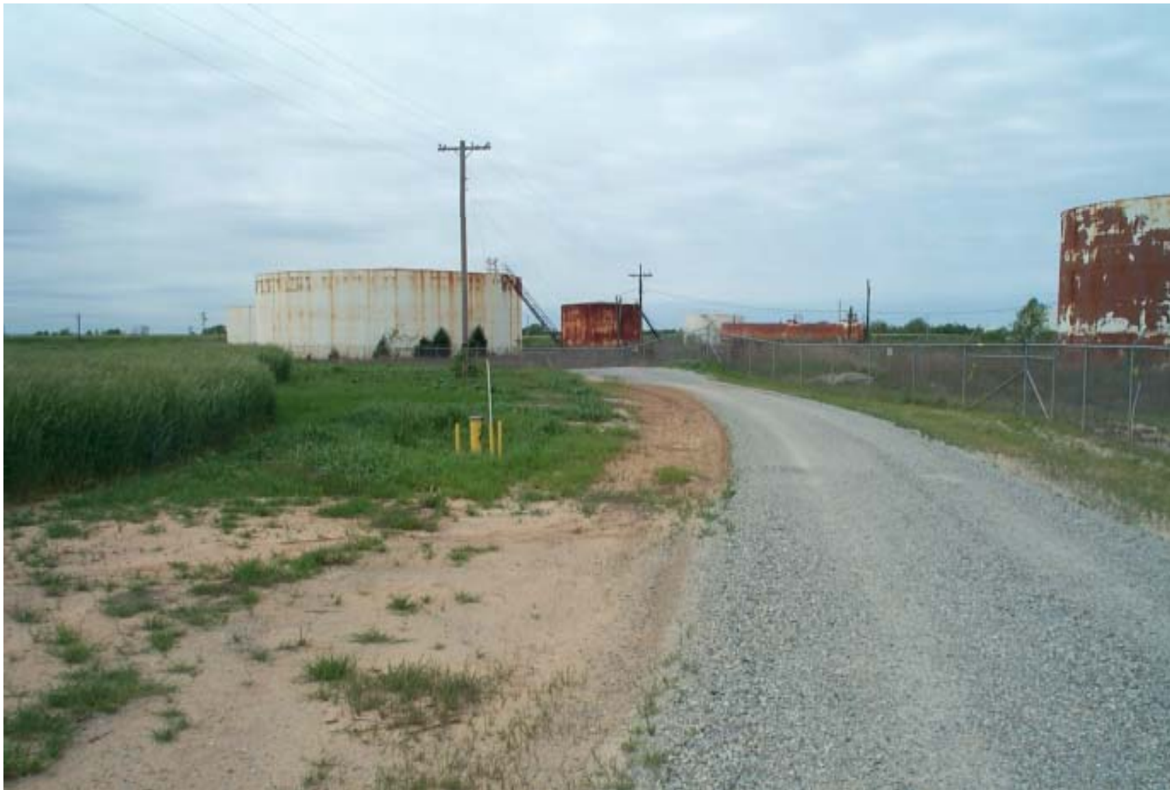
Photograph 19: Looking south towards CPC storage tanks.
