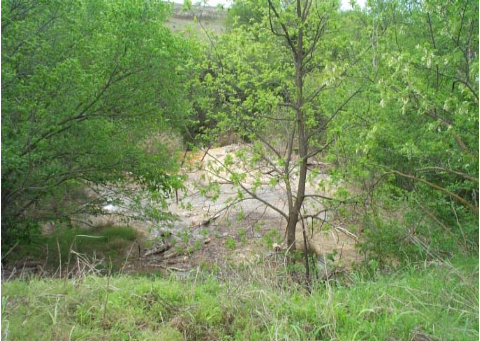
Photograph 10: Looking south, offsite at drainage feature/tributary to Gladys Creek.
