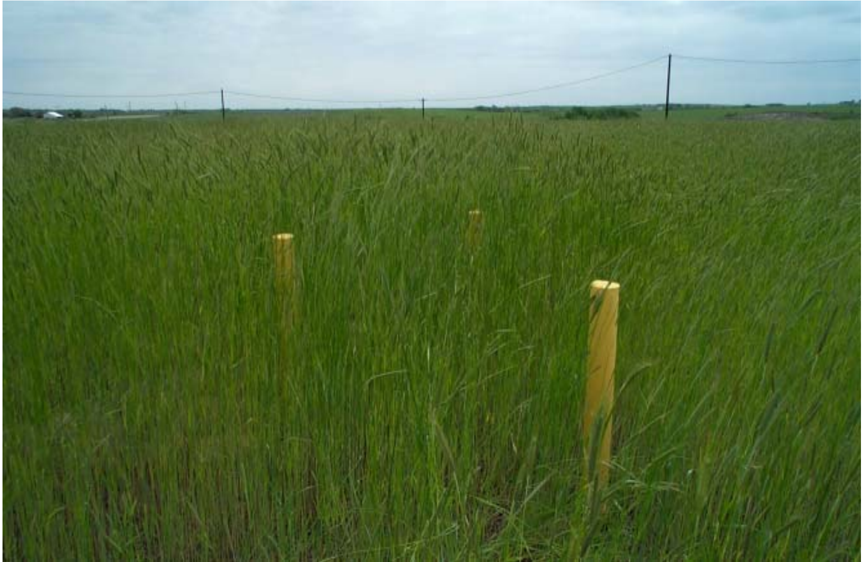
Photograph 20: Settlement monument on hazardous waste landfill.
