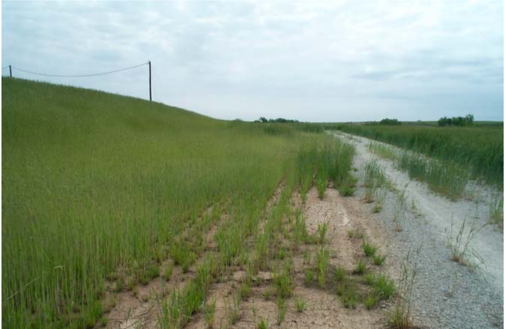
Photograph 24: Wheat cover on south embankment of hazardous waste landfill.
