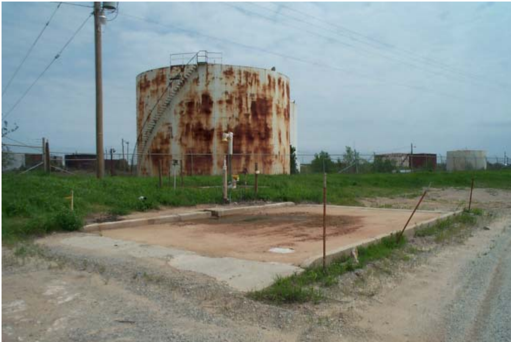
Photograph 35: On-site decon pad, CPC property with storage tanks in background.
