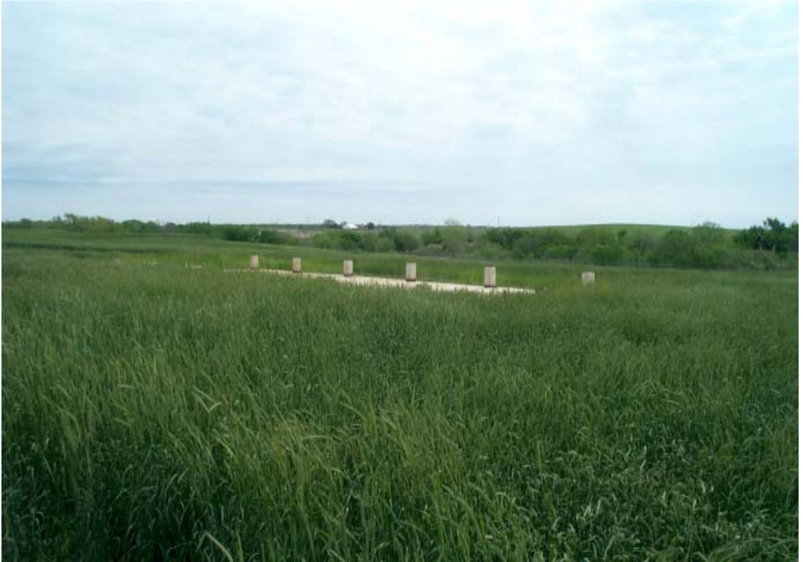
Photograph 26: Concrete foundation of former water treatment facility.
