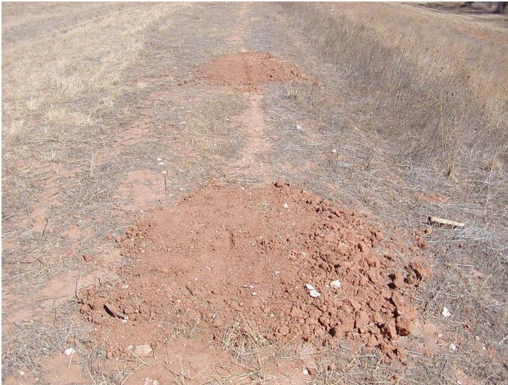
Repair of soil disturbance on landfill cap
