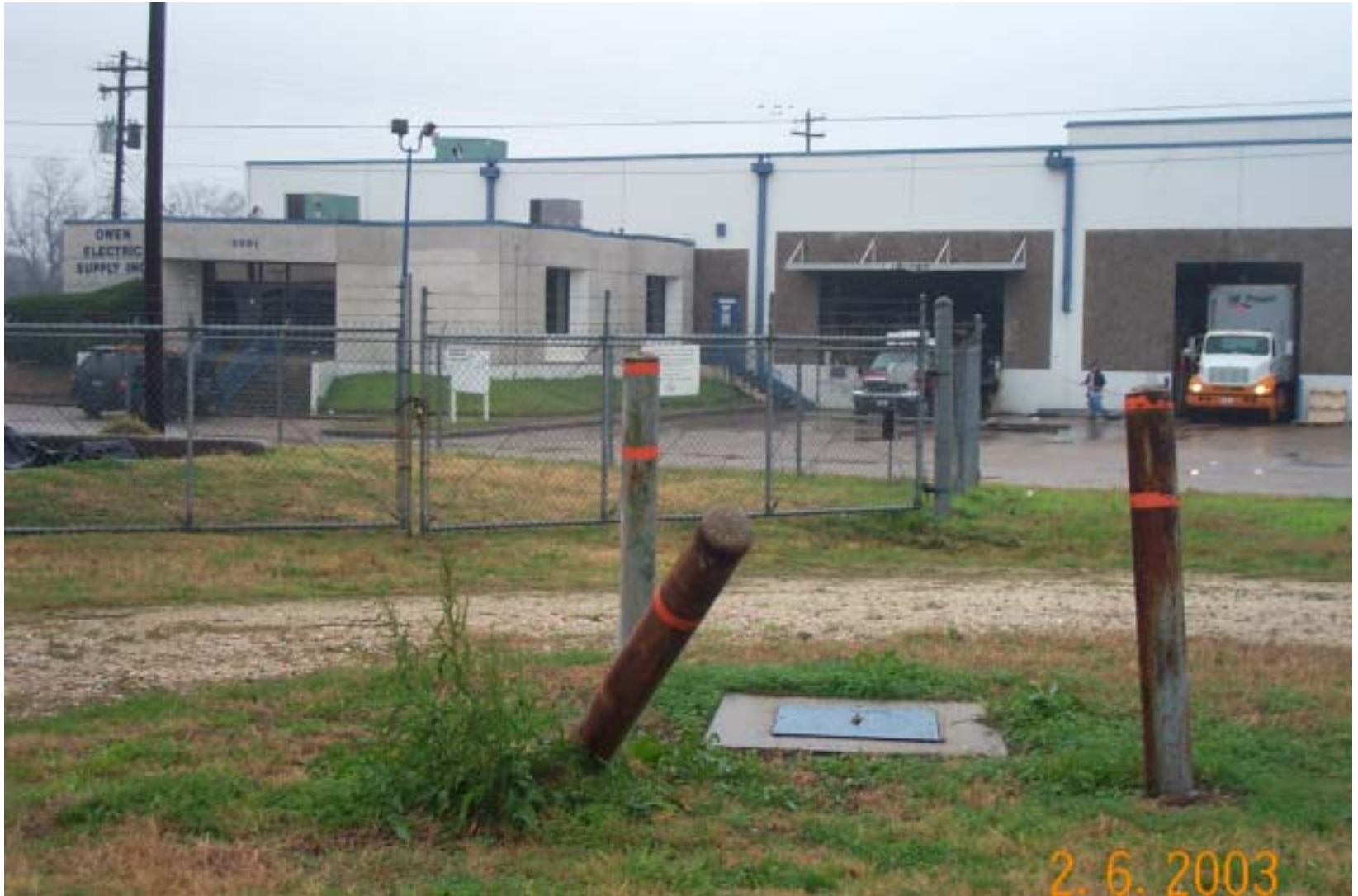
Looking west towards Owens Electrical Supply Inc. An extraction well is in the foreground/one of the protective posts is bent. The groundwater treatment system is to the left of the photograph inside the security fence.
