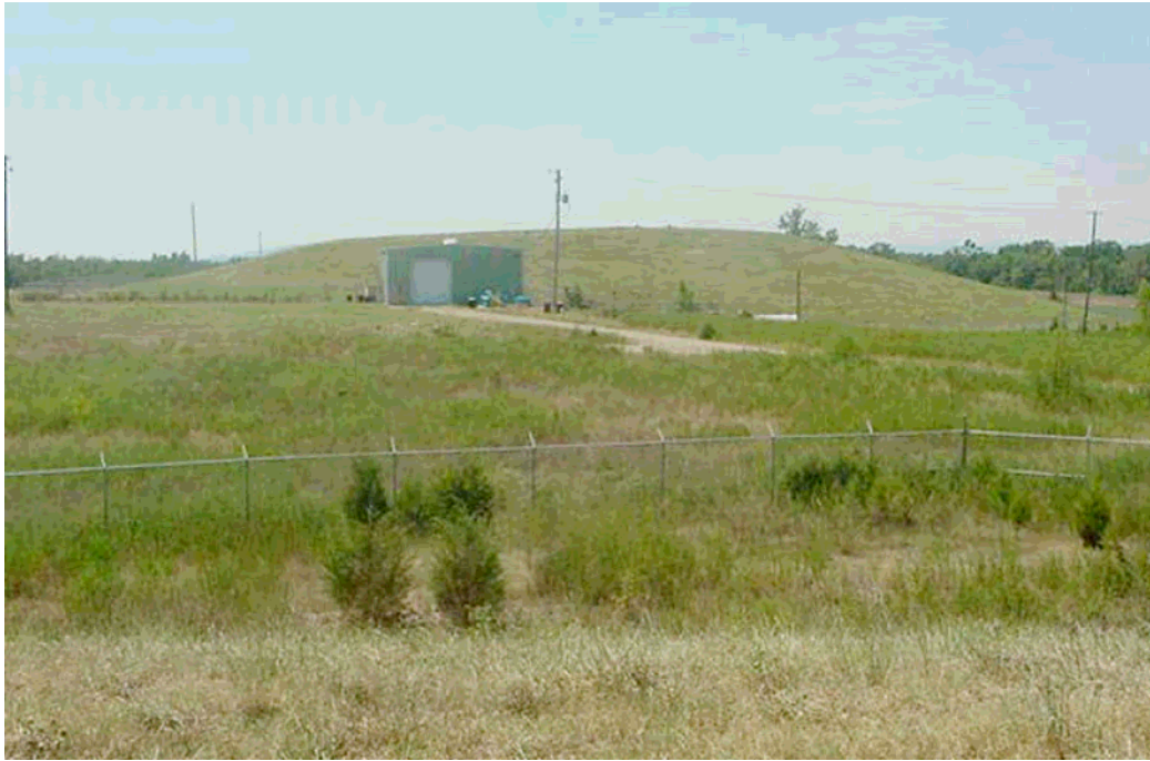
Photo 5: Standing on Old Pond capped area; note WWTP in distance and landfarm capped area; note perimeter security fence, which encircles Old Pond; fence also encircles Landfarm capped area
