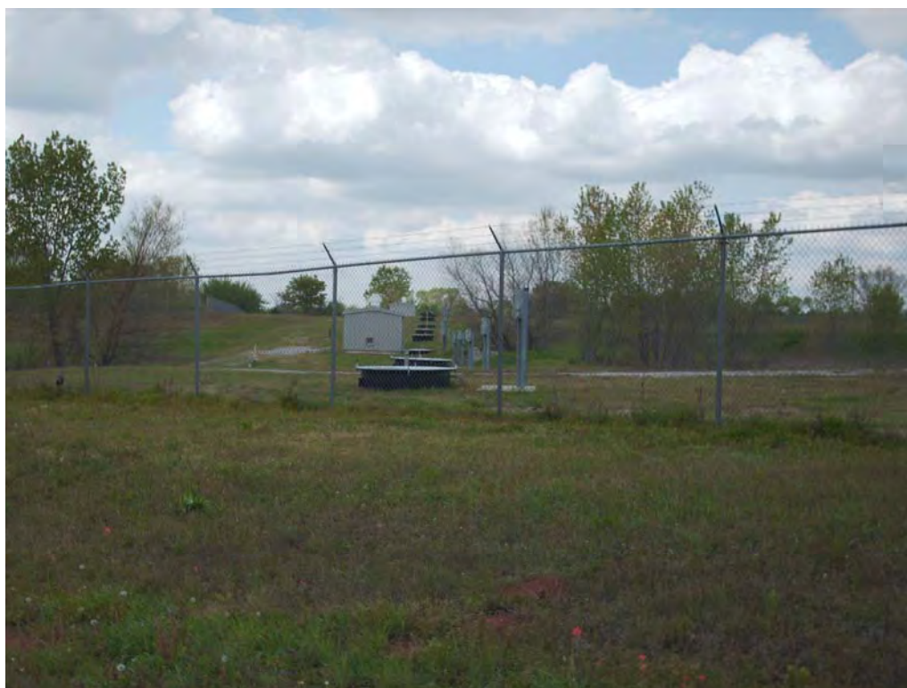
Photograph No. 19 Description: SWWRS
