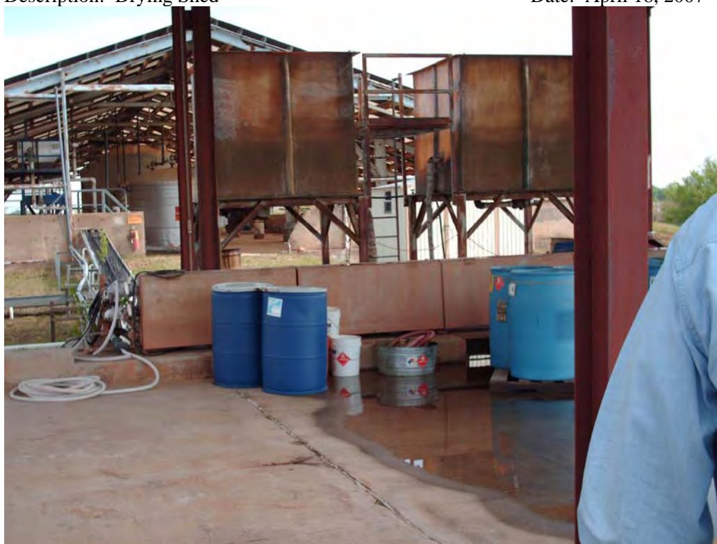
Photograph No. 12 Description: Storage at Drying Shed
