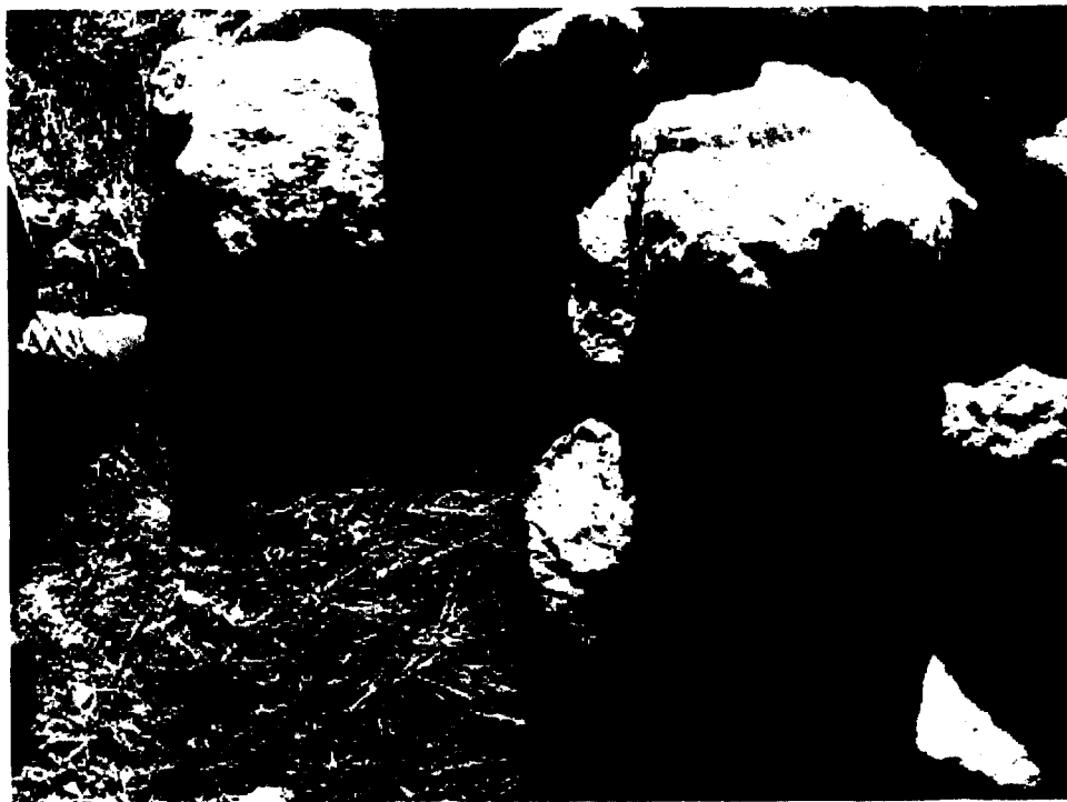
Close up of filter fabric not covered with rock.
