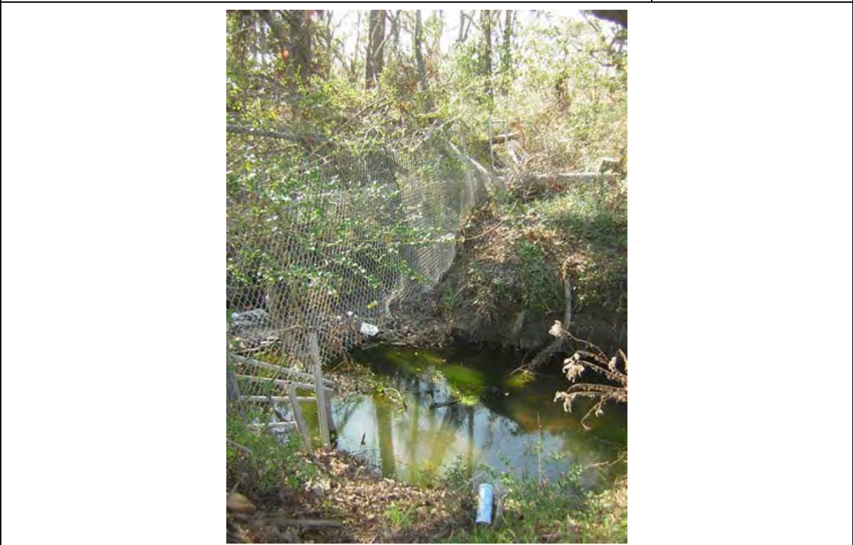
Photo 60: Damaged perimeter fence west of site entrance gate. Taken 2/16/2006
