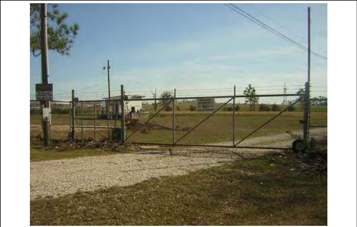
Photo 59: Front gate access to site. Taken 2/16/2006
