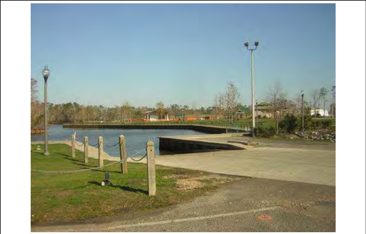
Photo 1: City park & boat ramp south of Bayou Bonfouca. The site landfill cover is visible in the background (past the structure in the photo center). Taken 2/16/2006.
