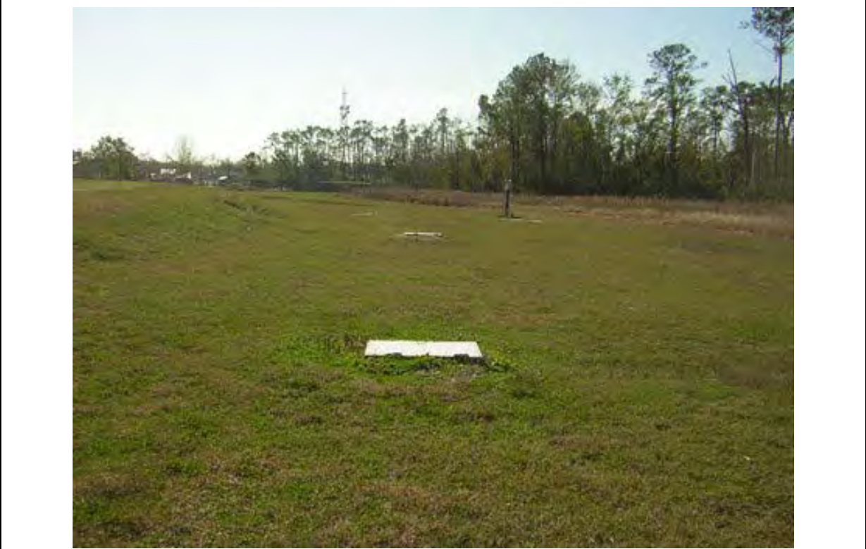
Photo 14: Looking south along recovery array 1A. Well vaults are flush-mount, and were inundated with water during Hurricane Katrina. Taken 2/16/2006
