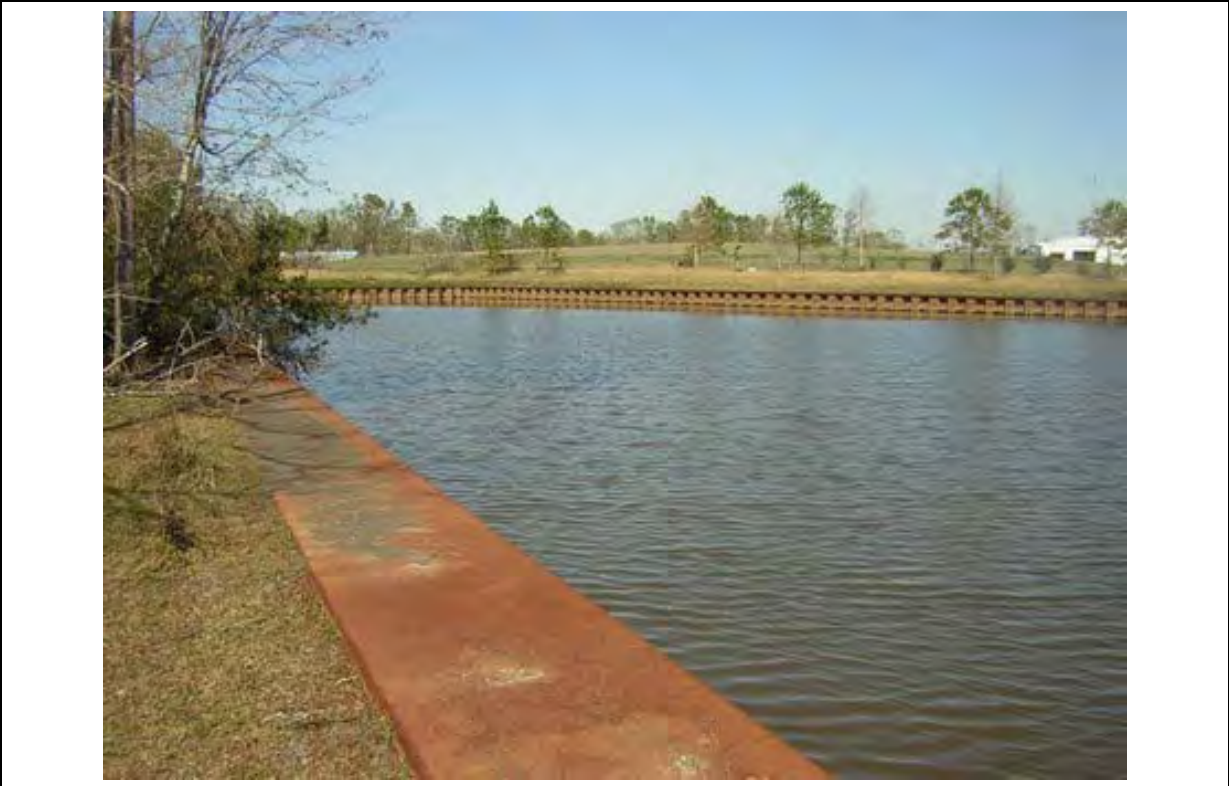
Photo 51: Looking north across Bayou Bonfouca toward onsite landfill. Ground water treatment plant is visible in far background left. Taken 2/16/2006
