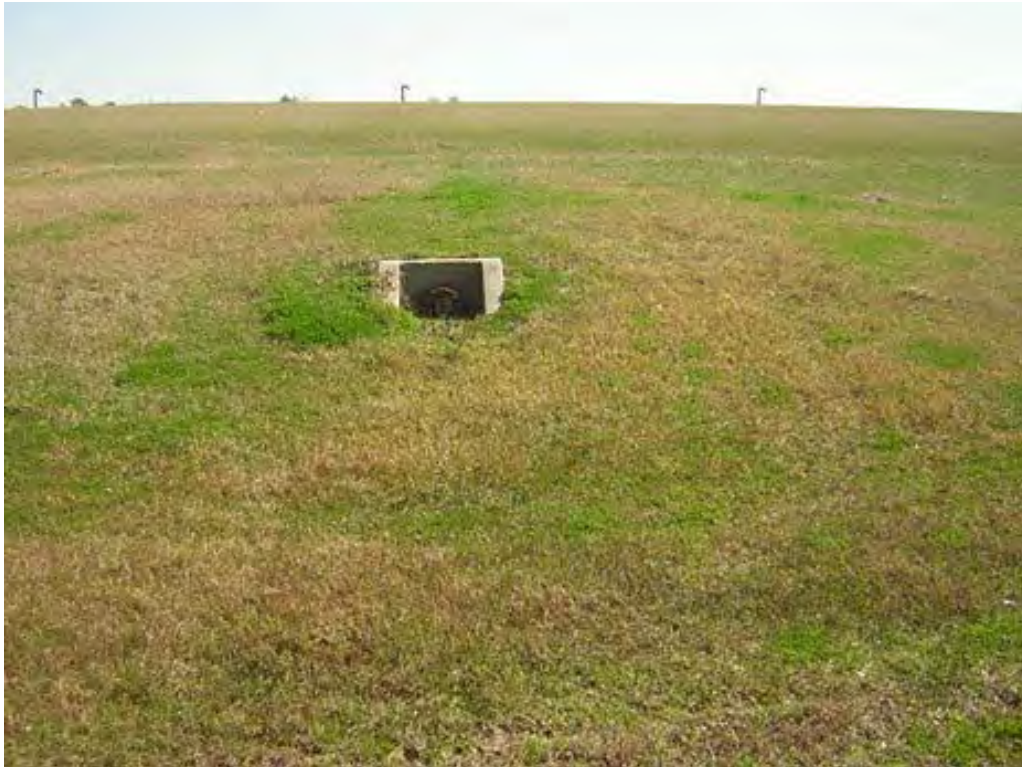
Photo 46: Surface drainage for landfill cover. Taken 2/16/2006
