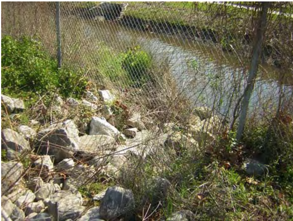
Photo 36: Surface drainage channel into East Drainage Channel on southeast side of site. Taken 2/16/2006
