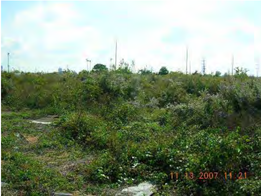
Photo 13: View looking southeast inside OU 1 showing overgrown vegetation on cap.
