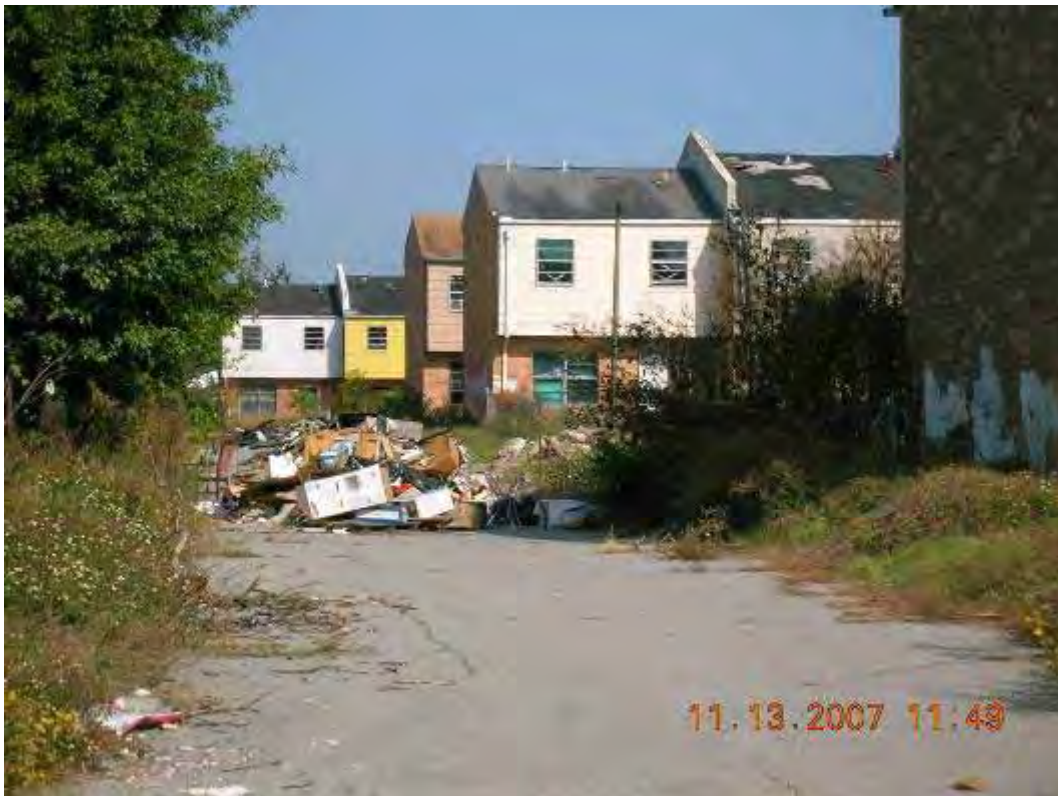
Photo 24: View looking north next to the HANO Housing Press Court Apartments. Mounds of debris are left in the drive.
