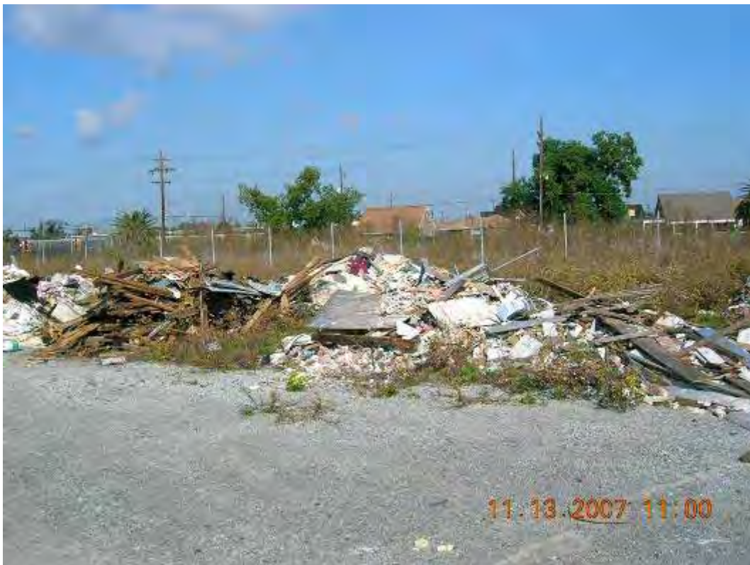
Photo 2: View looking northwest inside OU 1. Debris from reconstruction efforts were dumped at the former response action staging area.
