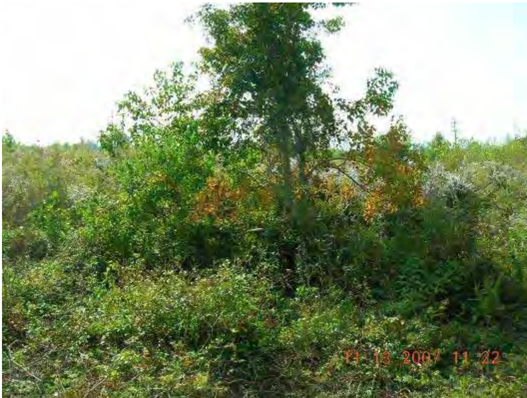
Photo 14: View inside OU 1 showing one of the several trees growing on the OU 1 cap.
