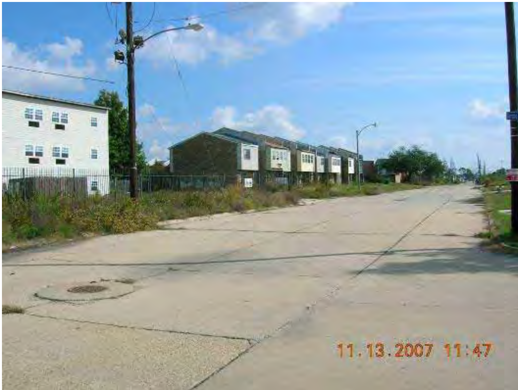
Photo 23: View looking east along Benefit St. Gordon Plaza Apartments on the left of the photograph and HANO Housing Press Court Apartments at center of photograph.
