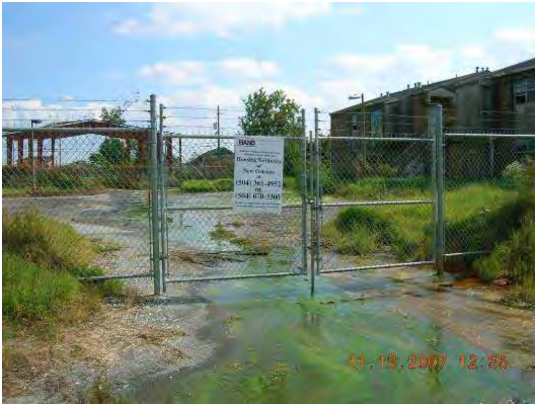
Photo 35: View looking east at one of HANOs Housing complex. A water leak was spotted at this location apparently coming from one of the apartments.
