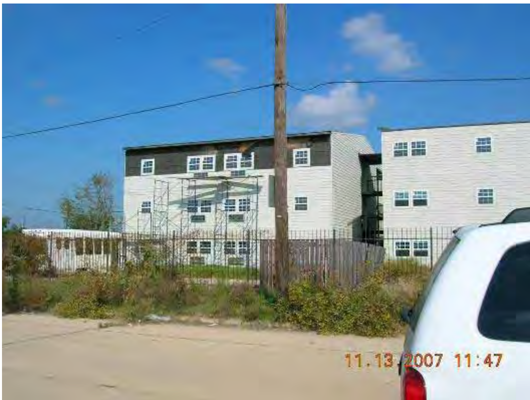
Photo 20: View looking north at Gordon Plaza Apartments.
