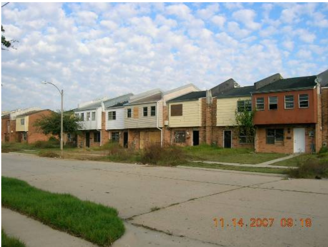
Photo 46: View looking northwest towards abandoned apartment complex along Abundance Street.
