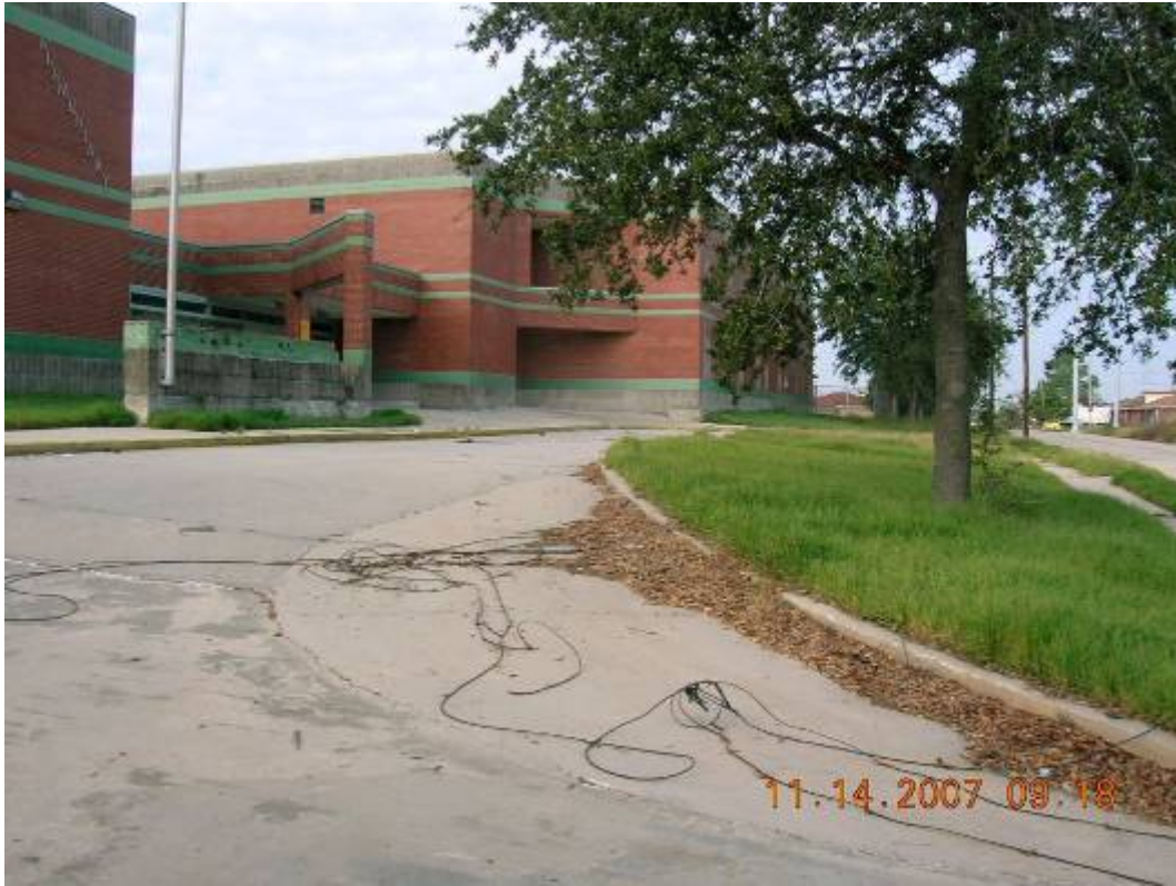
Photo 45: View looking west at the front of Moton Elementary School.
