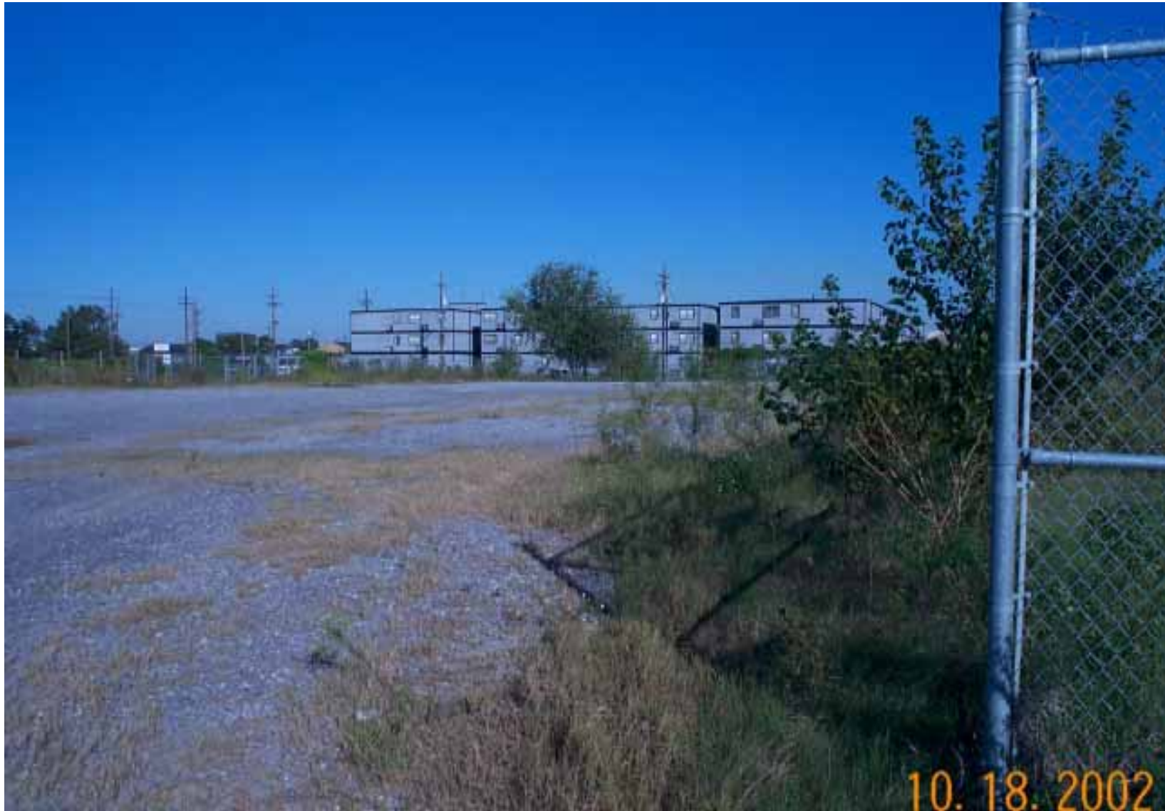
Photo 41: On north end of OU1, looking east towards staging area for response activities.
