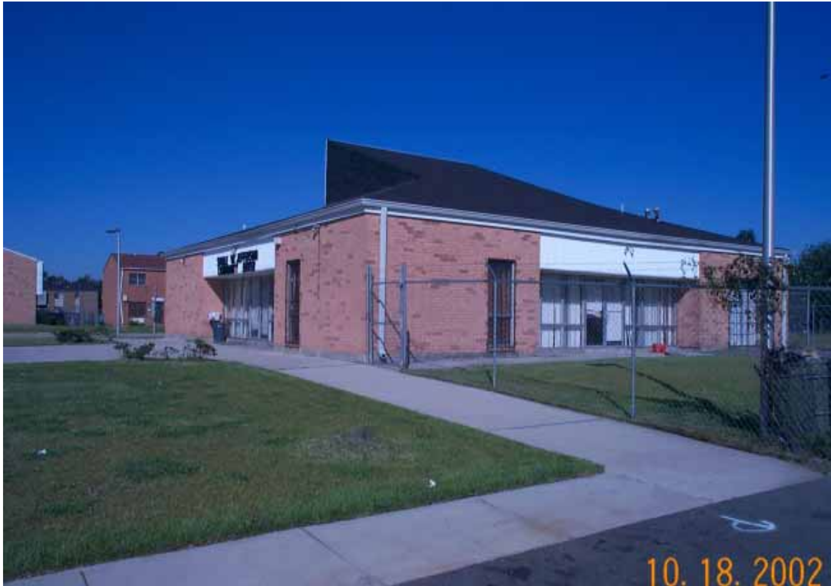
Photo 15: Looking northeast towards the Shirley Jefferson Community Center (OU3).
