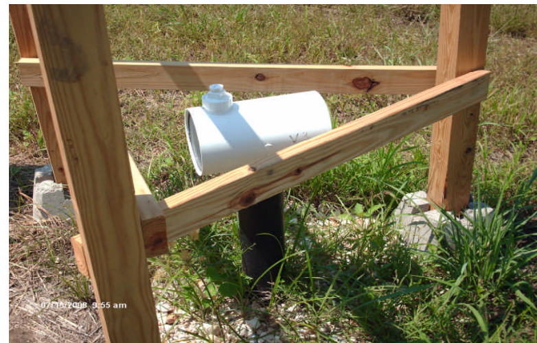
Photograph 8 Site: Cleve Reber Superfund Site Description: Close-up of gas vent system point V-3 (facing west). Date: July 15, 2008
