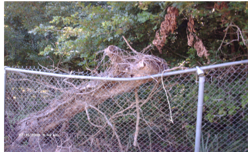
Photograph 4 Site: Cleve Reber Superfund Site Description: Fence damage due to fallen tree, located east of monitoring well P-10 (facing south). Date: July 15, 2008
