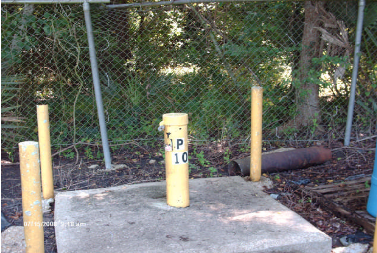
Photograph 5 Site: Cleve Reber Superfund Site Description: Monitoring well P-10 (facing south). Date: July 15, 2008
