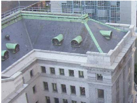
Example of a building that has attic space.
