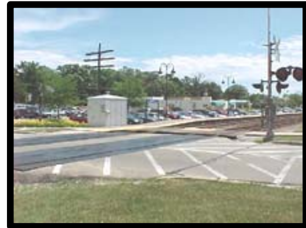
Figure 6. Southwest corner facing northeast.
