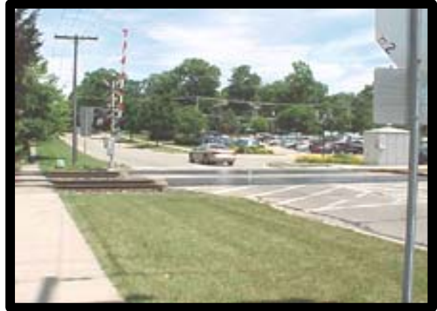
Figure 2. Southwest corner facing north.
