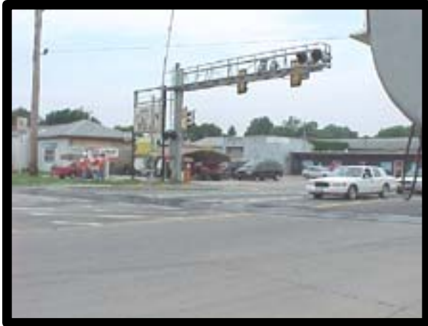
Figure 1. Southeast corner facing northwest.
