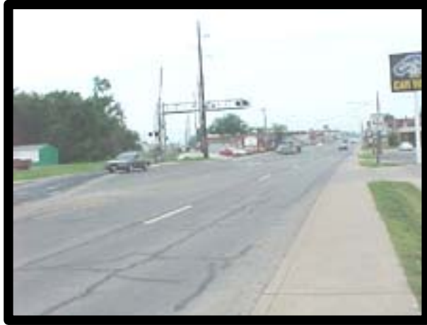
Figure 1. Northeast corner facing west.
