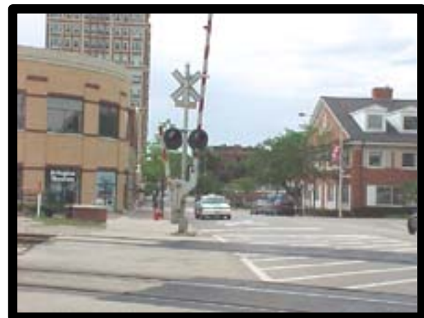
Figure 6. Northeast corner facing south.
