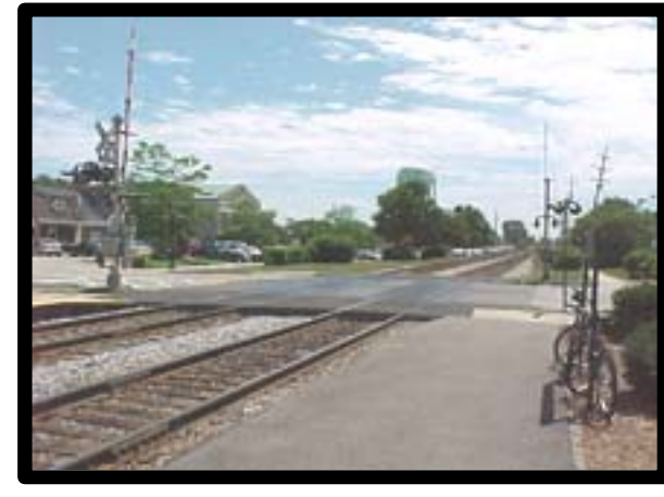
Figure 6. Southwest corner facing east.
