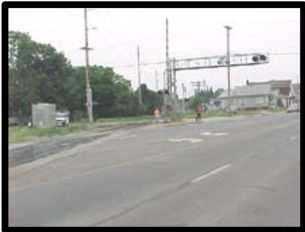
Figure 3. Southeast corner facing northeast.
