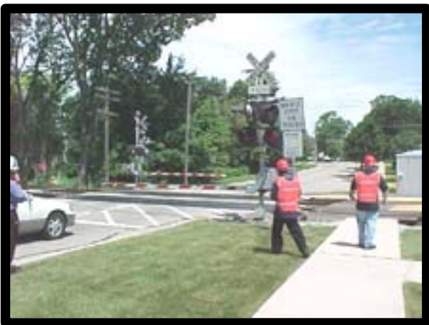
Figure 5. Southeast corner facing north.
