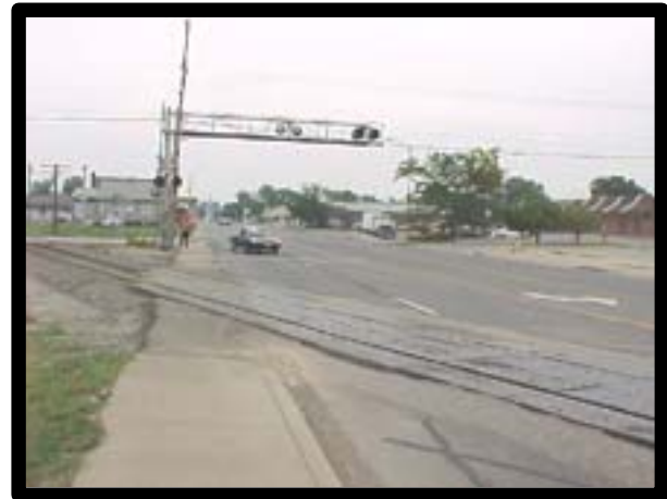
Figure 4. Northwest corner facing east.
