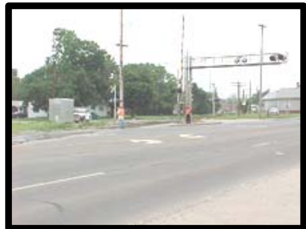
Figure 6. Southeast corner facing northeast.
