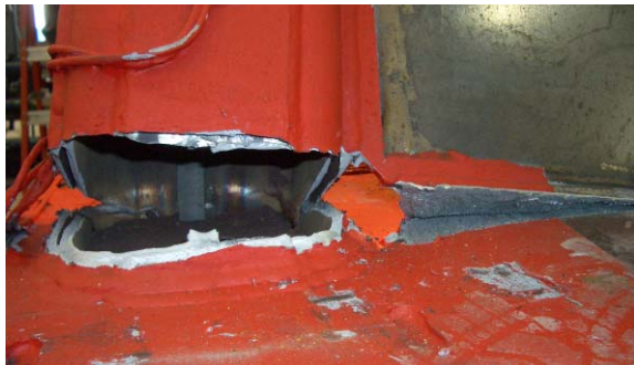
Figure 16. Quasi-static corner post post-test detail photos.
