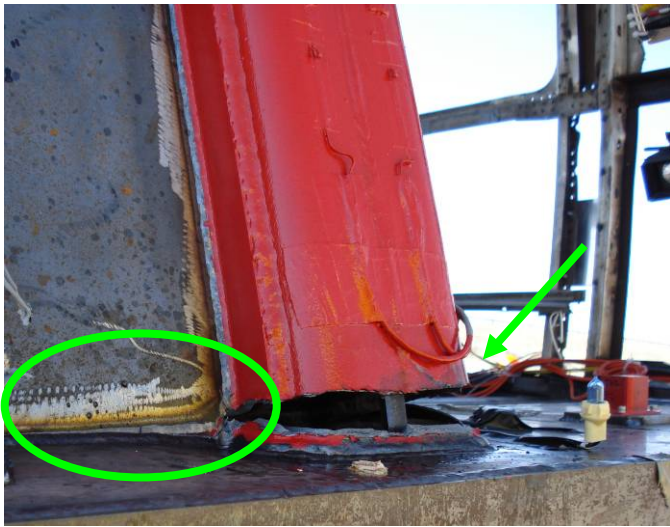
Figure 8. Fracture at the connection between the collision post and the buffer beam.
