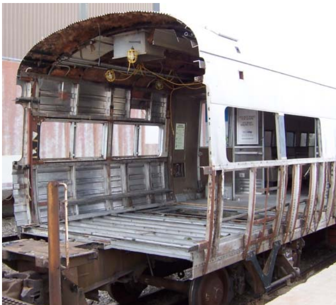
Figure 2. The cut M1 car ready for retrofit
