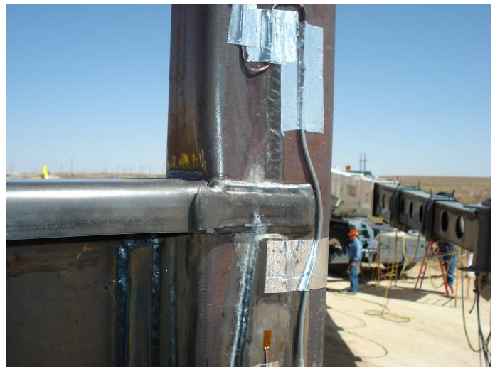
Figure 16. The connection of the shelf to the corner post, post-test
