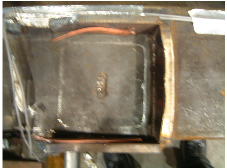
Figure 29. Bulging in the Primary Energy Absorber Attachment Plates
