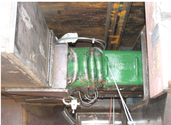
Figure 9. Primary Energy Absorbers, Post-Test
