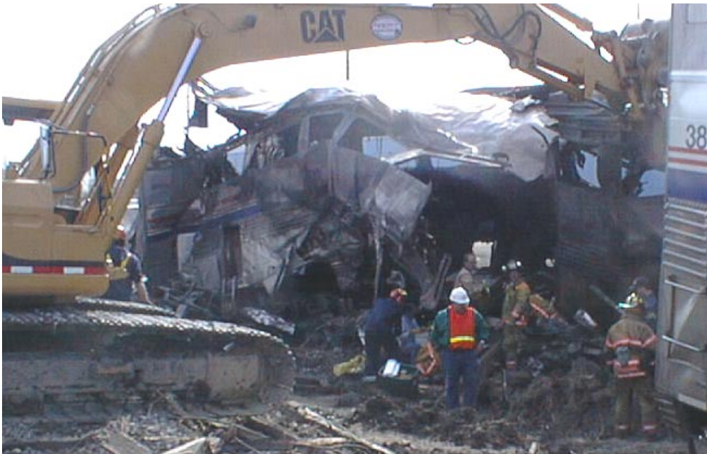
Figure 10. Post-accident photograph, second bi-level passenger car, Bourbonnais, Illinois collision.
