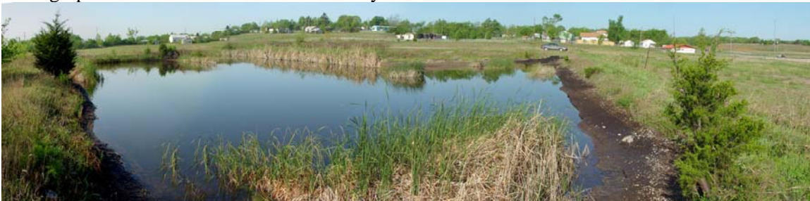
Photograph 5 – Coke Pond on South Refinery
