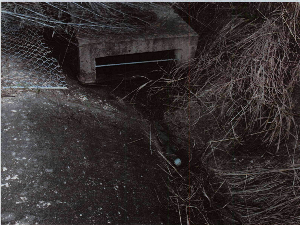
Picture 4: North collection drain on DOP North
