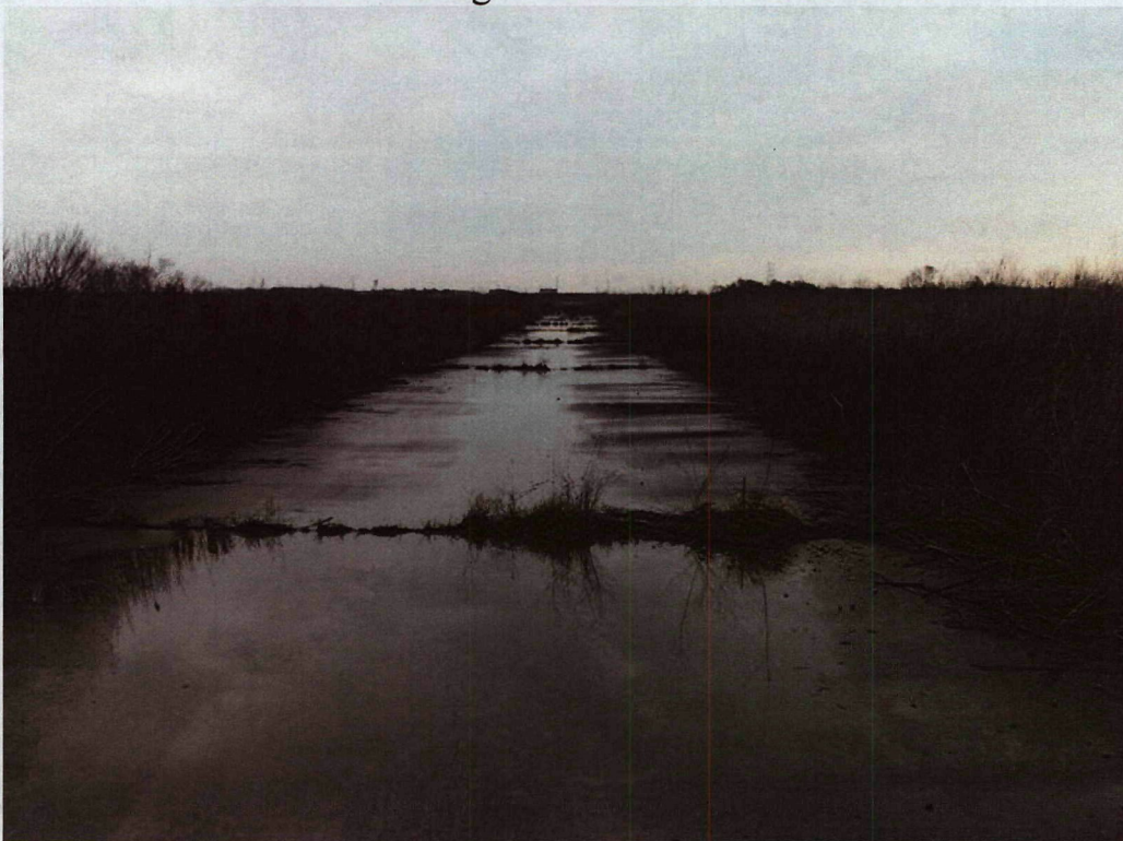
Picture 2: Center drainage swale on DOP North
