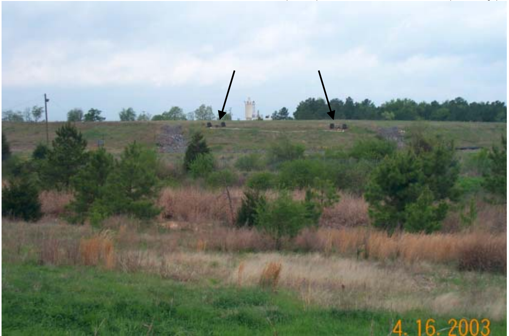
Photo 14: View of the OU1 landfill. View is facing west. The leachate collection and detection system sumps are visible near the top of the landfill (arrows).
