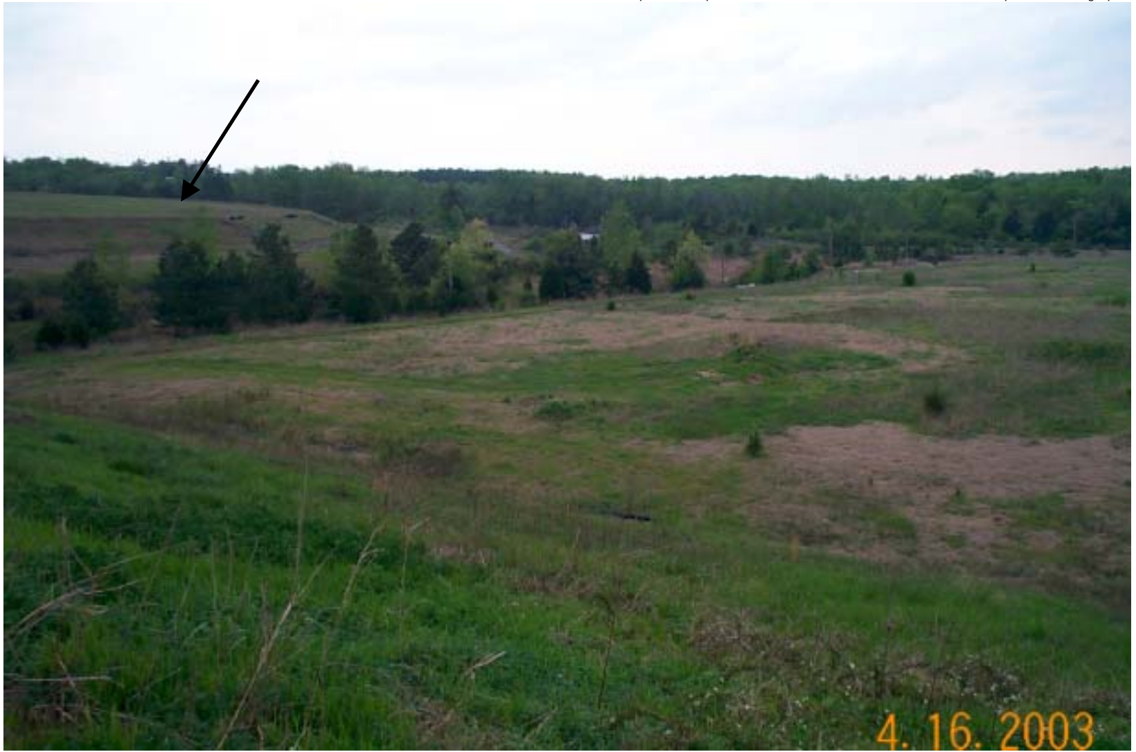
Photo 8: View across the North Burial Area from Sedimentation Vault (Mt. Vertac), facing northwest. Note trees growing on top of cap. The OU1 landfill is visible in the background at left (arrow).
