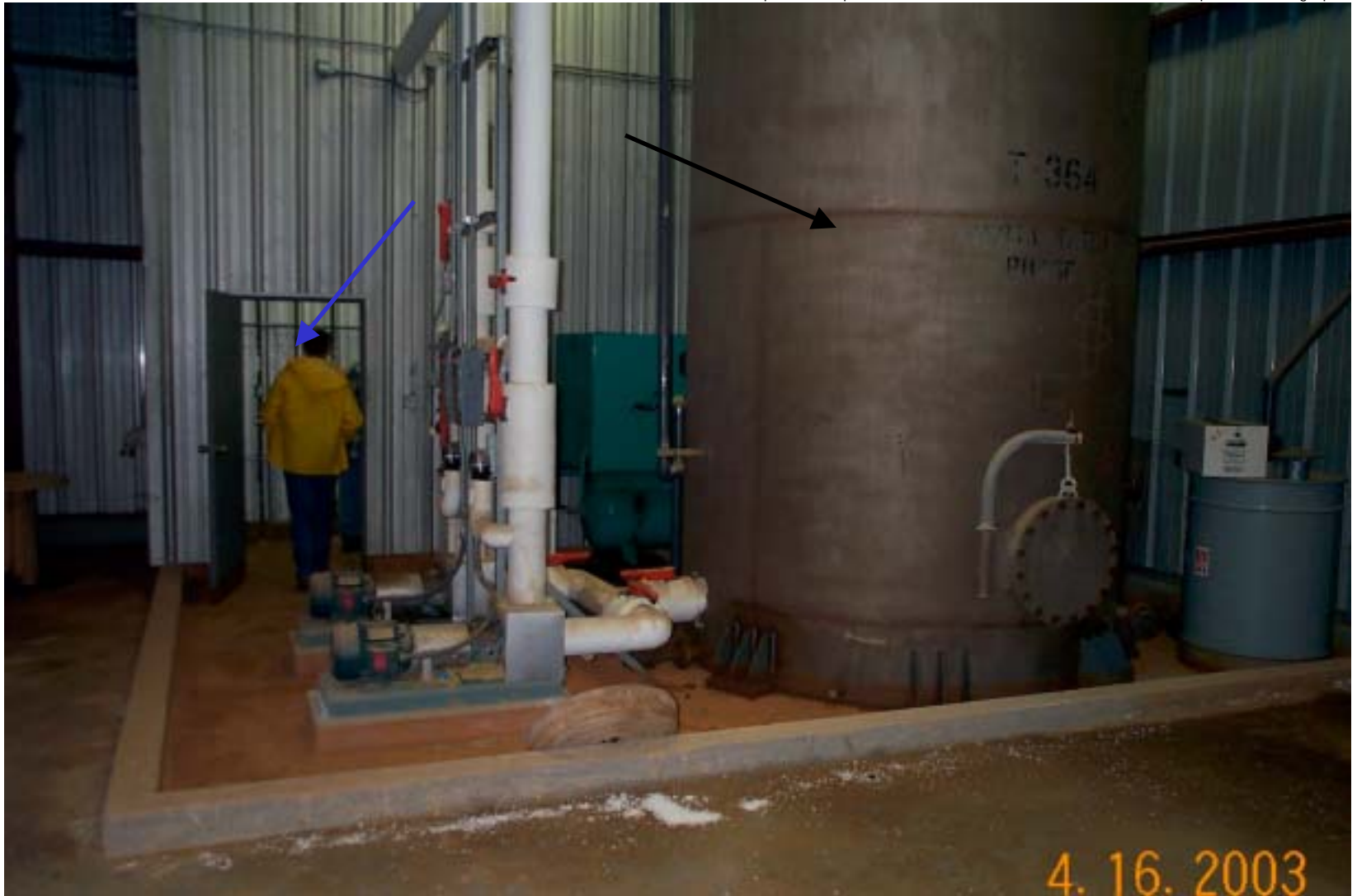
Photo 43: View inside the Groundwater Recovery Building. Tank to the right (black arrow) is used to store extracted ground water prior to transfer to the Wastewater Treatment Plant. The room at the back (blue arrow) contains valves for sampling monitor wells and extraction wells. Note dirt on the floor from leaking wall.
