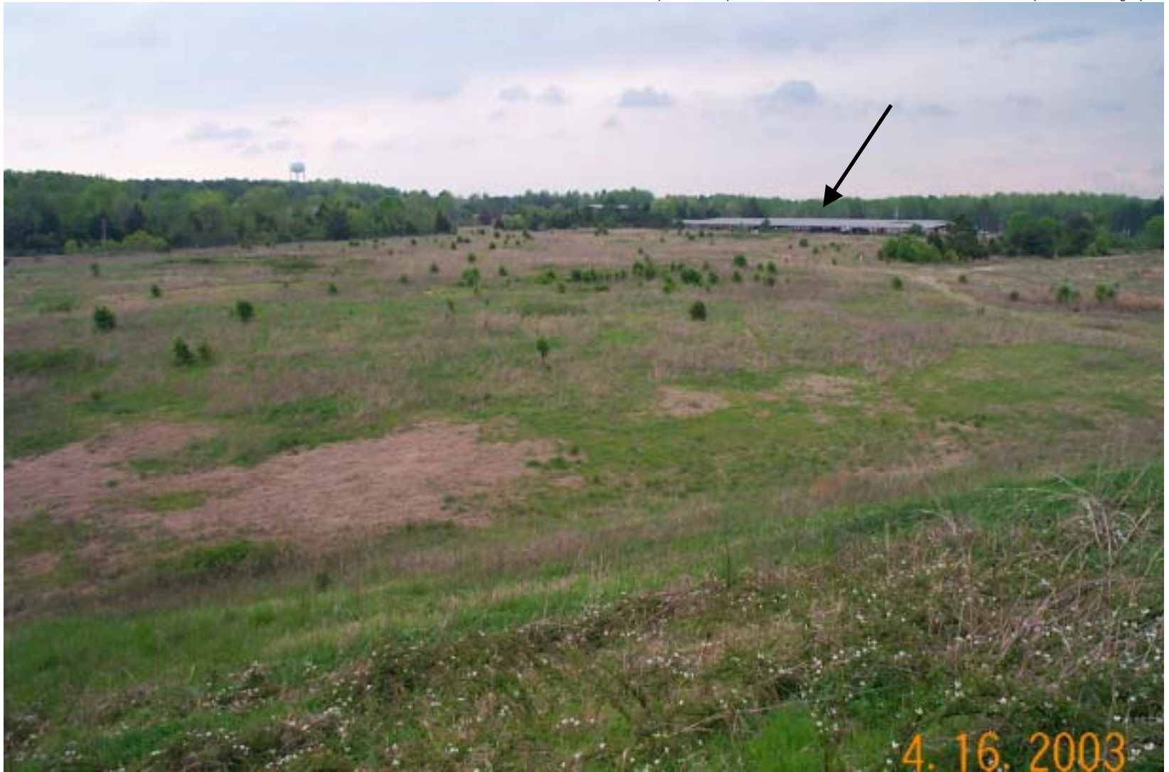
Photo 6: View across the North Burial Area from Sedimentation Vault (Mt. Vertac), facing north. Note trees growing on top of cap. Shed in background (at arrow) is a former storage shed used to store drums as part of the incineration (now used by City as part of recycling center).
