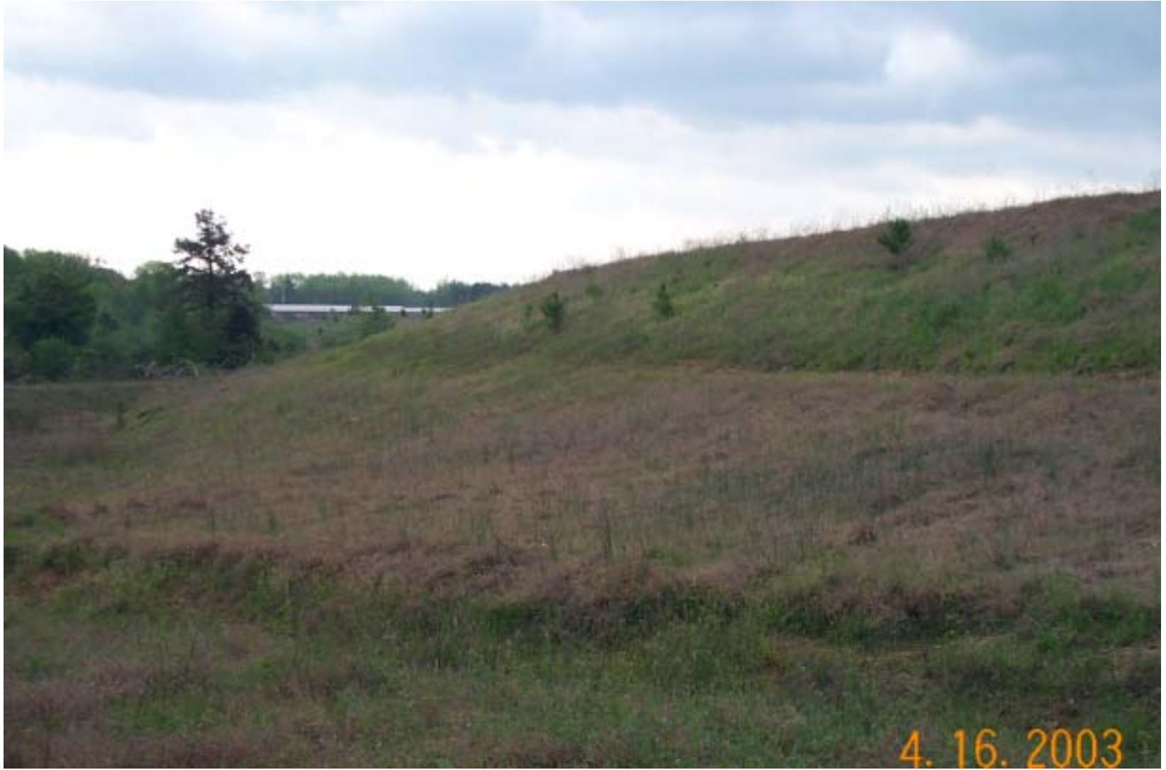
Photo 27: View of the north side of the OU1 landfill. View is facing east. Note small trees growing on the cap.
