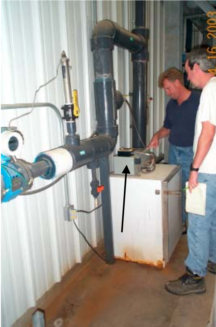
Photo 51: View of the automatic sampler unit (black arrow) inside the Wastewater Treatment Plant. This unit collects samples of the treated water prior to discharge.
