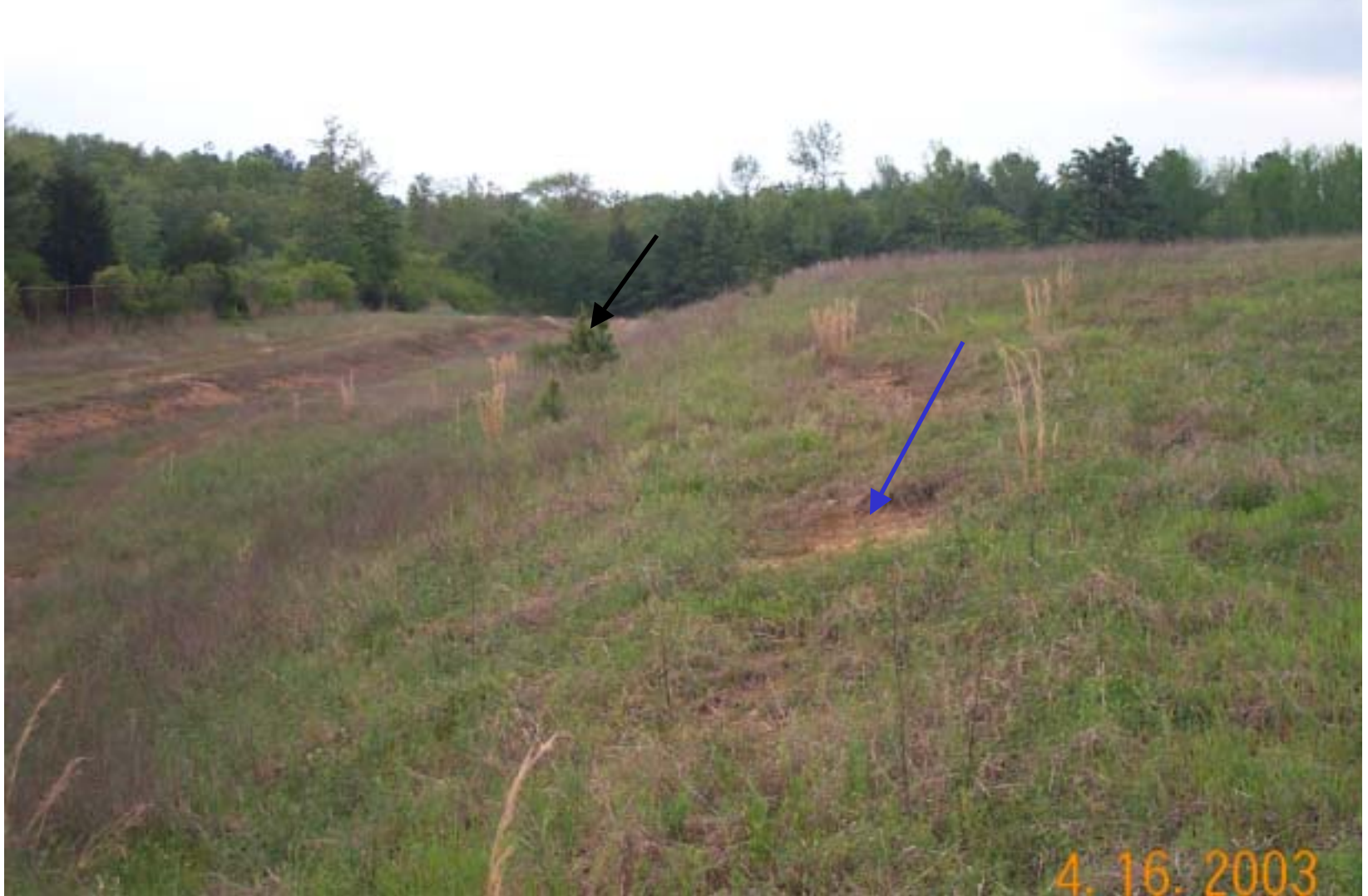
Photo 30: View of the west side of the OU1 landfill. View is facing north. Note small trees growing on the cap (black arrow) and area of sparse vegetation (blue arrow).
