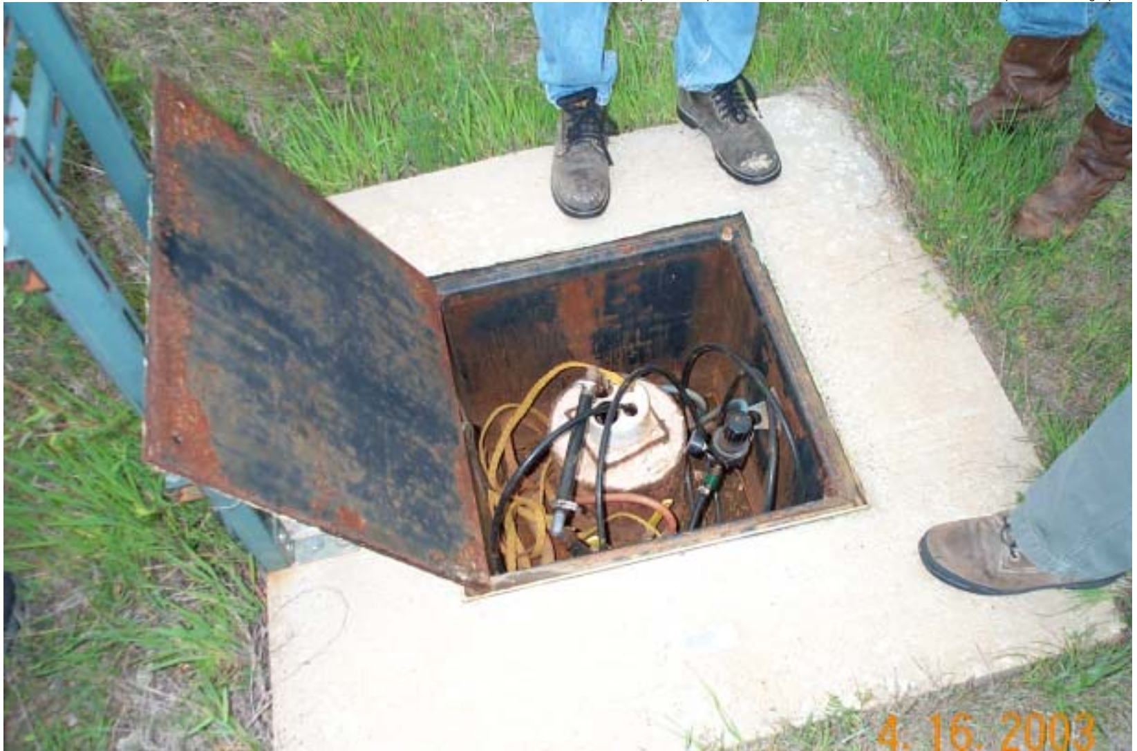
Photo 40: View of the inside of the well vault of a ground water extraction well.
