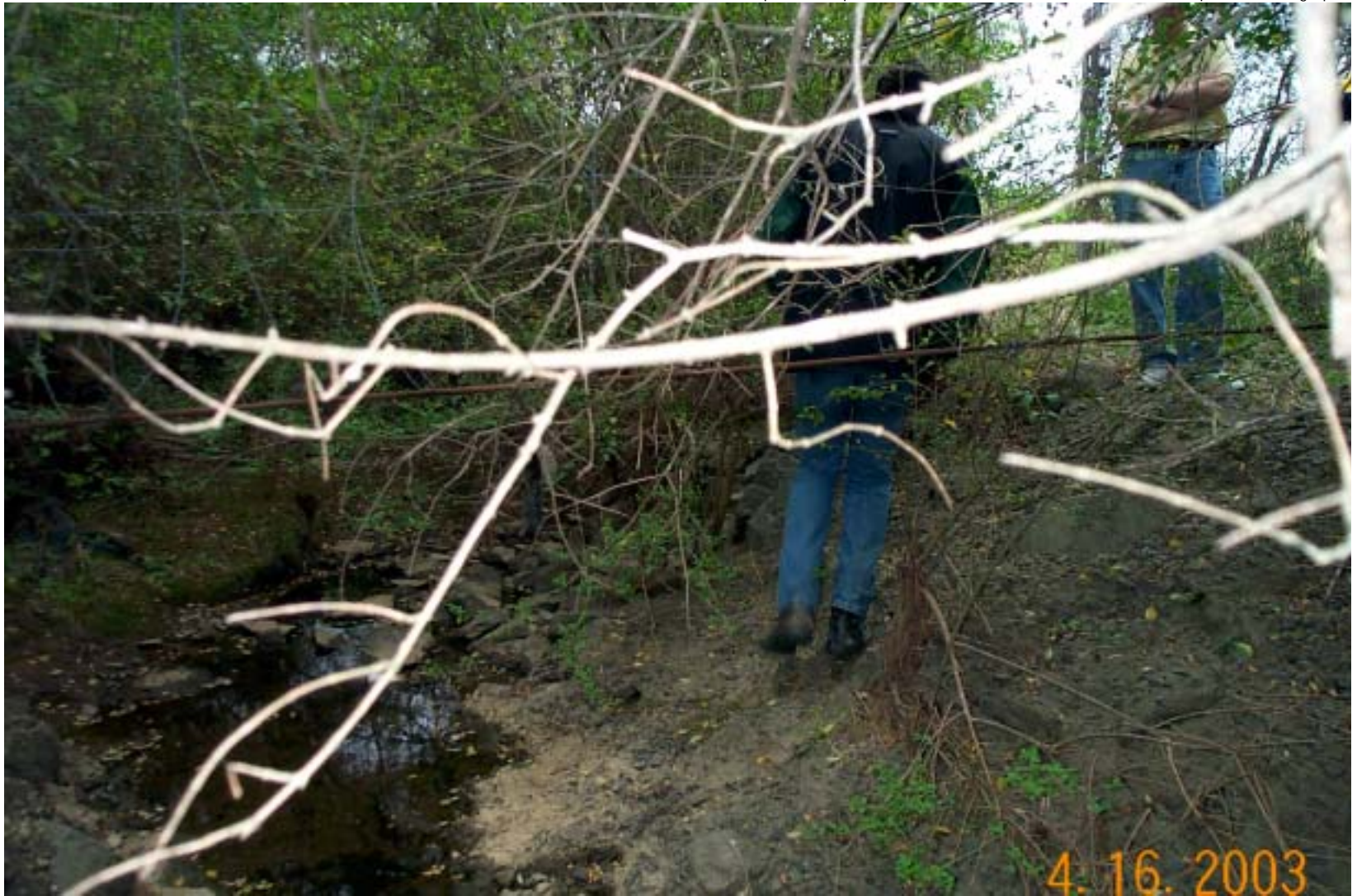
Photograph 34: View of Rocky Branch Creek near discharge pipe from the Wastewater Treatment Plant.
