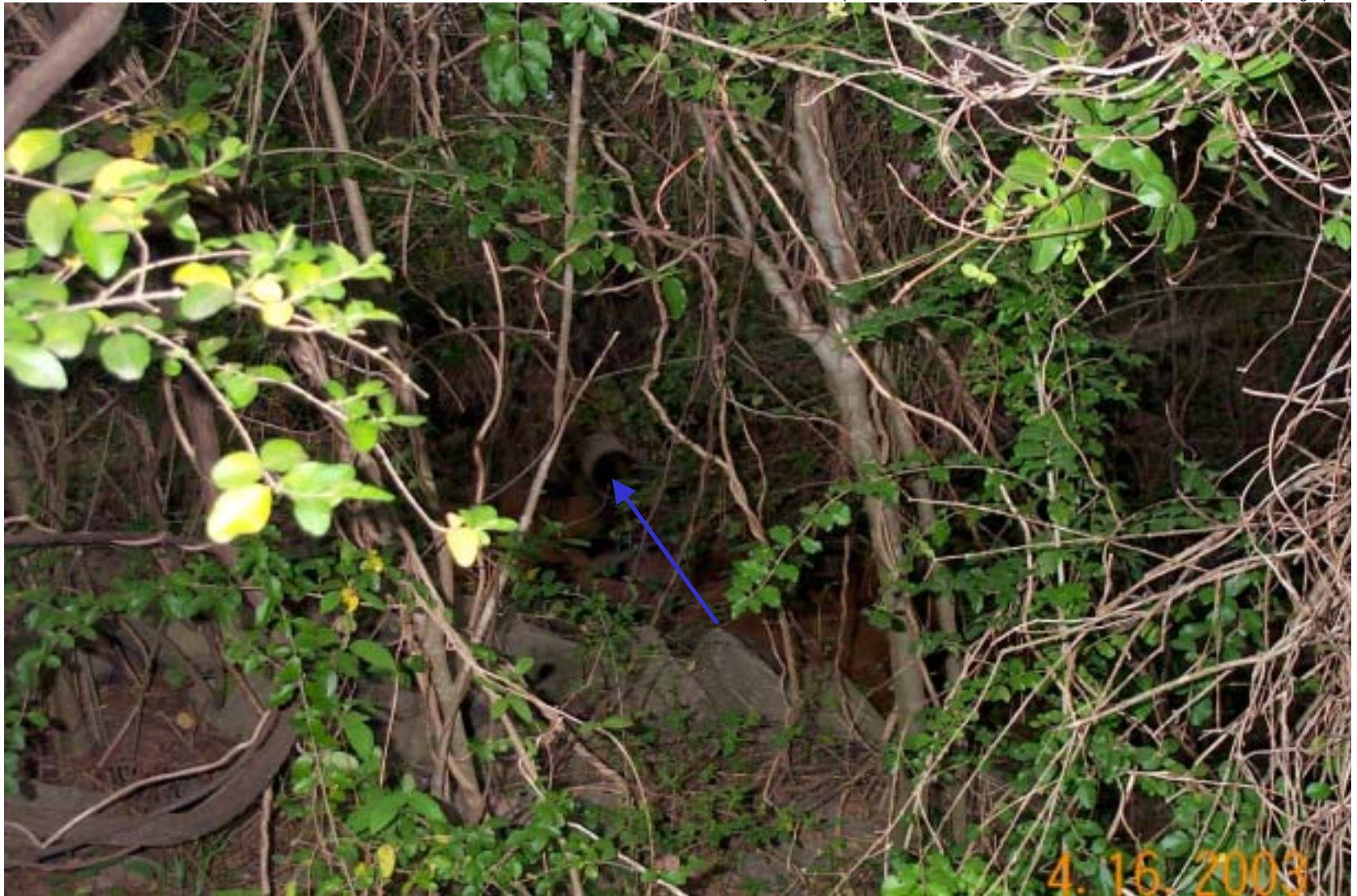
Photo 35: View of discharge pipe from the Wastewater Treatment Plant (blue arrow).
