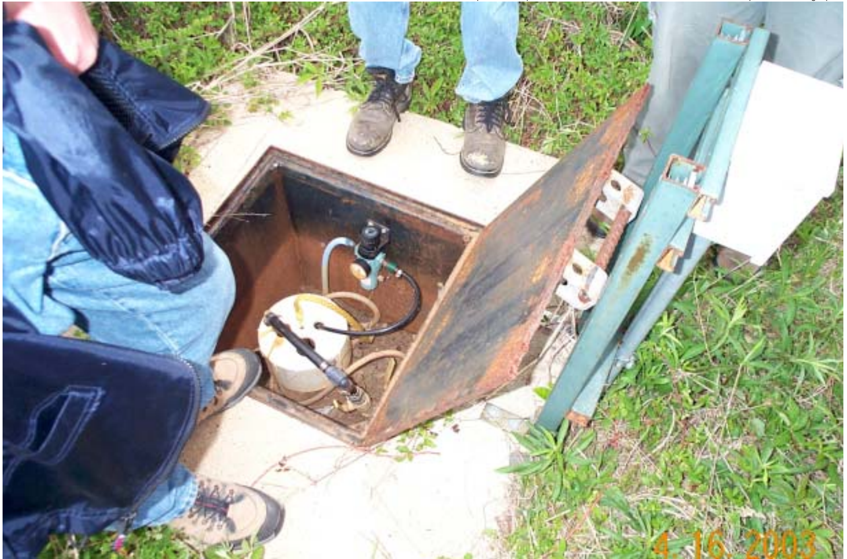
Photo 42: View of the inside of the well vault of a ground water extraction well.
