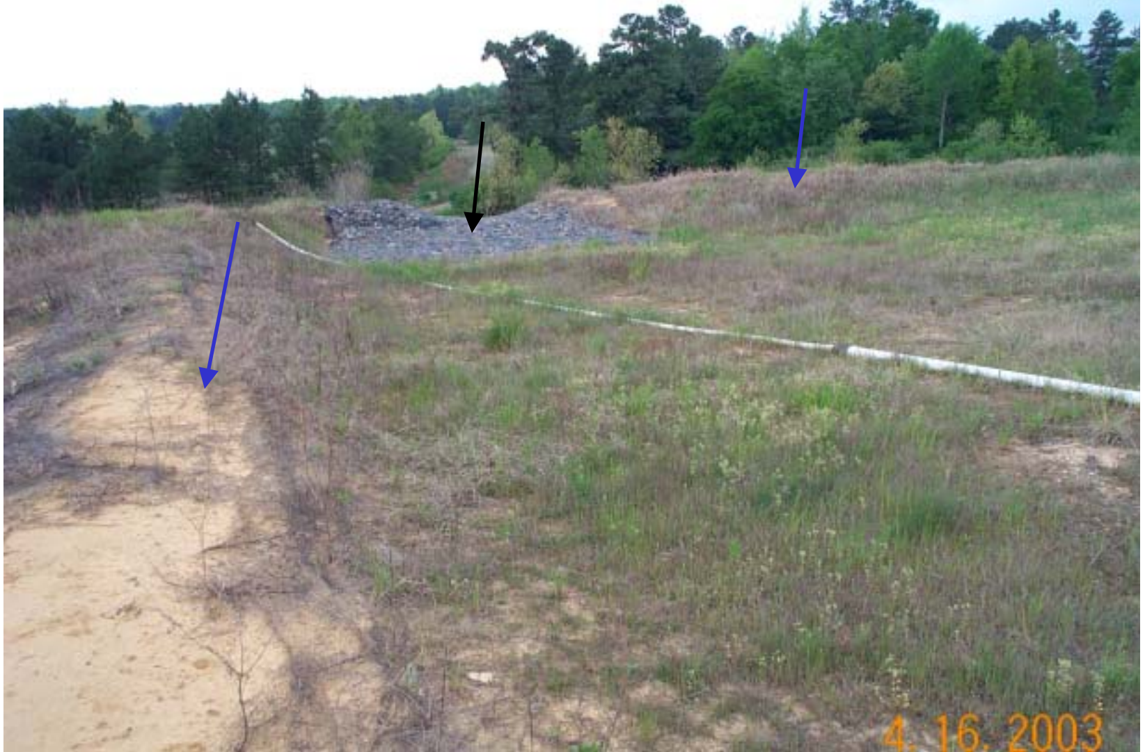
Photo 22: View of letdown channel (black arrow) from the top of the cap at the OU1 landfill. Berms (blue arrows) around outside edge of cap direct runoff to the letdown channels.
