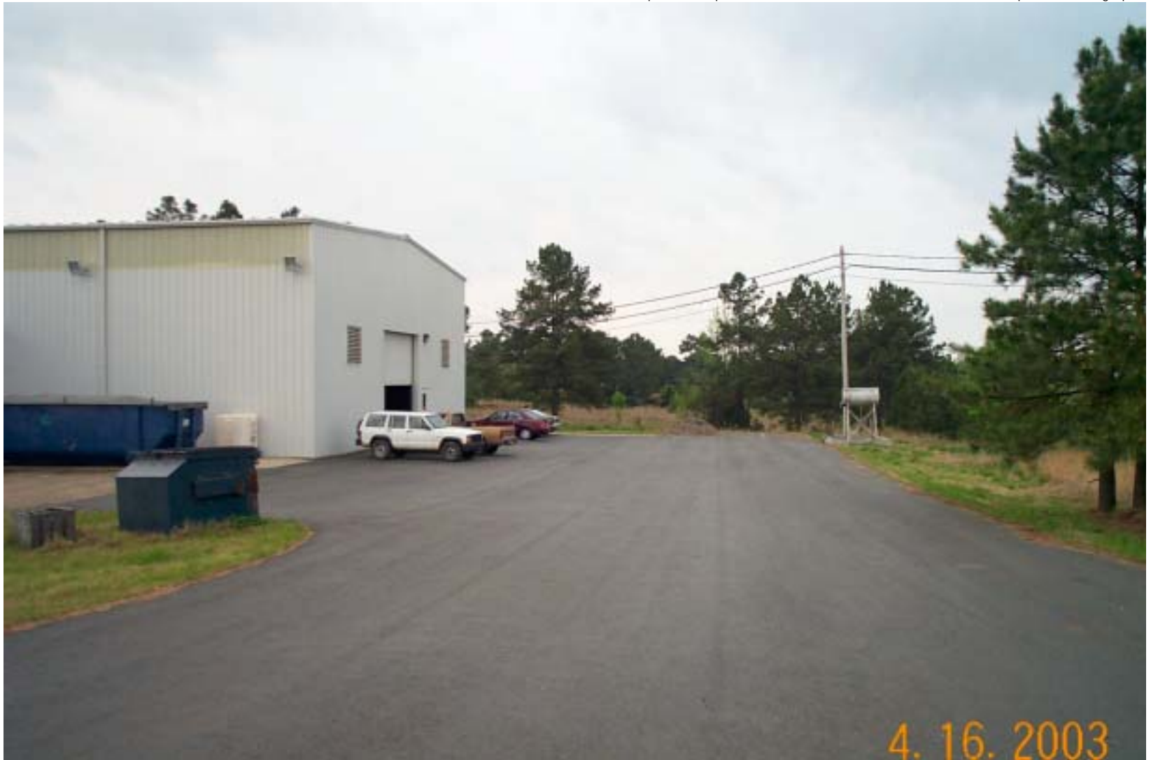
Photo 3: View to the south along the west side of the Wastewater Treatment Plant.
