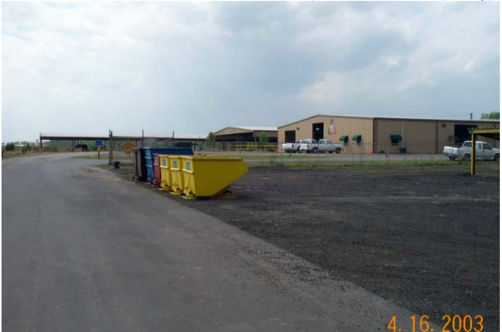
Photo 53: View of the City of Jacksonville's Sanitation Department and drive-through recycling center. These facilities are located in a shed on the northern portion of the site. View is to the west.
