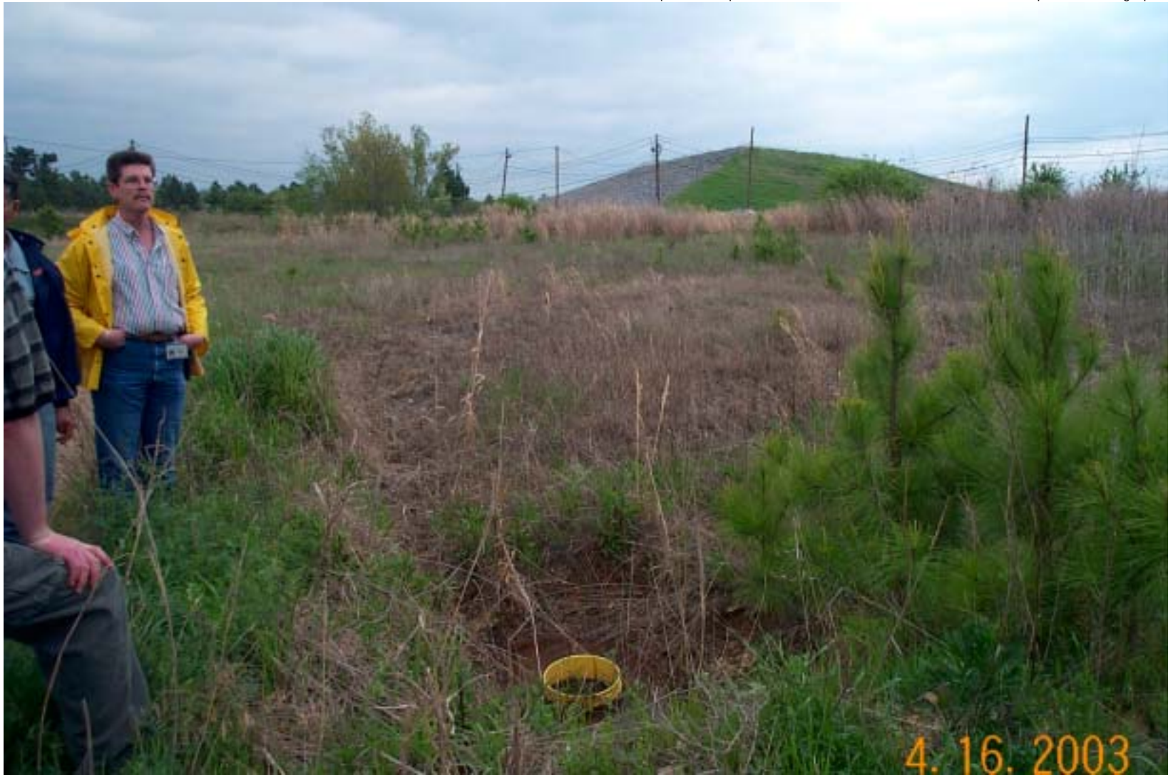
Photo 31: View facing north toward Mt. Vertac, across Reasor Hill Burial Area in center of photo. Yellow bucket is sump installed to collected observed surface seep.
