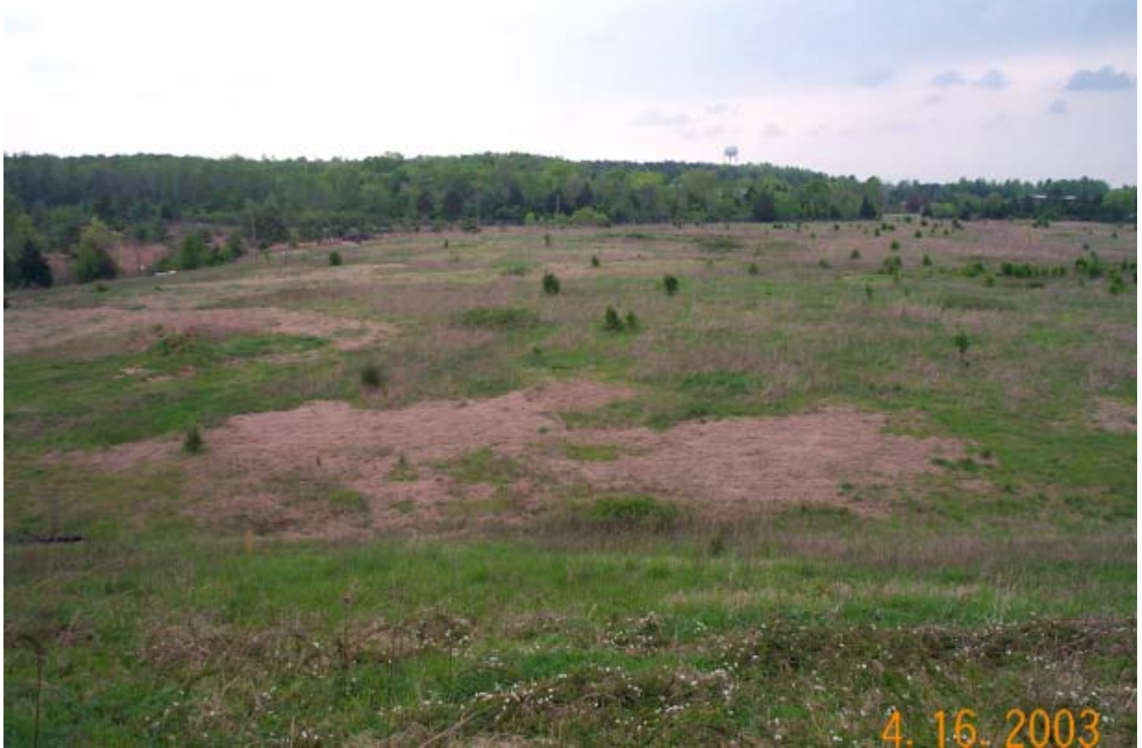
Photo 7: View across the North Burial Area from Sedimentation Vault (Mt. Vertac), facing north. Note trees growing on top of cap.
