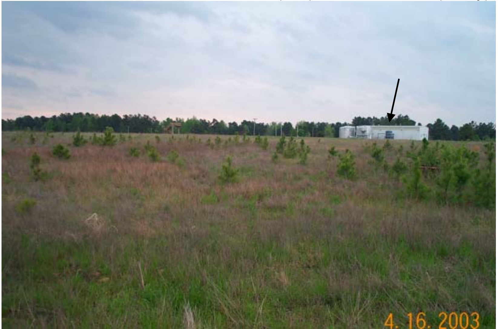
Photo 5: View of the former Central Process Area. View is to the south. The Wastewater Treatment Plant is in the background (Arrow).
