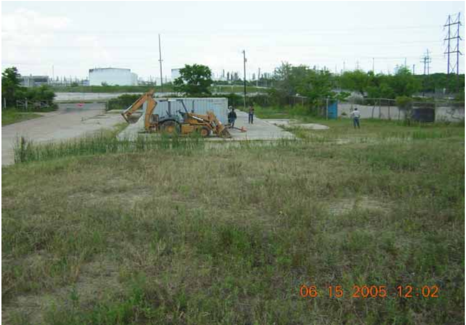
Photo 33: OU1: Equipment staging northwest of Pond 7 on former smelter concrete pads.
