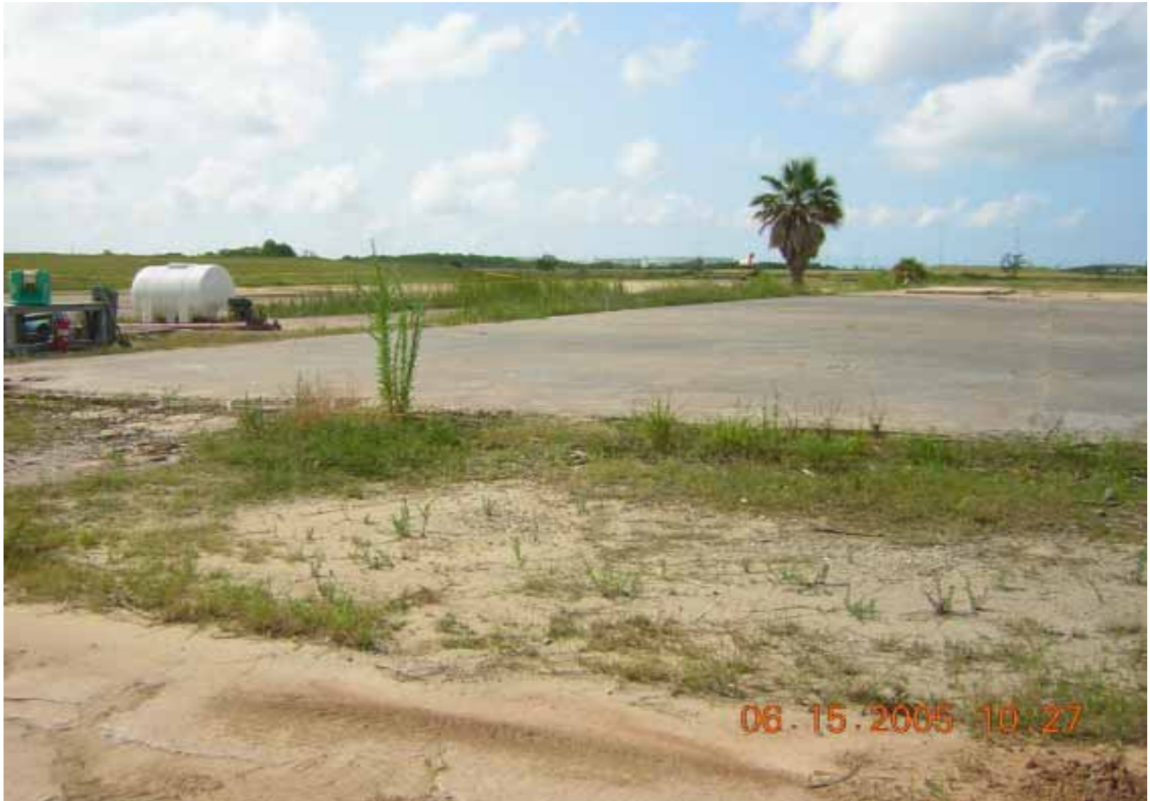
Photo 2: OU1: Concrete floor slab from former building.
