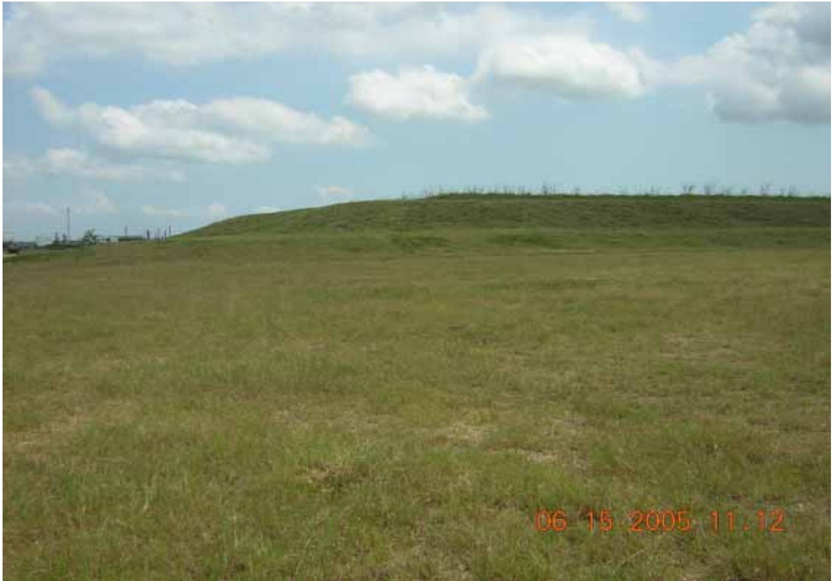
Photo 13: OU1: NORM disposal cell.
