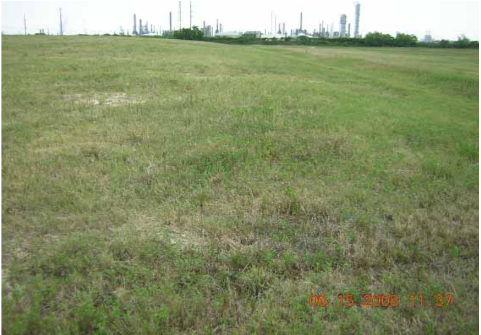
Photo 26: OU1: Facing north from the top of the Consolidation Cell.
