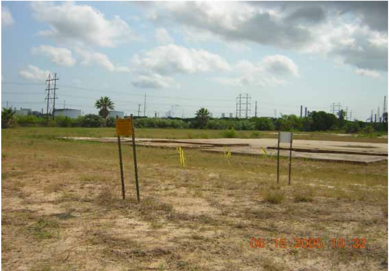
Photo 3: OU1: Concrete floor slab from former building. Signs mark the location of the slurry wall.
