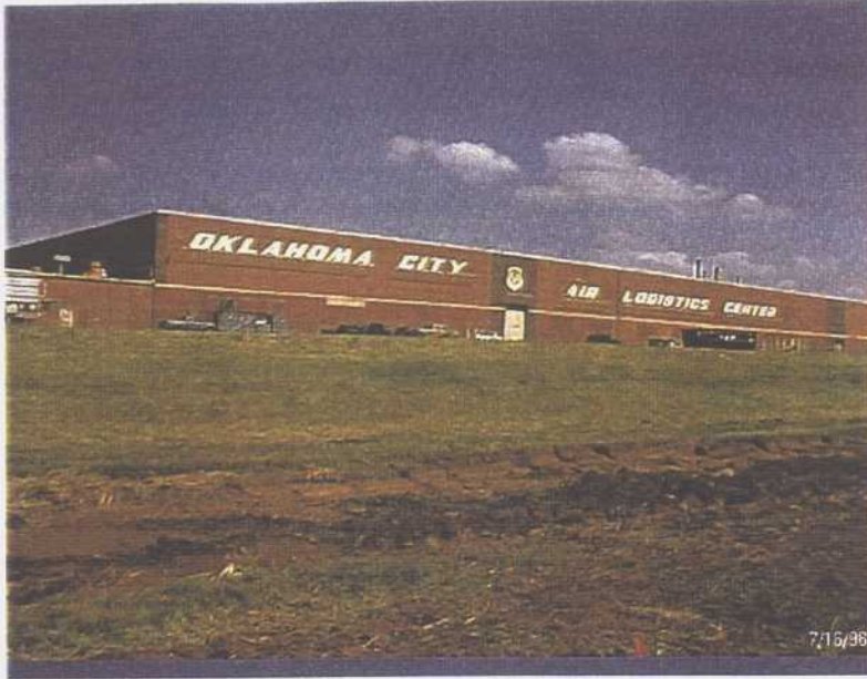
1. North end of Building 3001. Soldier Creek in foreground.
