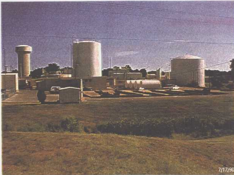
2. Industrial wastewater treatment plant overlying Operable Unit 4.
