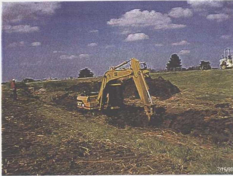
5. Excavation at West Soldier Creek, prior to concrete pouring.
