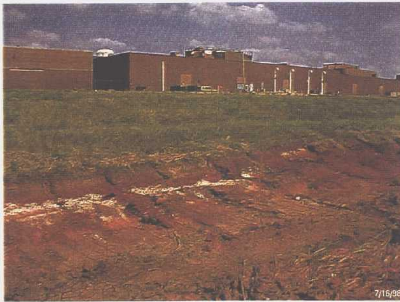
6. Preparation for concrete channel along West Soldier Creek.
