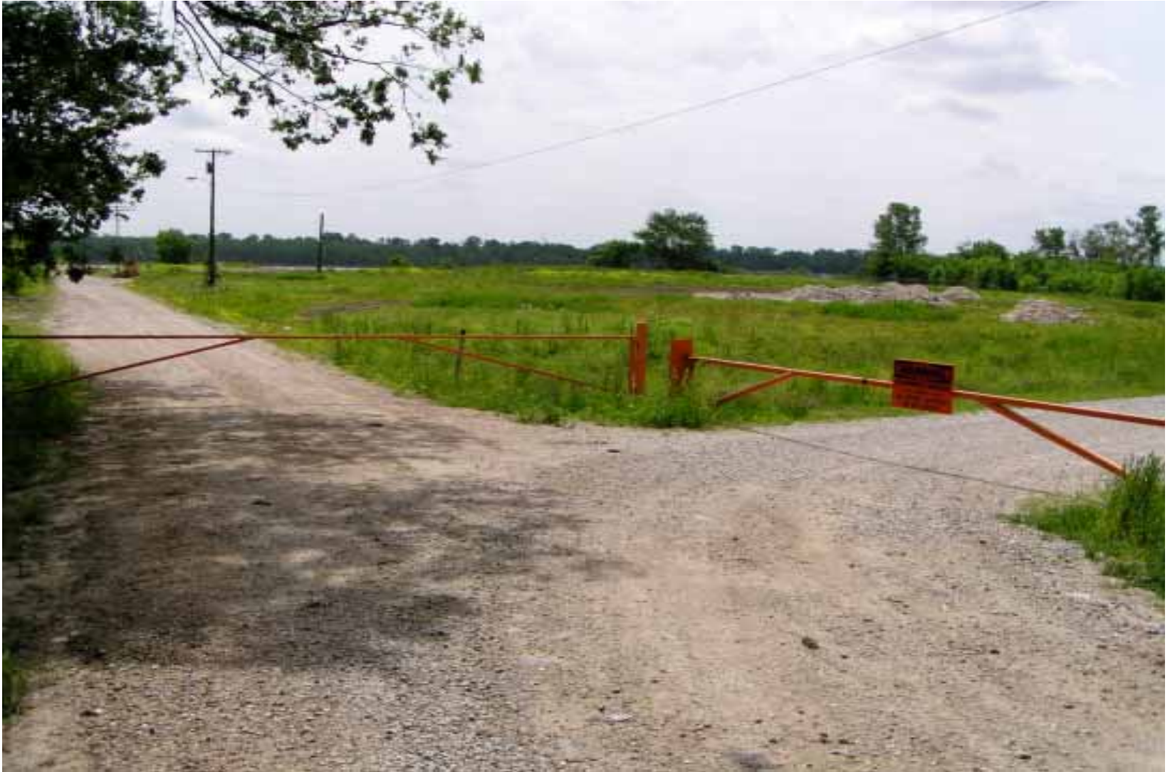
View of the two security gates at the main entrance to the site. The road and gate on the right is in Area 1 of the Site and leads to the southern barge terminal operation. The road and gate on the left separates Area 1 from the the oily sludge mound in Area 2. April 2004
