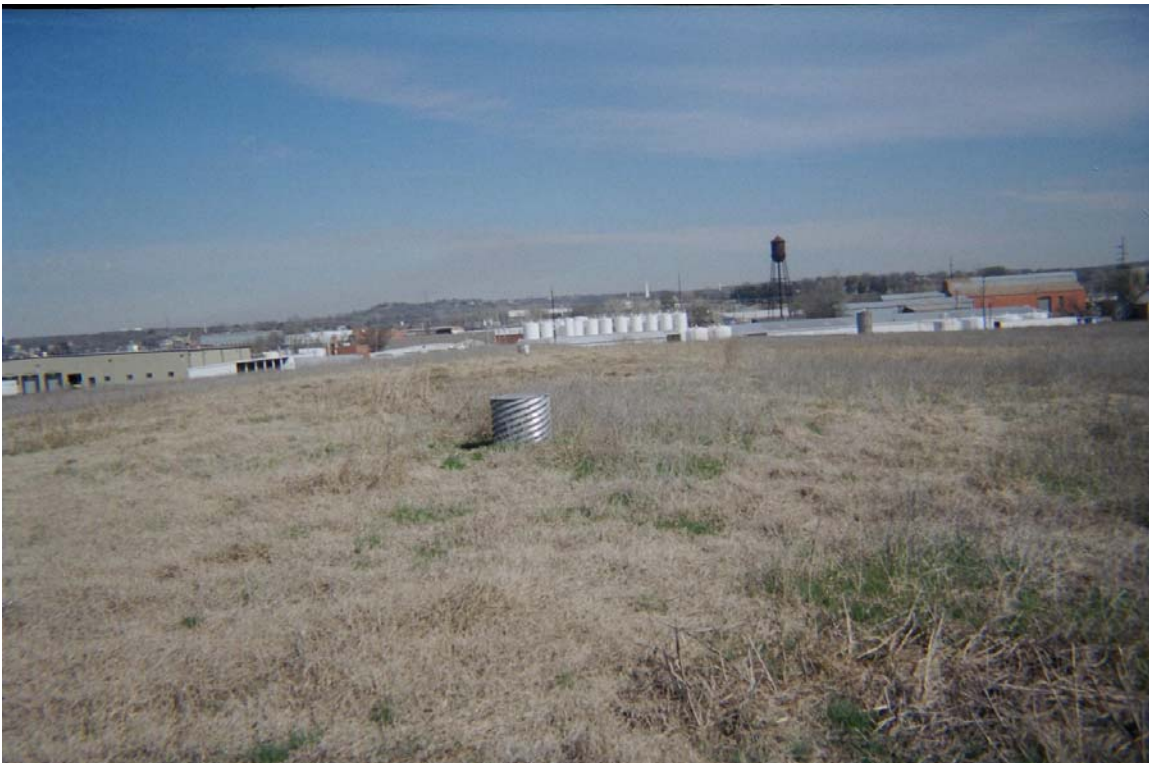
Photograph No. 6 Orientation: Northwest Description: Top of landfill cap, corrugated vent pipe in center
