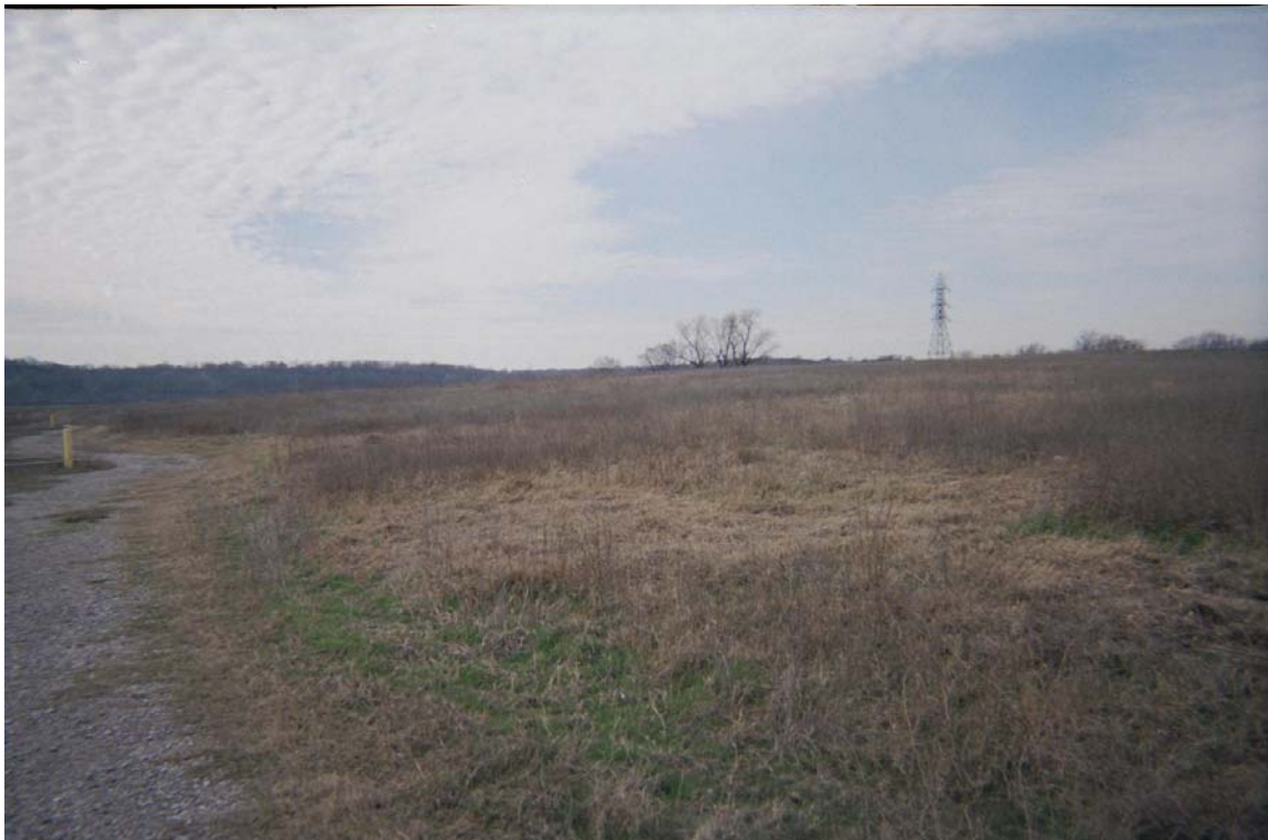
Photograph No. 2 Orientation: Southwest Description: Landfill cap with perimeter road
