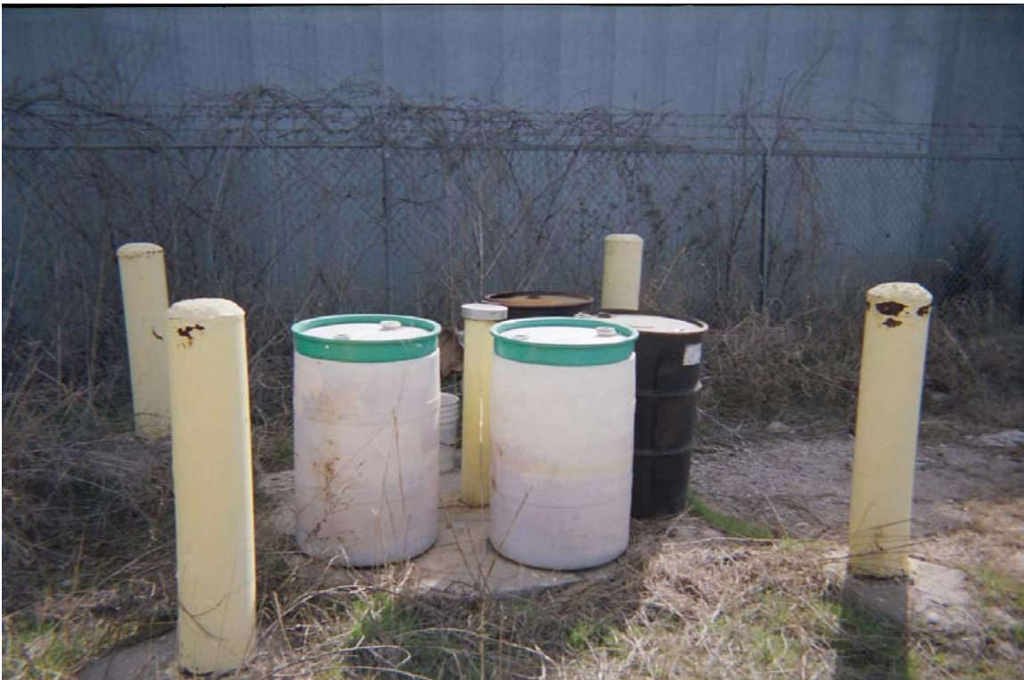
Photograph No. 4 Orientation: East Description: Monitor well MW104, with storage drums for collection of light nonaqueous phase liquid extracted from well
