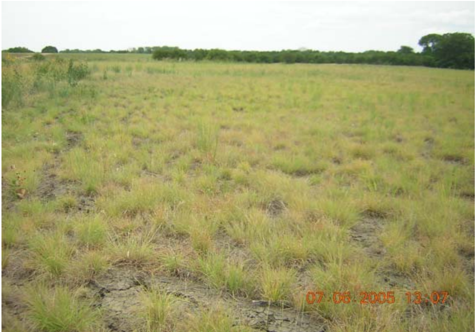
Photo 25: OU3, Site 4 – view of soil cover at site, facing west. There are numerous desiccation cracks in the surface of the soil cover and the vegetation is sparse.
