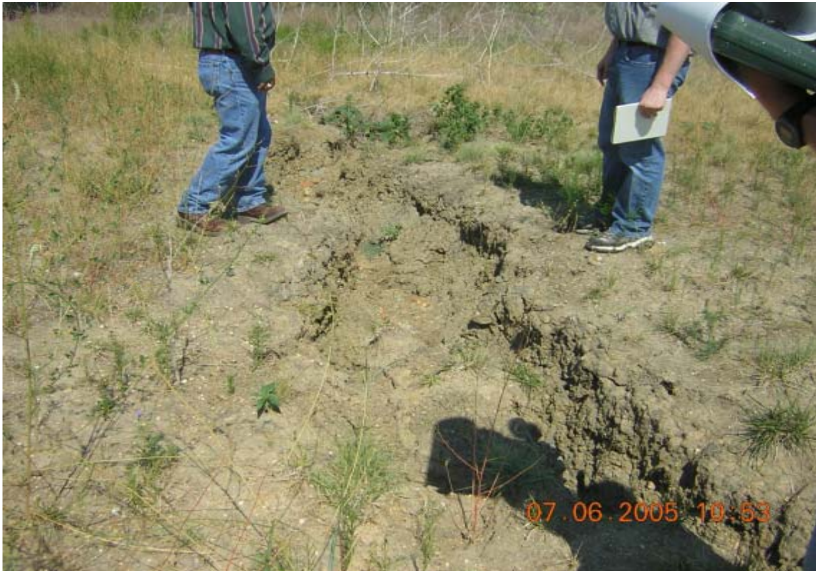
Photo 9: OU5, Subarea 2 – View of large erosion channel west of cover over former landfill.
