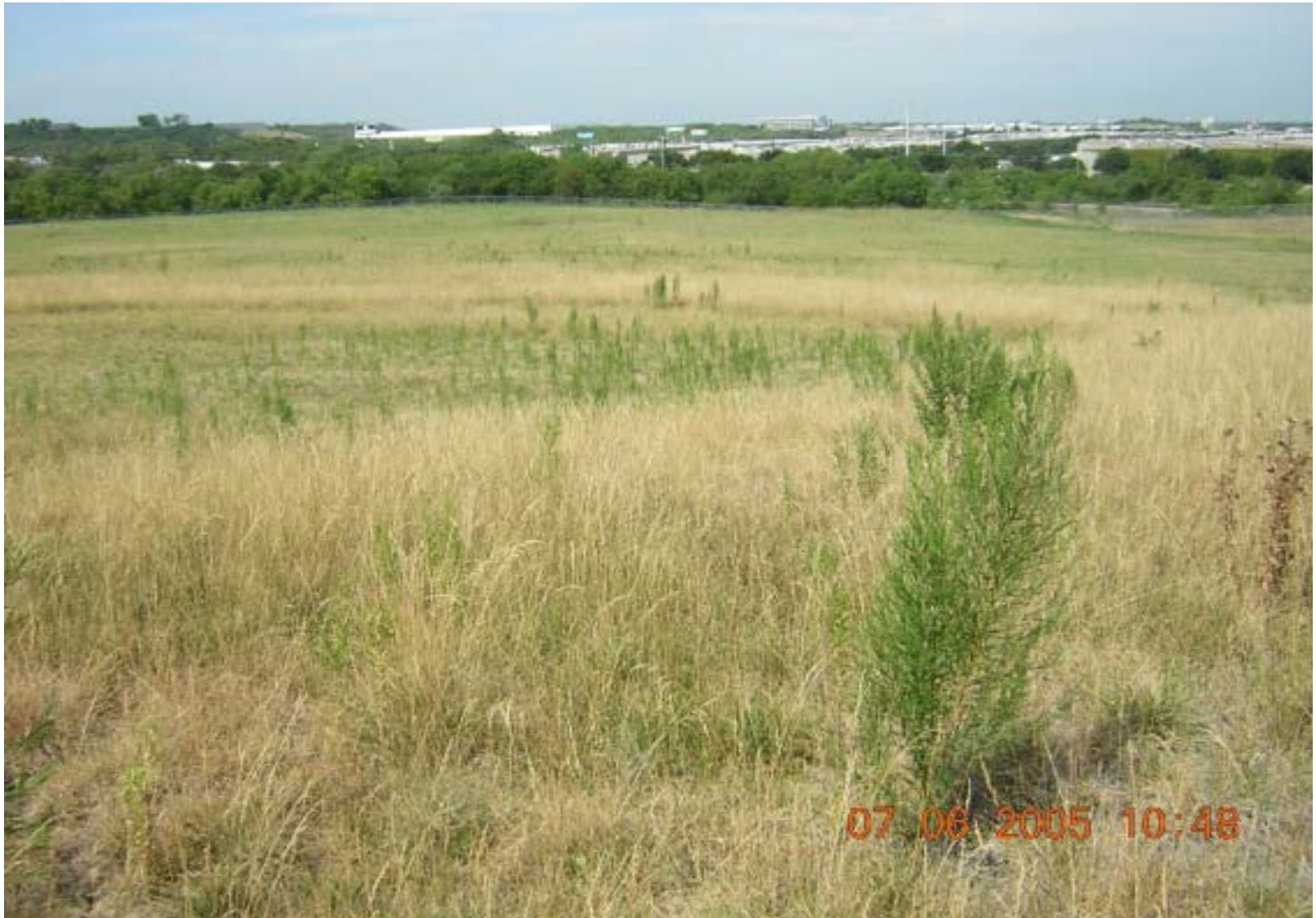
Photo 6: OU5 – Subarea 2, view of cover on former landfill, facing northwest.
