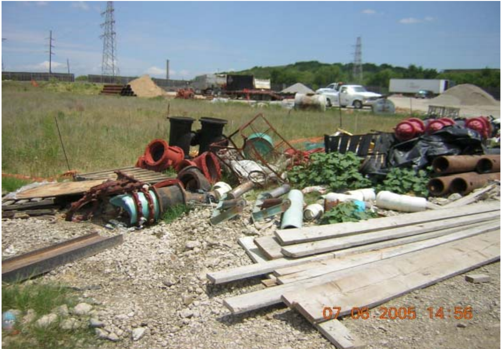
Photo 35: OU4 – View of site. Construction company has stored equipment and materials on the site.
