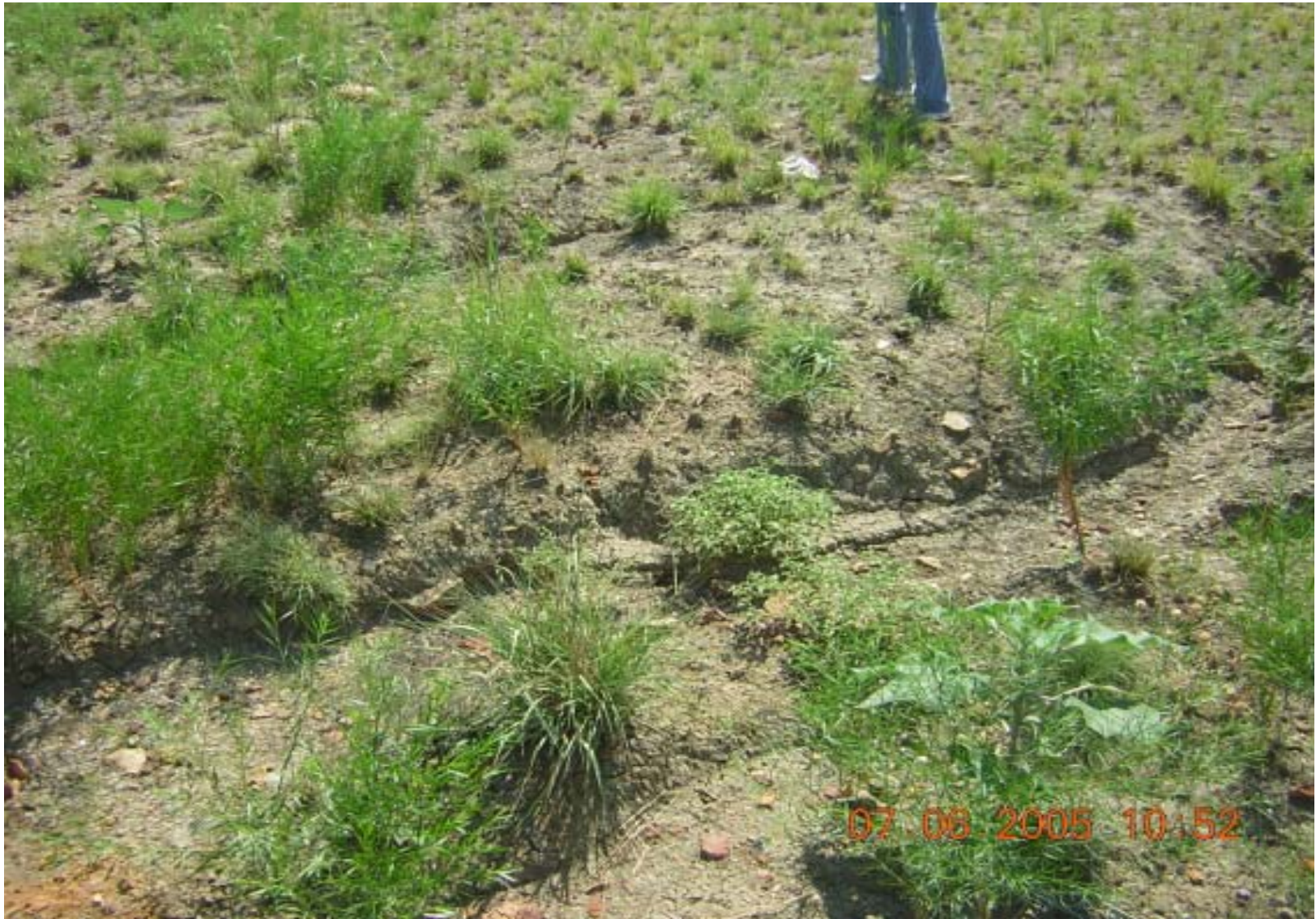
Photo 8: OU5 Subarea 2 – view of erosion channel near former landfill cover.
