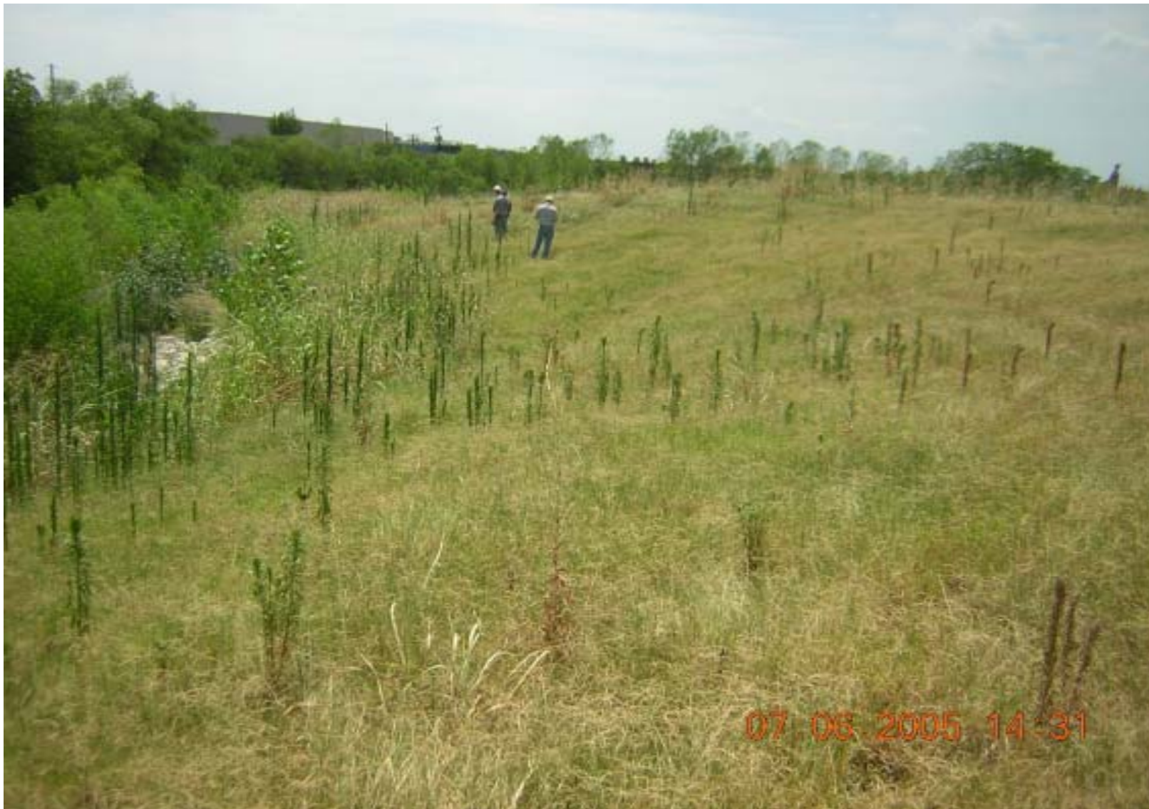
Photo 28: OU5, Subarea 1 – View of the cover over the buried slag area, facing west. The drainage channel is present on the left.
