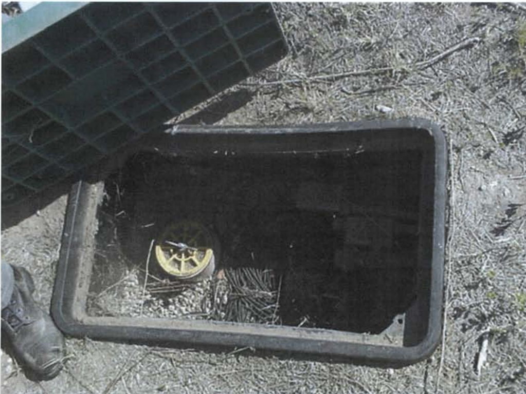
Photograph No. 8 Description: Monitoring well TW-6C
