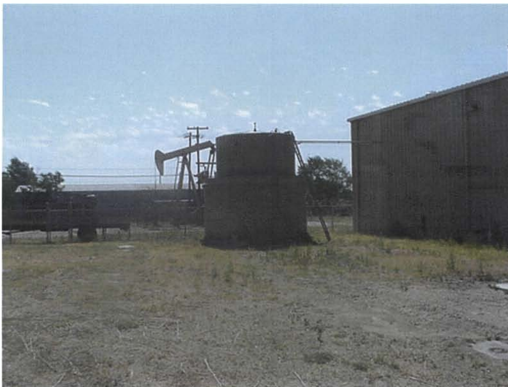
Photograph No. 3 Description: Eastern portion of the site
