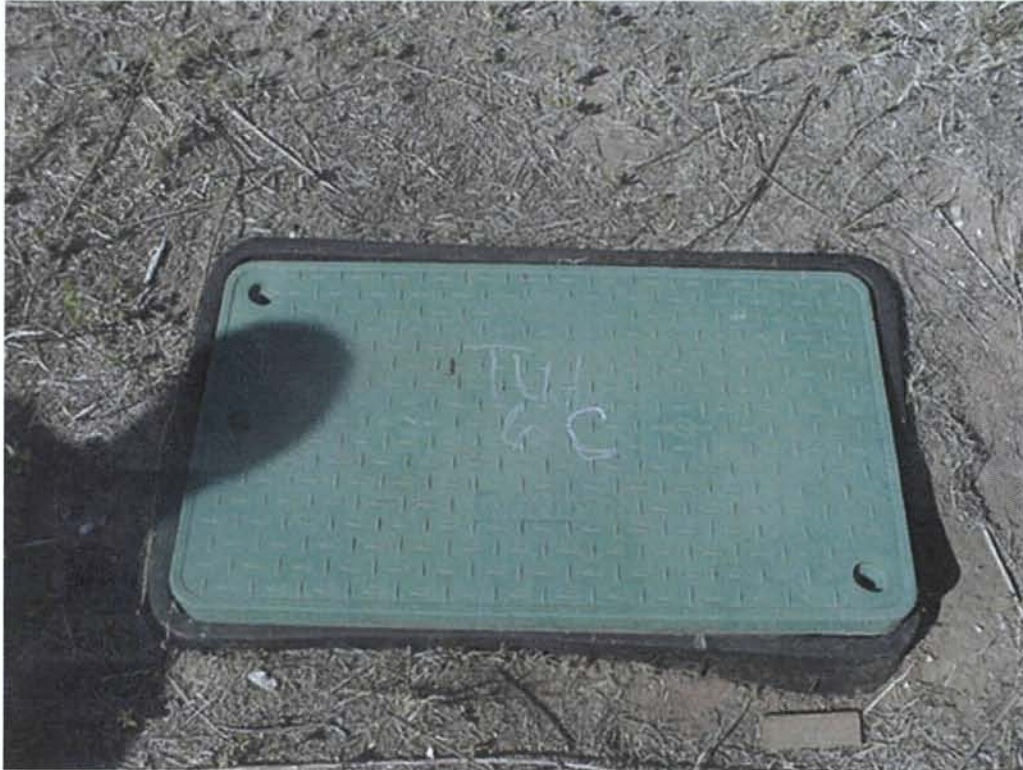
Photograph No. 7 Description: Monitoring well TW-6C
