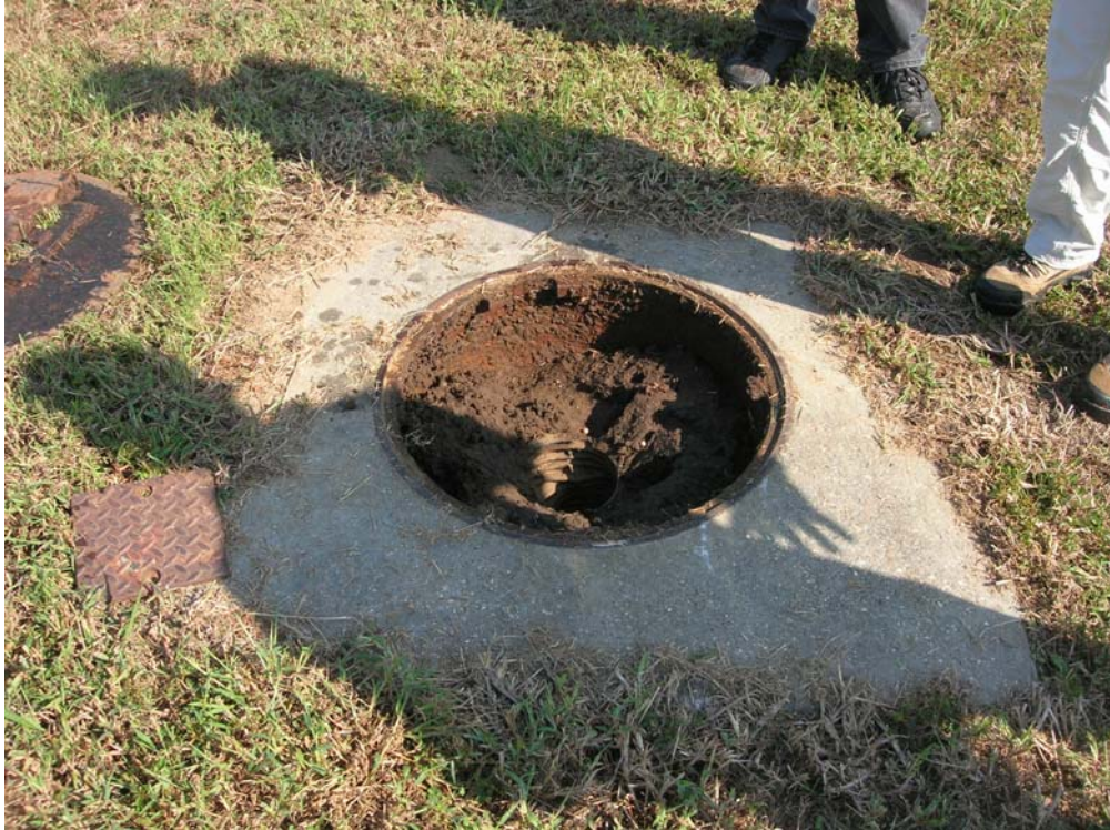
Photograph No. 19 Orientation: North Description: Recovery trench #9 cleanout
