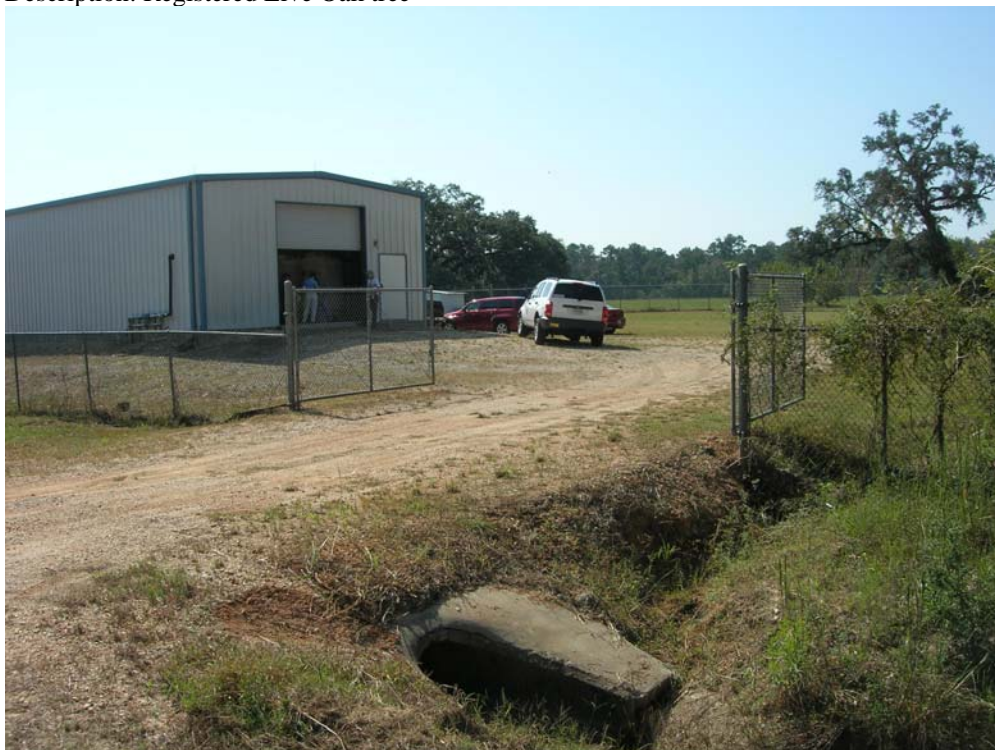
Photograph No. 2 Orientation: Southeast Description: Wastewater Treatment Plant Building (registered live oak in center rear of photo)
