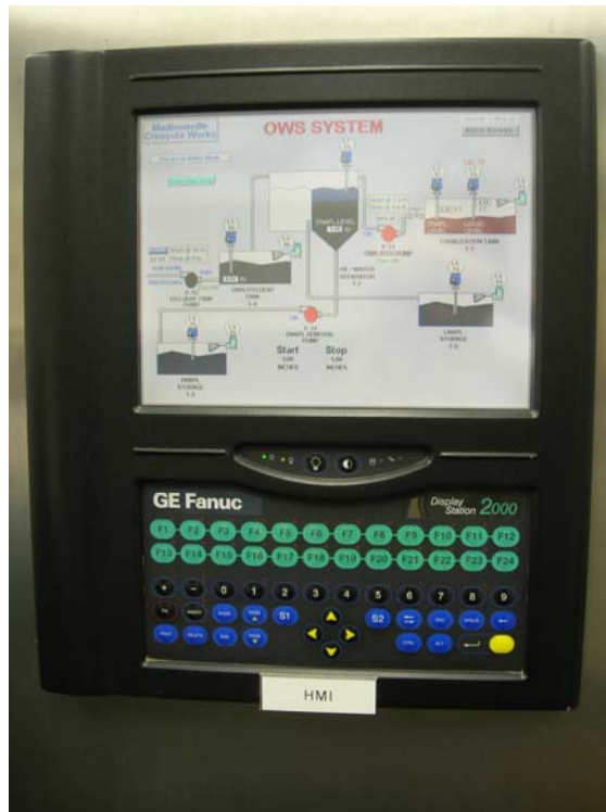
Photograph No. 10 Site: Madisonville Creosote Works Orientation: North (Wastewater treatment plant interior) Date: 30 September 2008 Description: Wastewater treatment plant programmable logic controllers (PLC) screen
