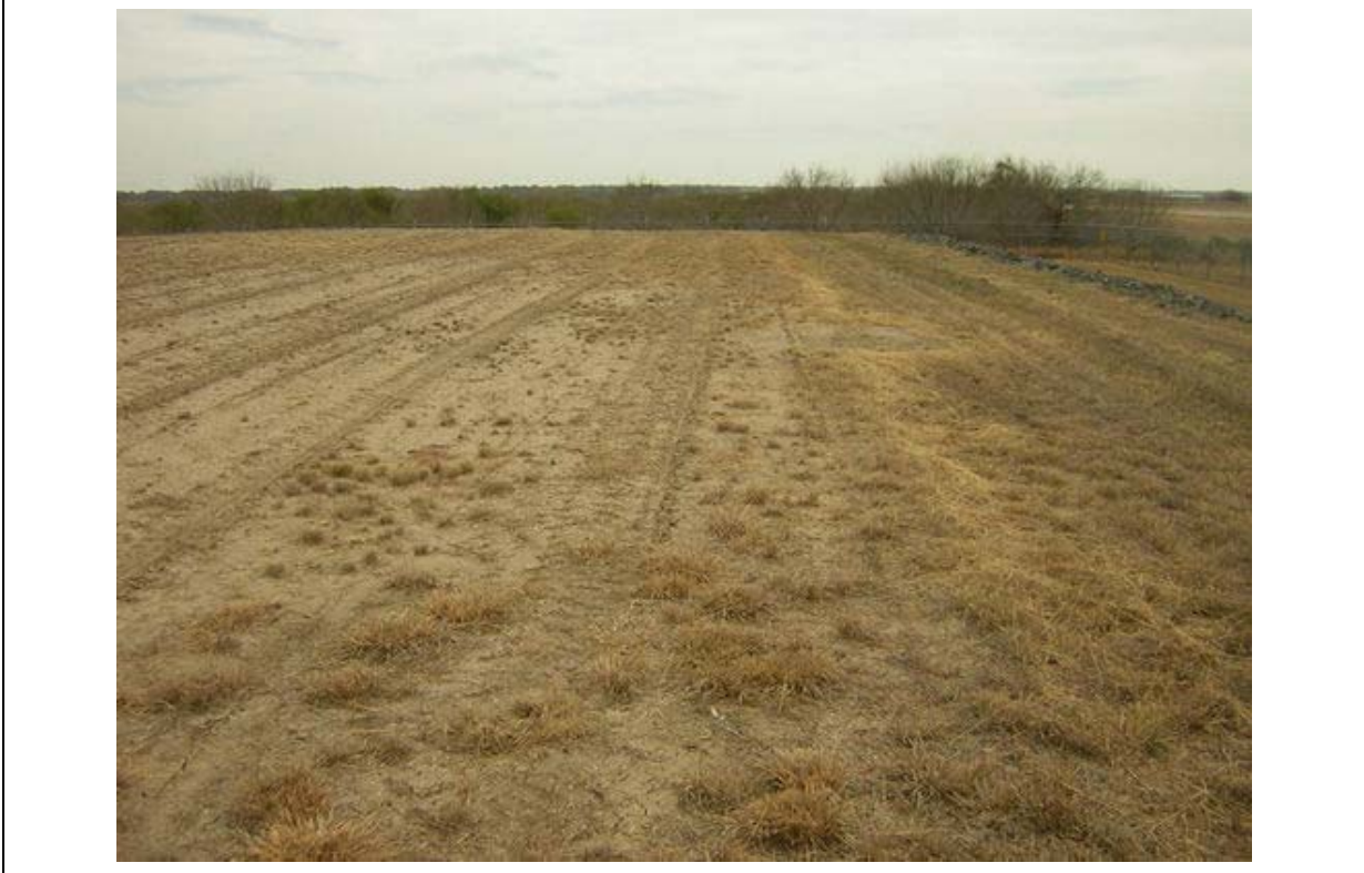
Photo 6: View of landfill cover. Note stressed vegetation due to dry conditions.
