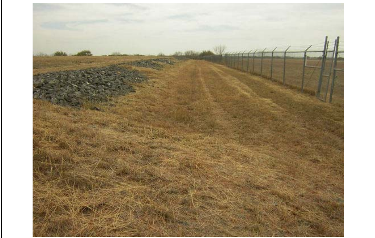
Photo 4: View along southwest side of landfill, inside fence.
