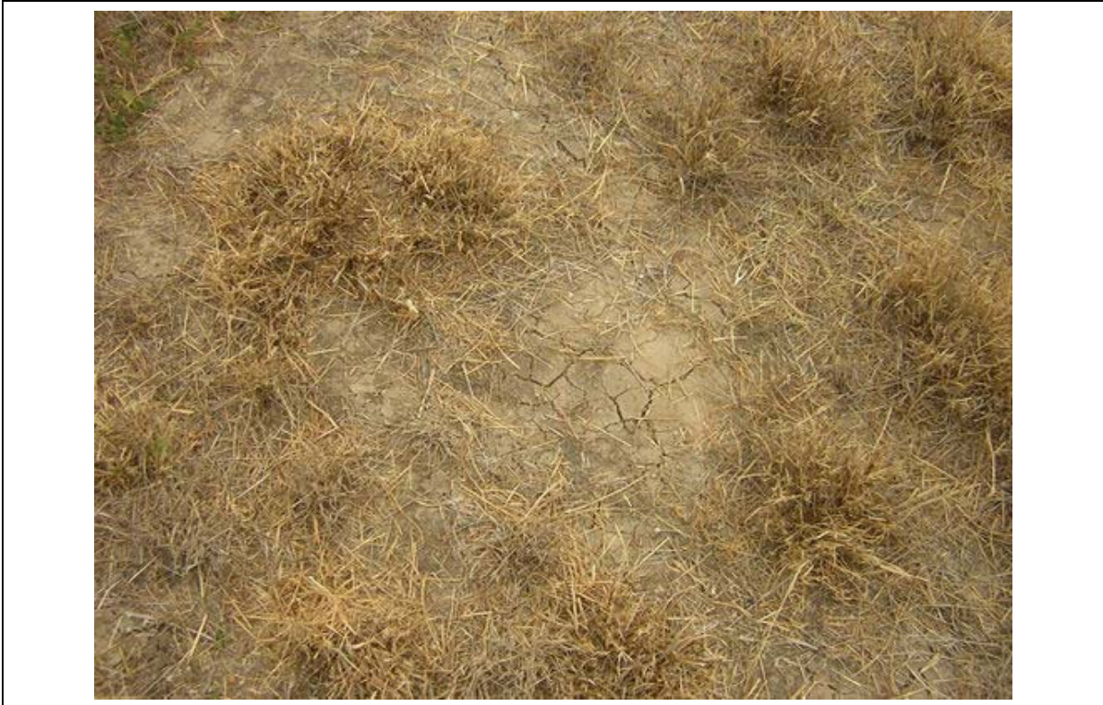
Photo 7: Minor cracks in landfill cover due to dry conditions.
