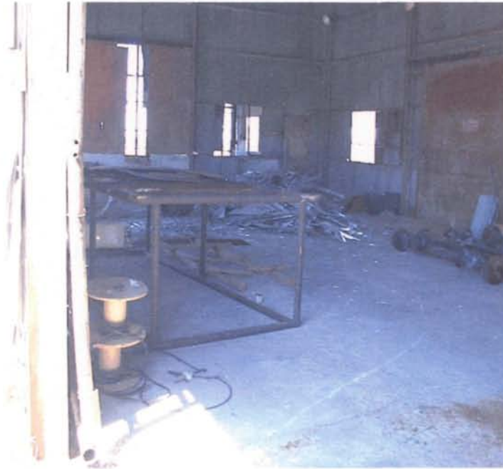
Photo 7 - Middle building being used for welding operations.
