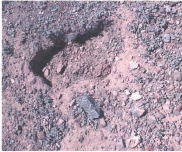
PHOTO 3 - PHOTO OF LOCATION WHERE ANIMAL BURROWED ON SURFACE OF REPOSITORY CELL
