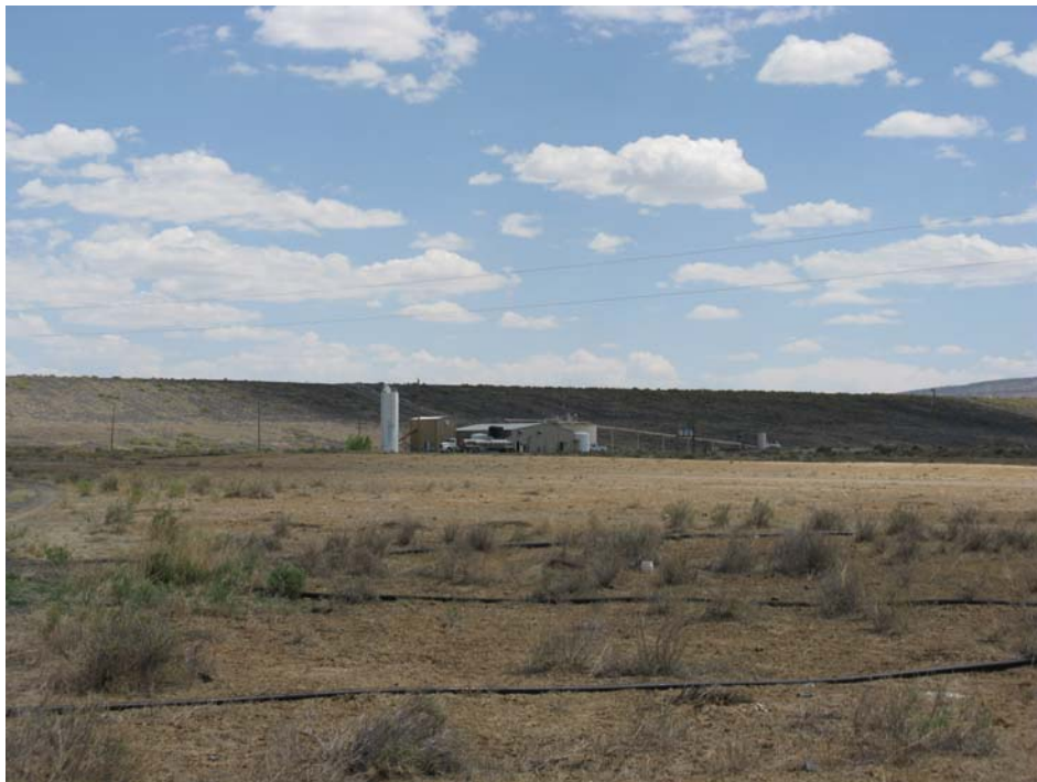
Large Tailings Pile in distance behind RO plant with aboveground piping in the foreground (looking northeast)
