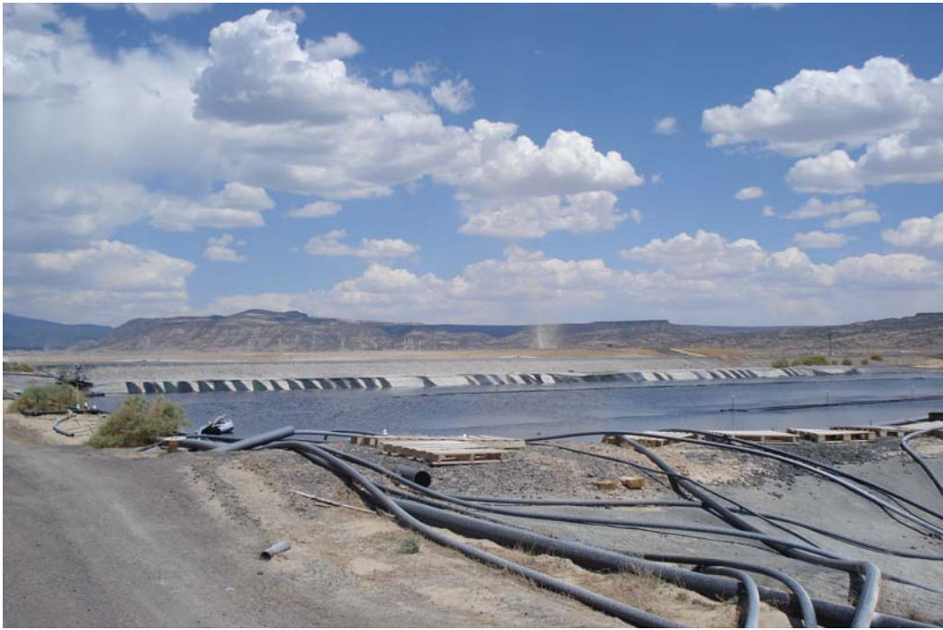
Collection Pond #2 (looking east)
