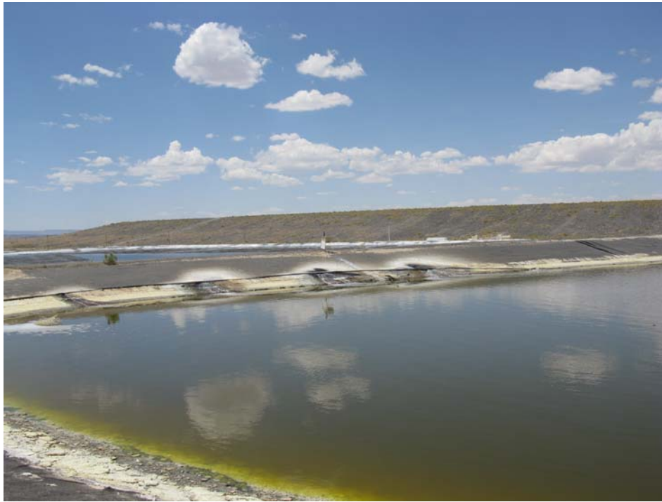
Evaporation Pond #1 showing pumping of water to cover liner with brine (yellow-white color) (looking northwest)
