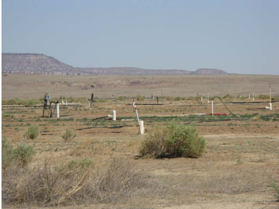
Extraction and injection (red striped) wells (looking northwest)
