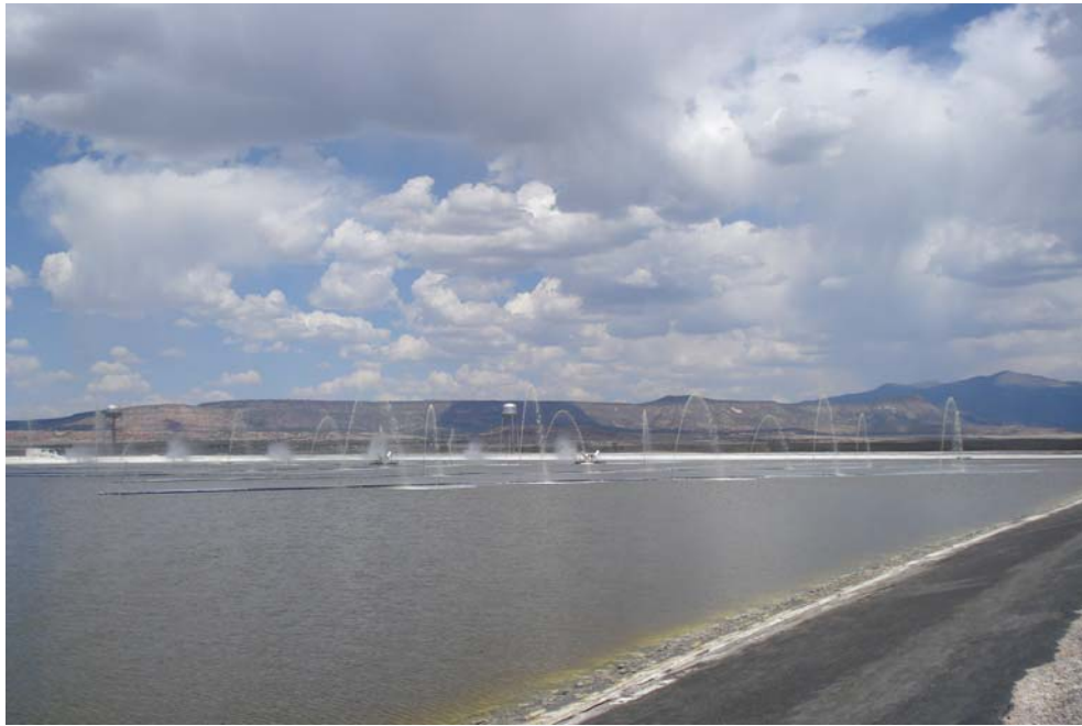
Evaporation Pond #1 with sprayers (looking northeast)
