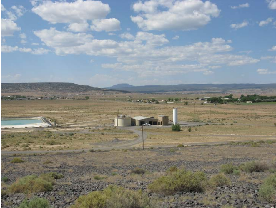
RO Plant from Large Tailings Pile (looking southwest) (Clarifier to the left and lime slaker unit to the right)
