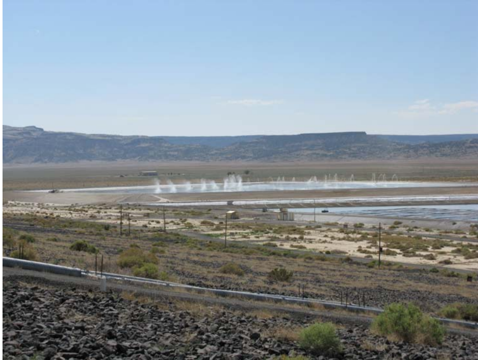
Evaporation Pond # 1 with sprayers on from Large Tailings Pile (looking southeast)
