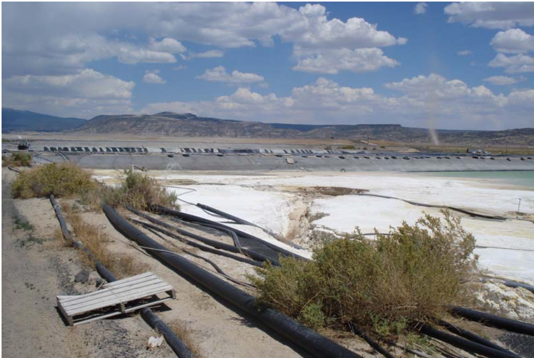
Collection Pond #1 (looking east)
