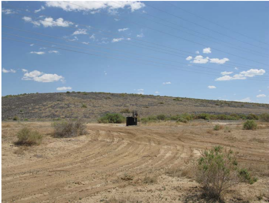
Toe drain collection sump with tailings pile behind (looking northeast)
