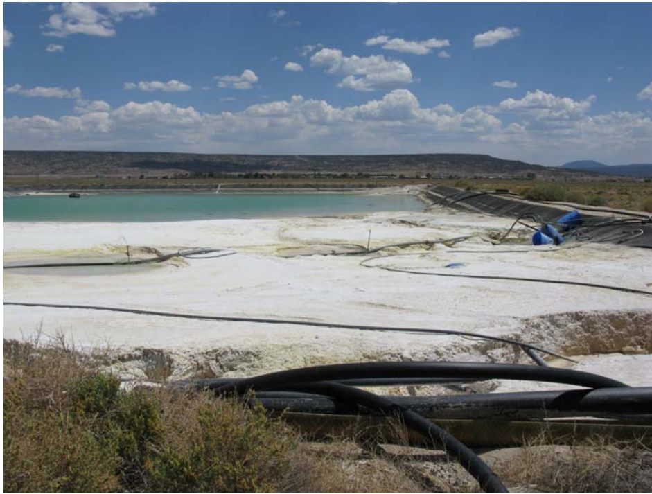
Collection Pond #1 showing sludge and various discharge lines (looking south)
