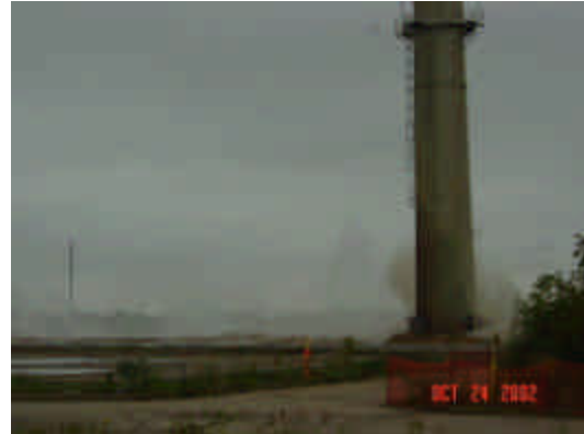
Figure 1: Base of smokestack being imploded.
